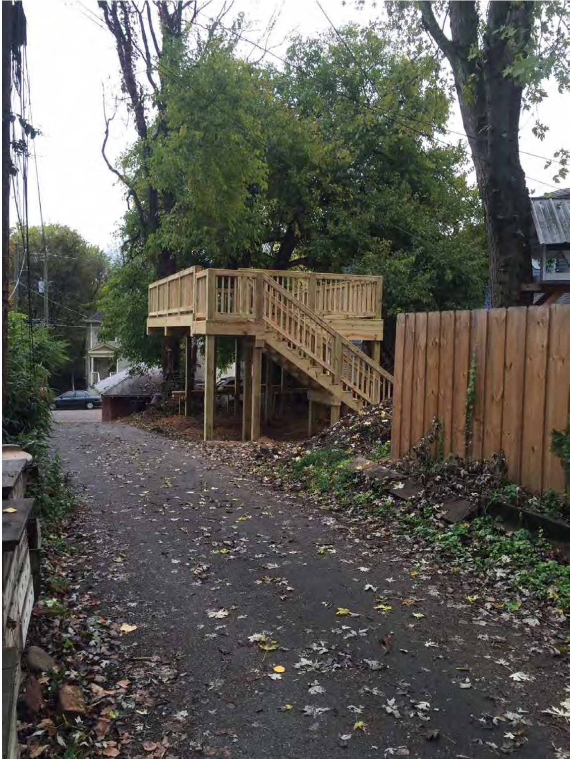
706 Luttrell – From the alley - existing view looking south towards 3rd St.
