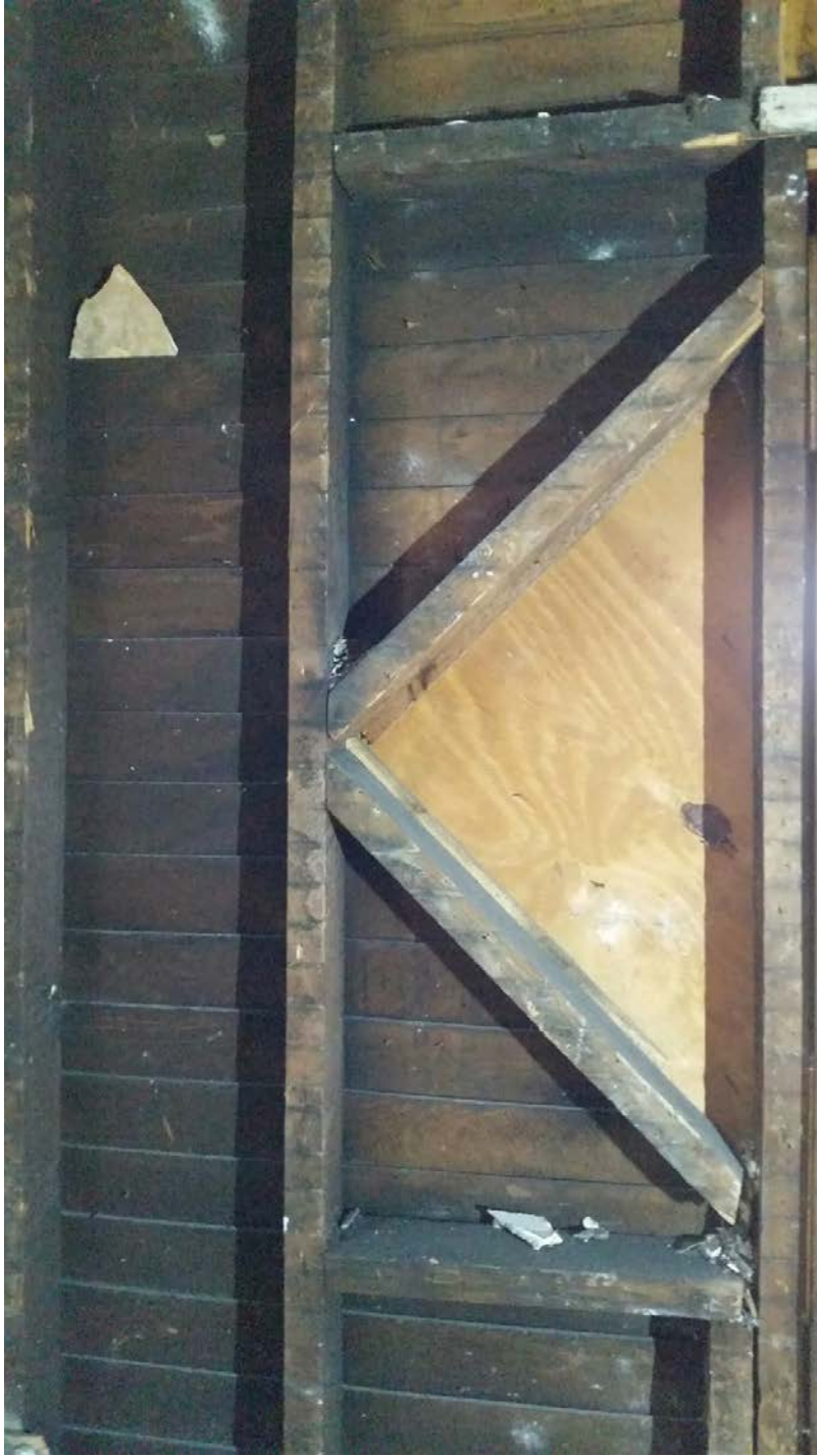
129 Ok – Possible diamond-shaped window framing at front porch
