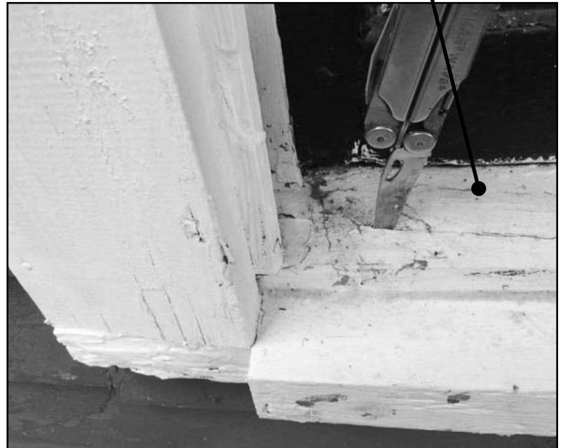
Original Window: First level_west side toward front
