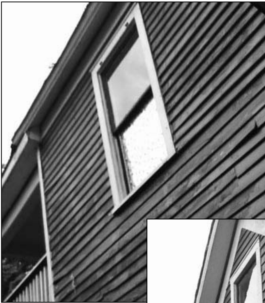
East side view: Original window toward front, second level
