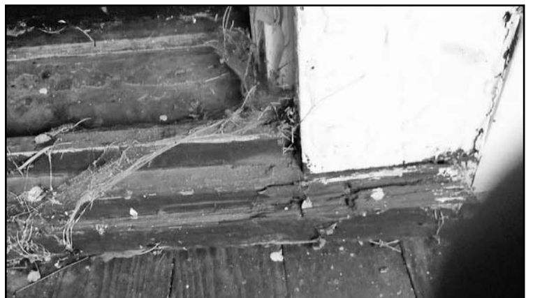
Below: Front door double threshold
