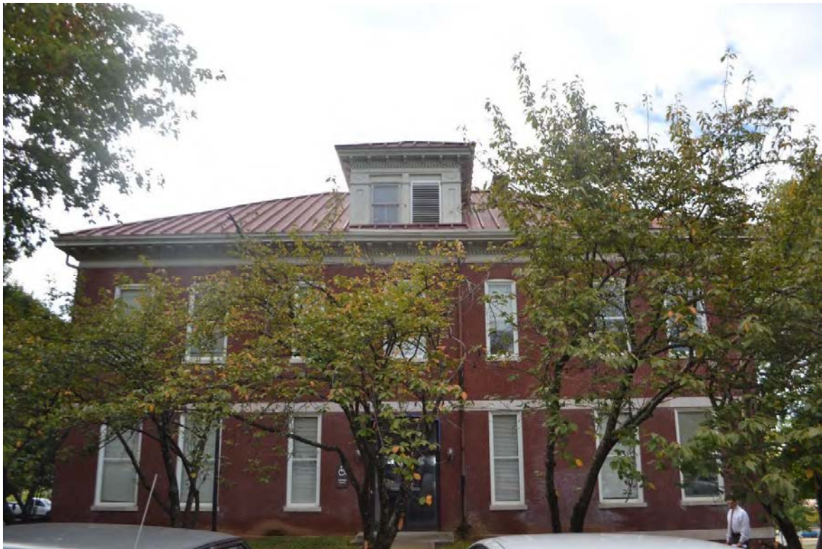
Duncan Law School – North side showing main entry
