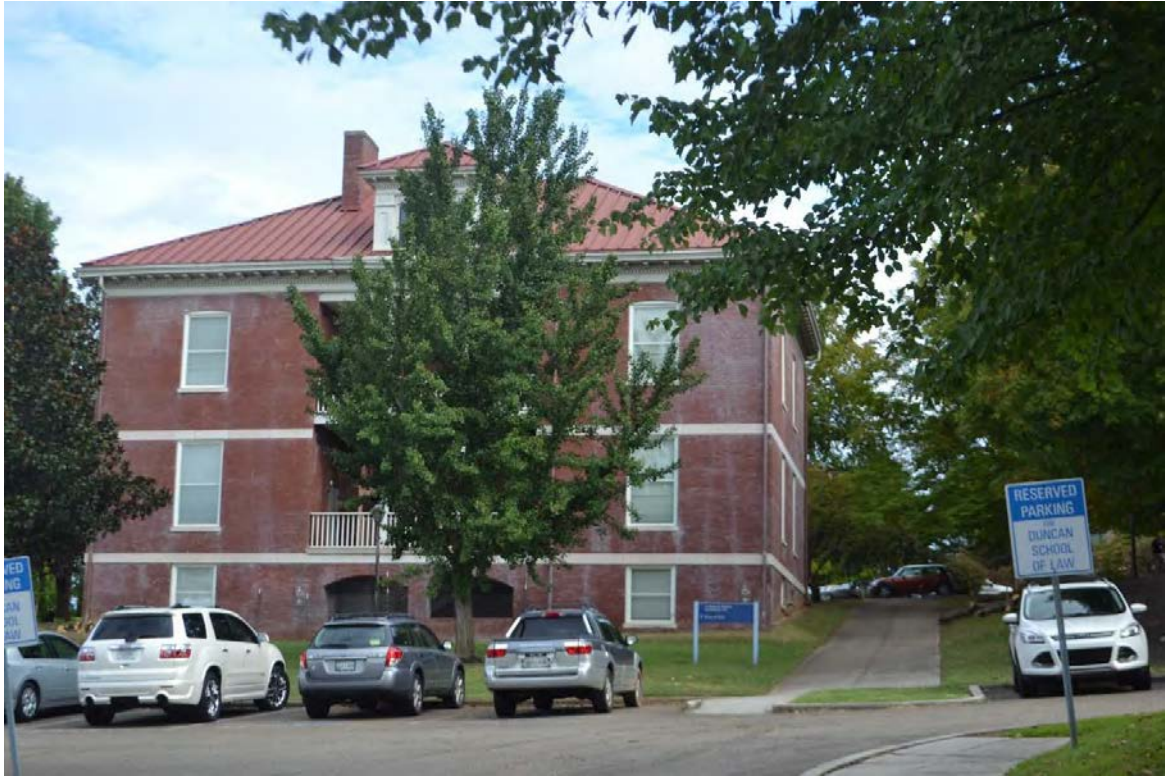
Duncan Law School – Parking lot and landscaping along south side and to the east
