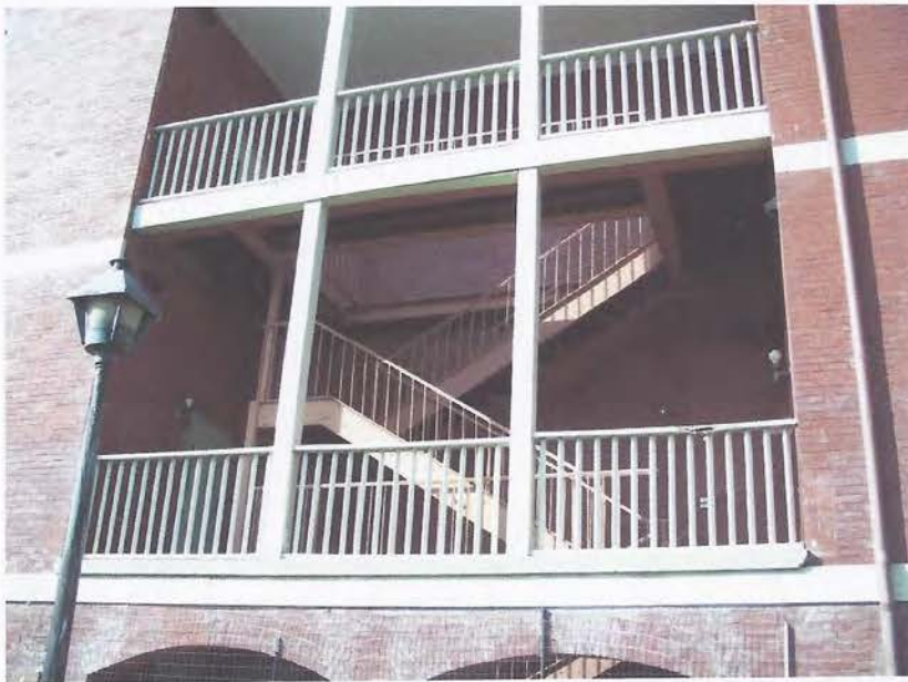
Non-historic steel stair to be removed
