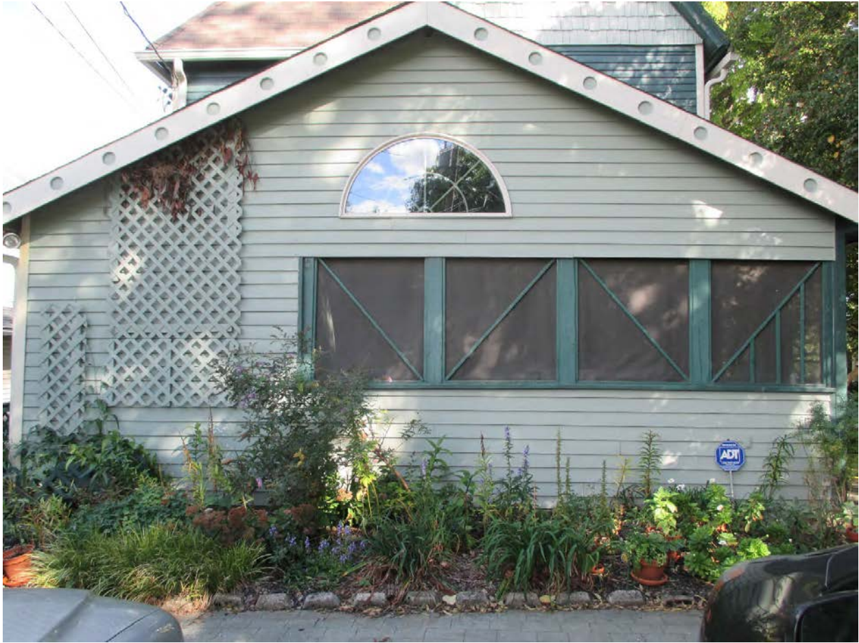
1007 Luttrell – Close-up of rear addition
