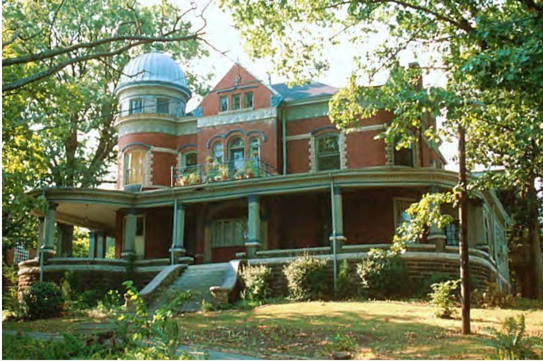
1633 Clinch Ave. – Before burn
