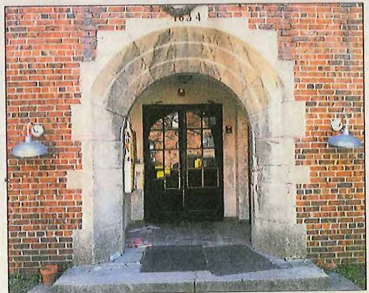
An apartment building at 1634 Laurel Ave. will undergo a complete renovation.
