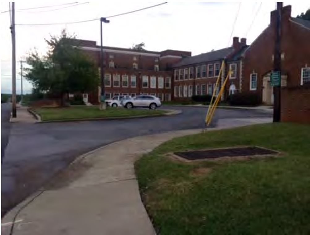
Brownlow Lofts – As seen from sidewalk approaching from the west
