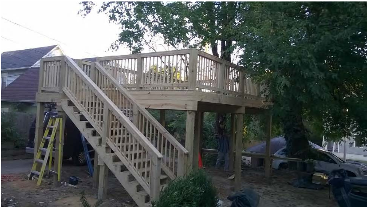
706 Luttrell – From house looking southeast across alley
