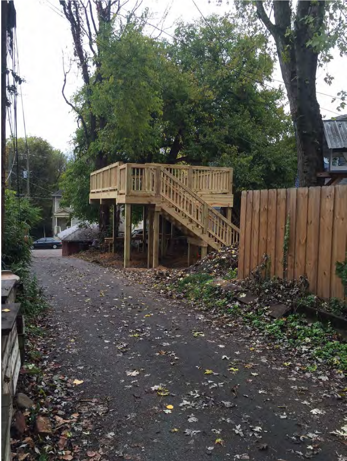
706 Luttrell – From the alley looking south towards 3 rd Street
