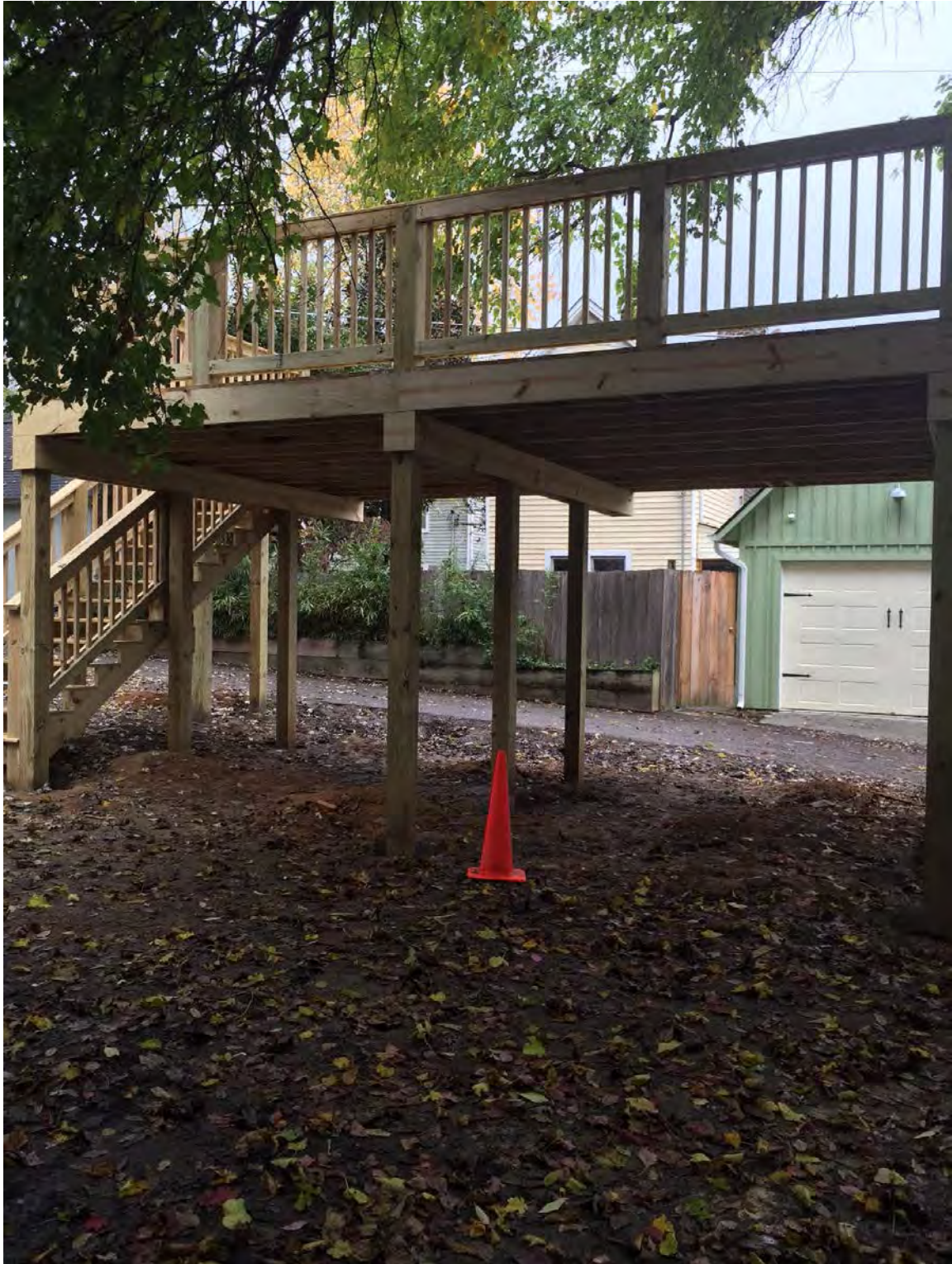
706 Luttrell – From house looking towards deck and across alley
