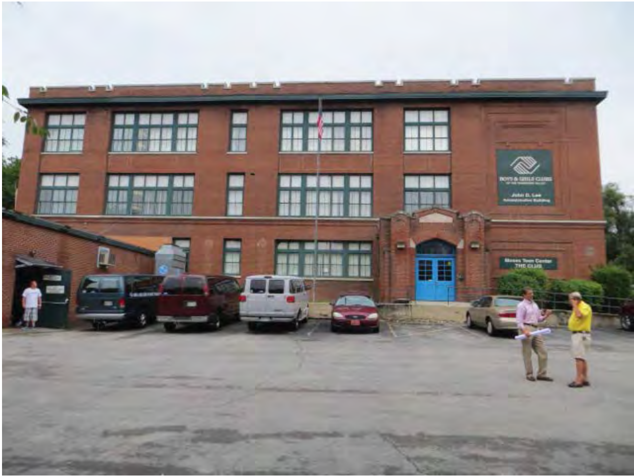
Emerald Academy - Overall south façade showing existing Boys and Girls Club metal signage proposed to be replaced.
