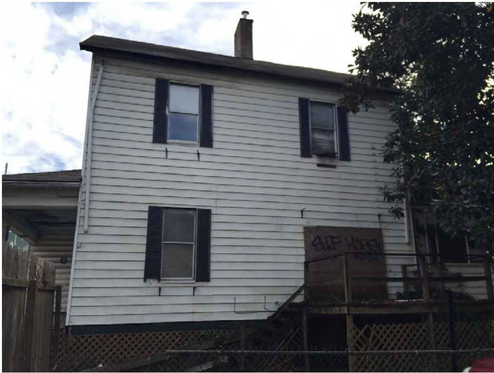
219 Twelfth – East side of house, 1
