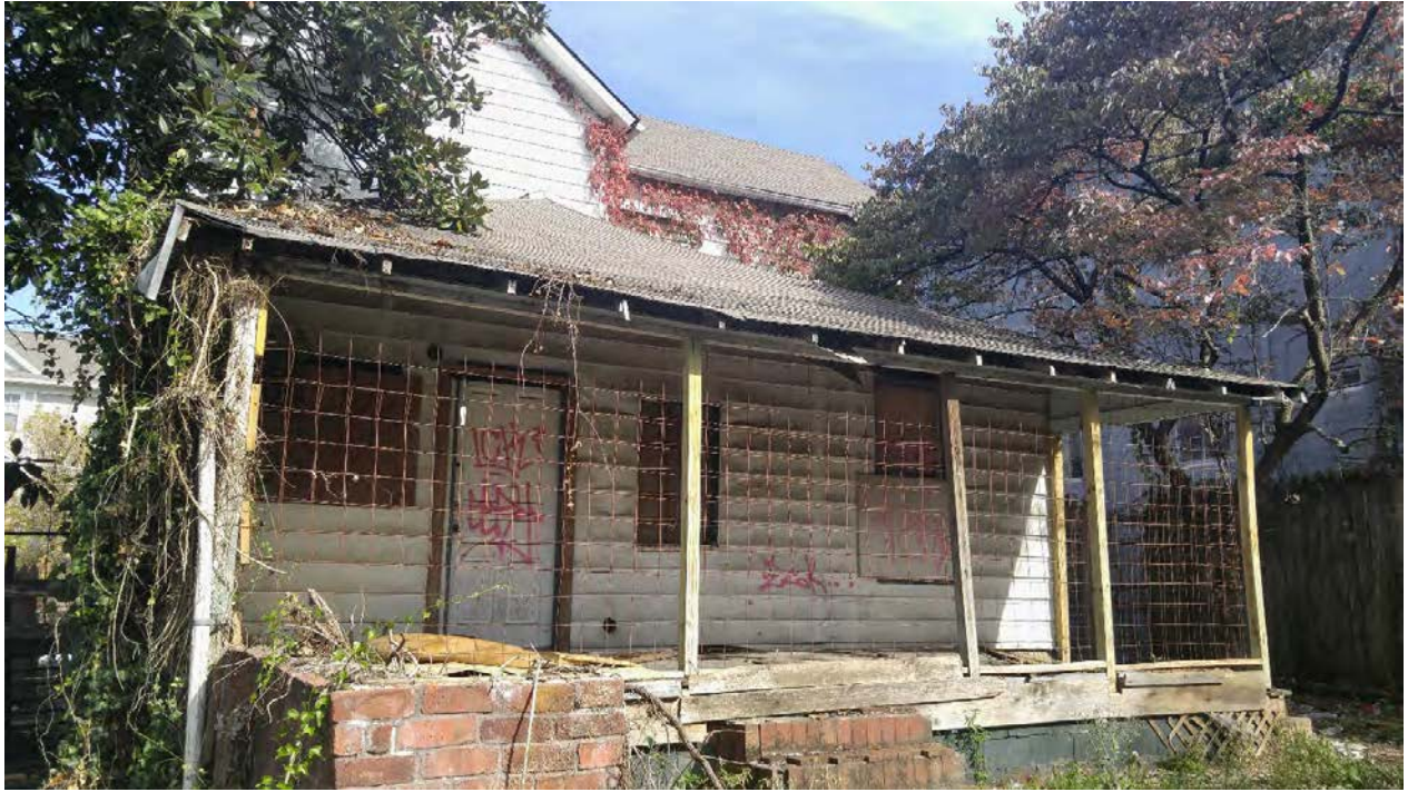
219 Twelfth – Rear (west) elevation showing non-original porch roof
