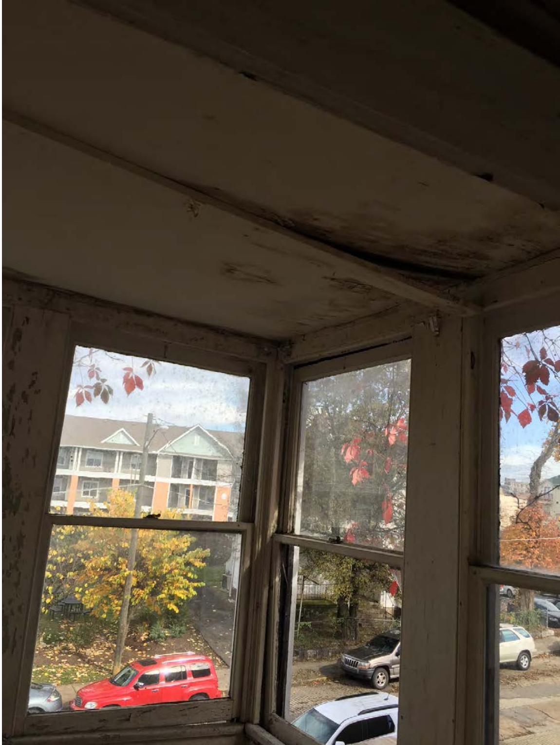
219 Twelfth – Interior view looking out front room
