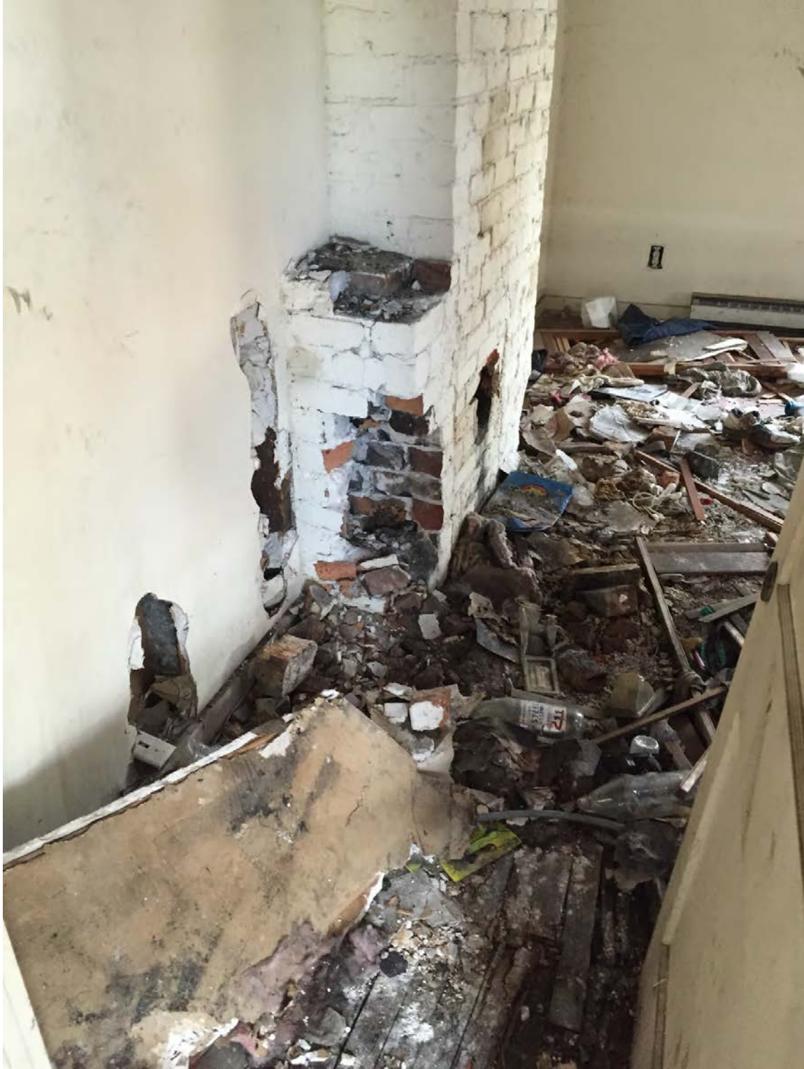
219 Twelfth – Interior view showing stove chimney
