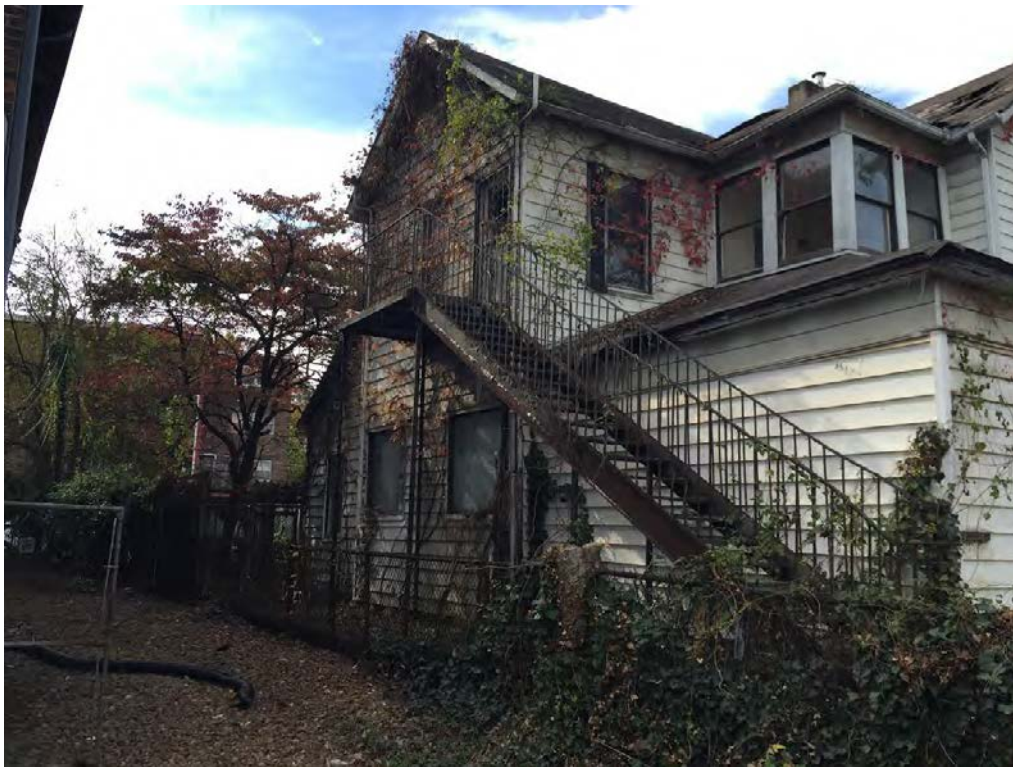
219 Twelfth – West side of house
