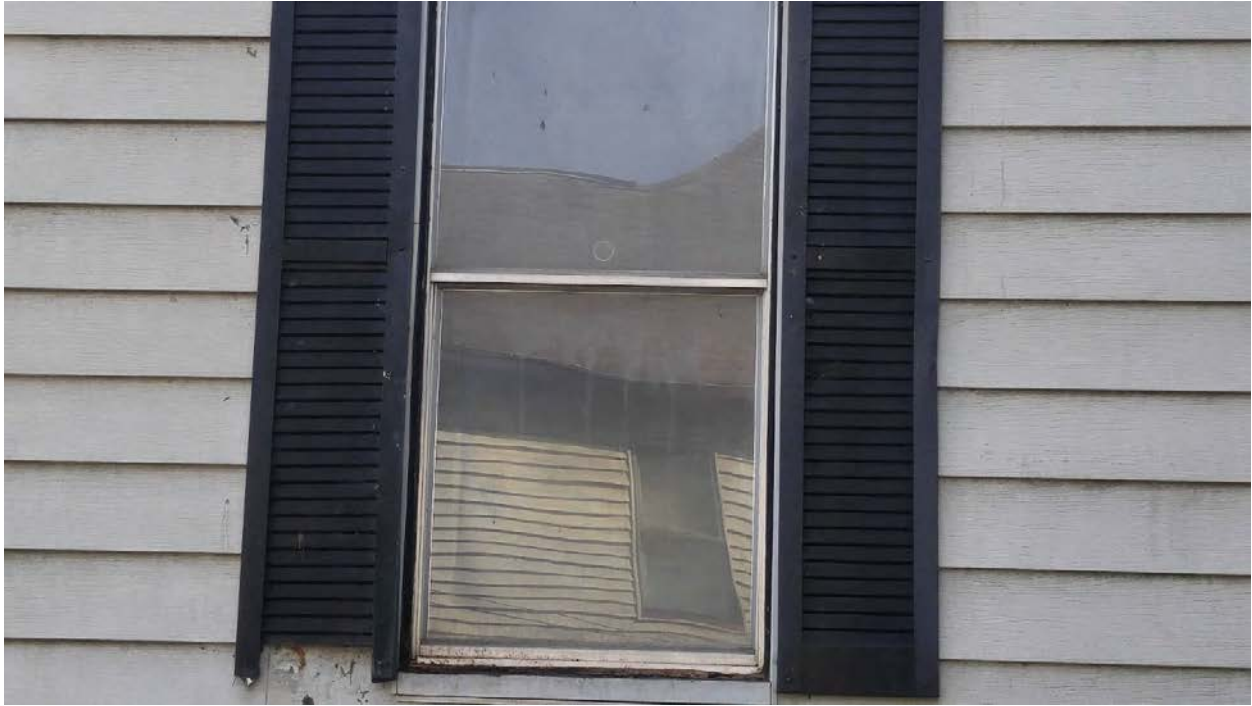
219 Twelfth – Non-original window on north side – 1 st level
