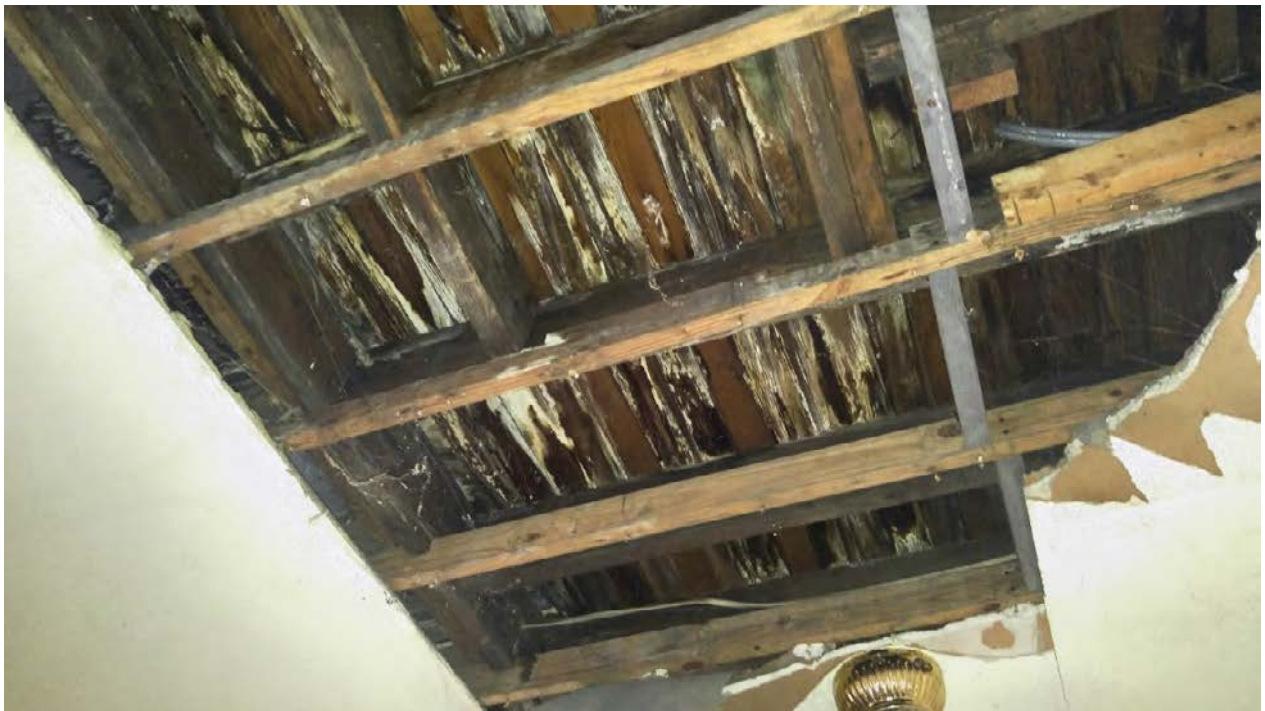
219 Twelfth – looking up at ceiling lathe
