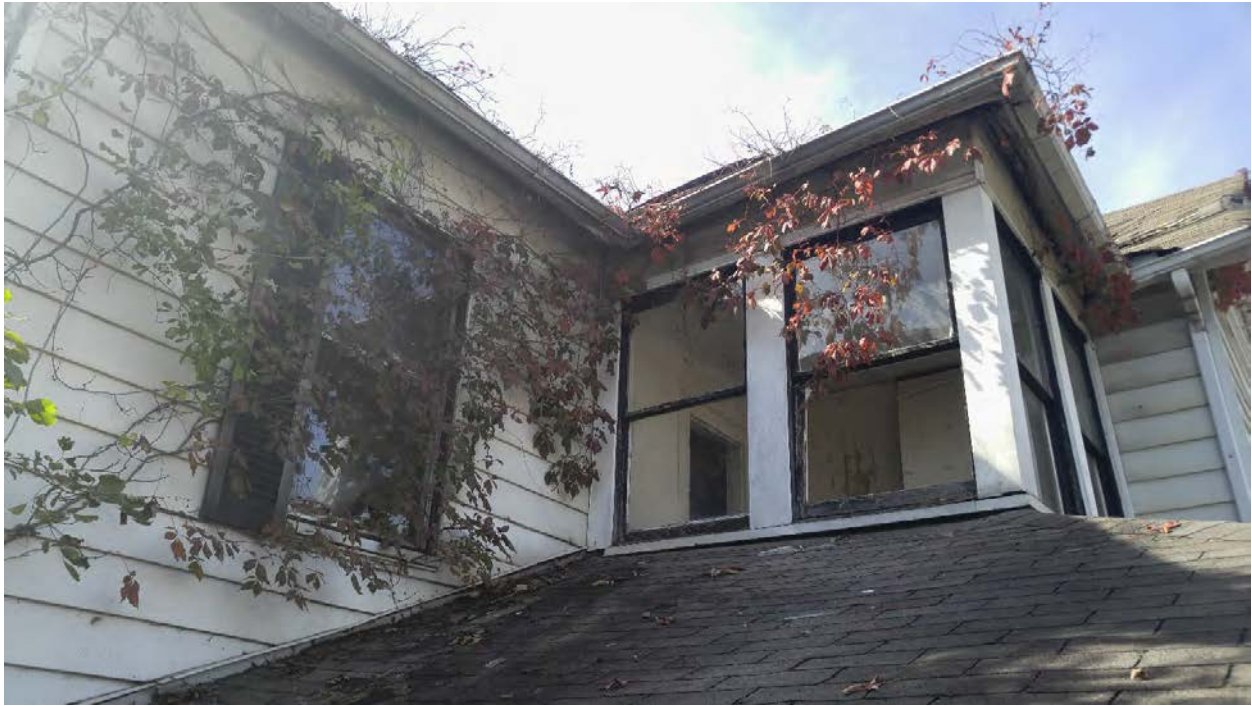
219 Twelfth – front add-on to 2 nd level over porch
