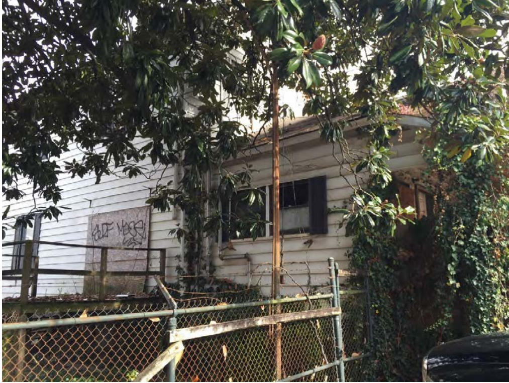
219 Twelfth – East side of house, 2
