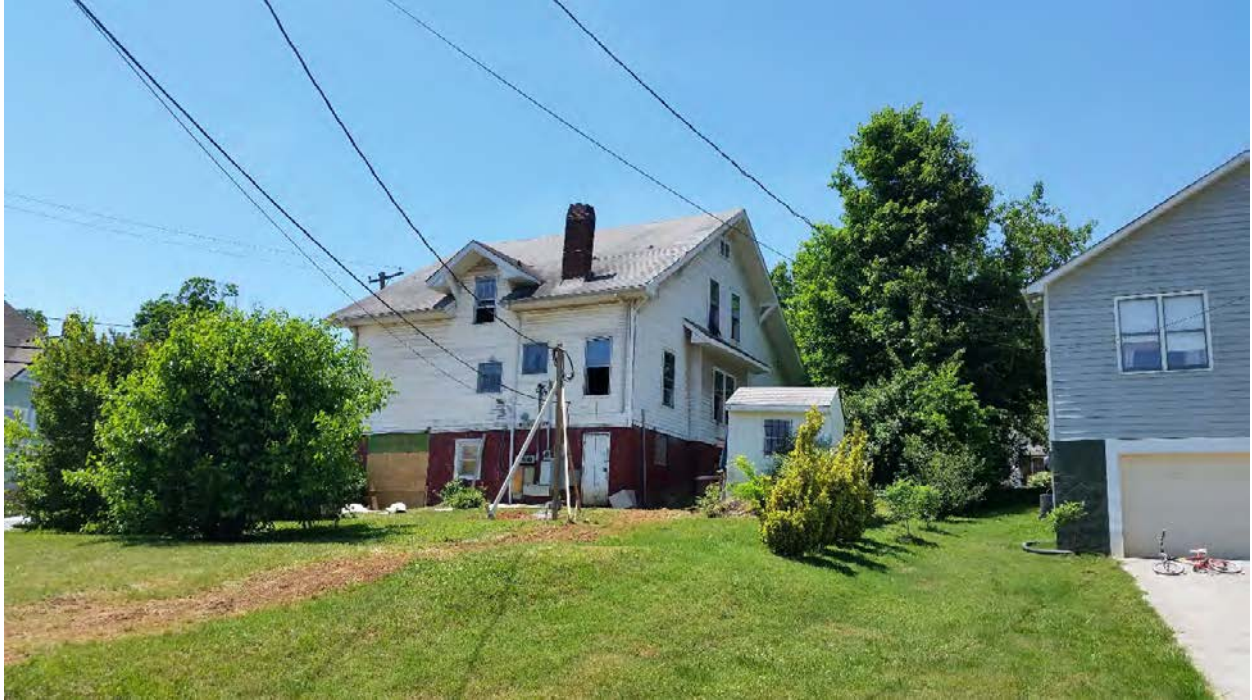
300 E. Oklahoma - Rear of house looking southwest from alley
