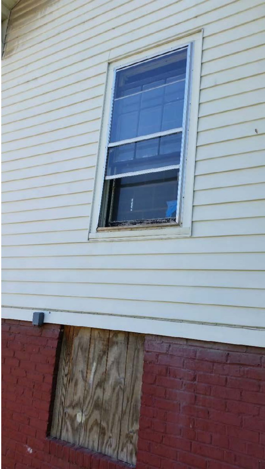
300 E. Oklahoma - Close-up of Window D on northeast
