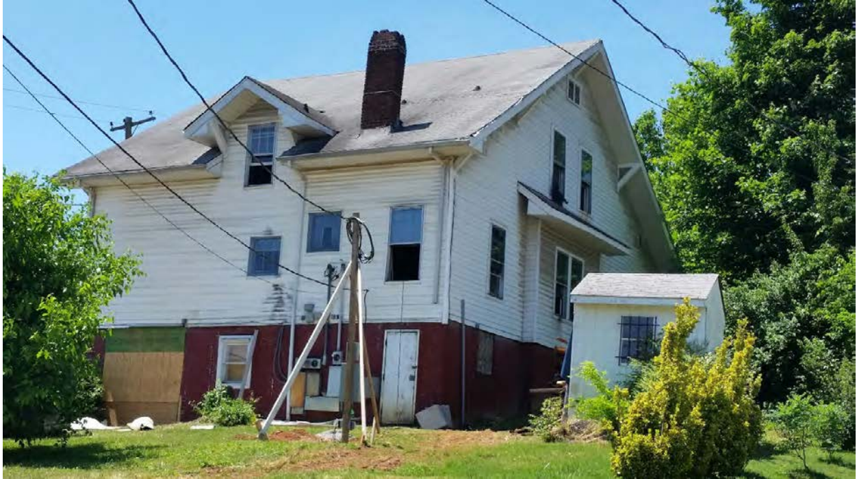
300 E. Oklahoma - Rear of house looking southwest from back yard
