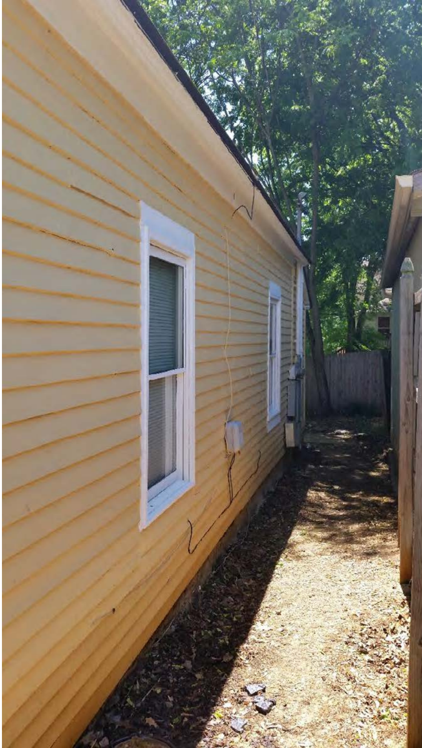
1209 Harvey - North side of house where windows are to remain
