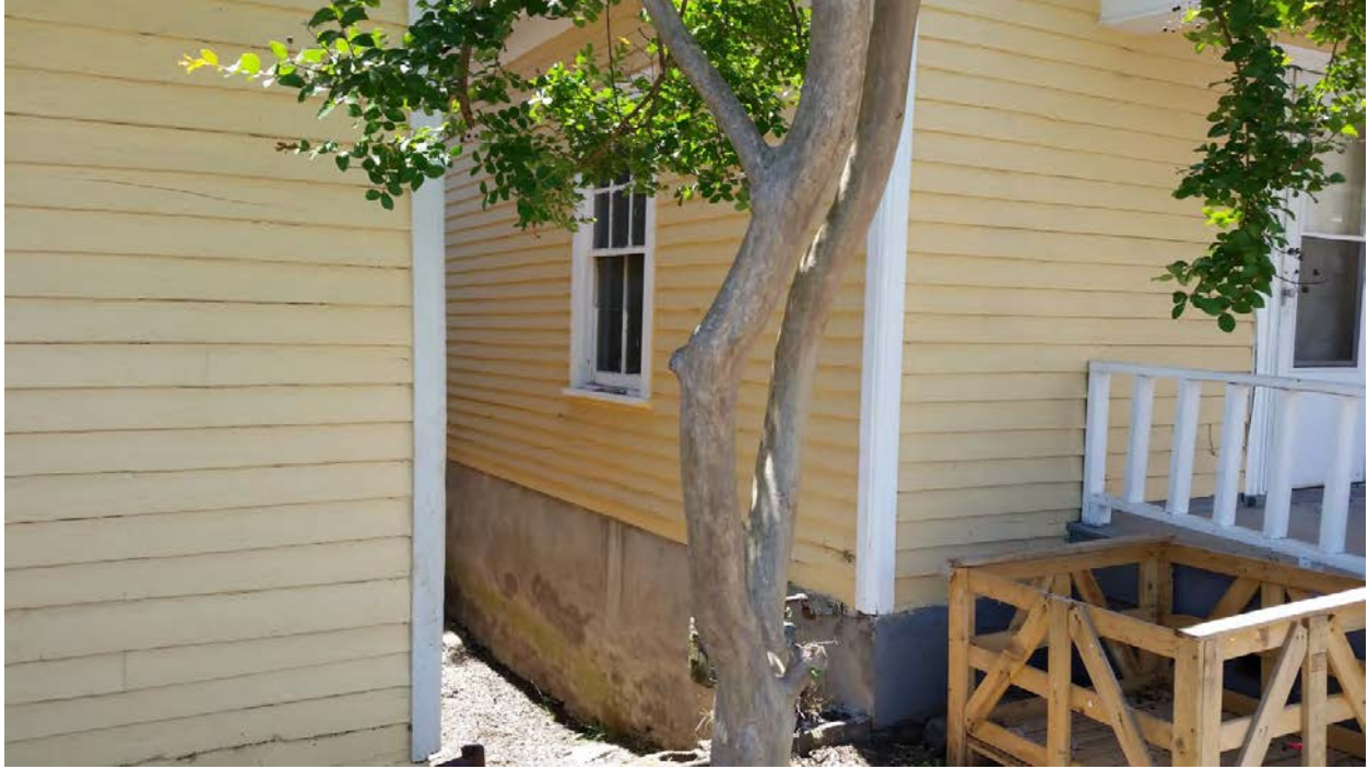
1209 Harvey - Window on south side as seen from street
