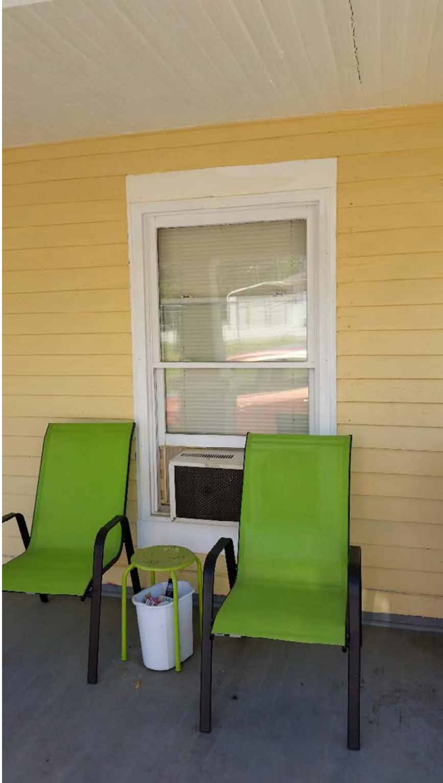
1209 Harvey - 1-over-1 window on front to remain
