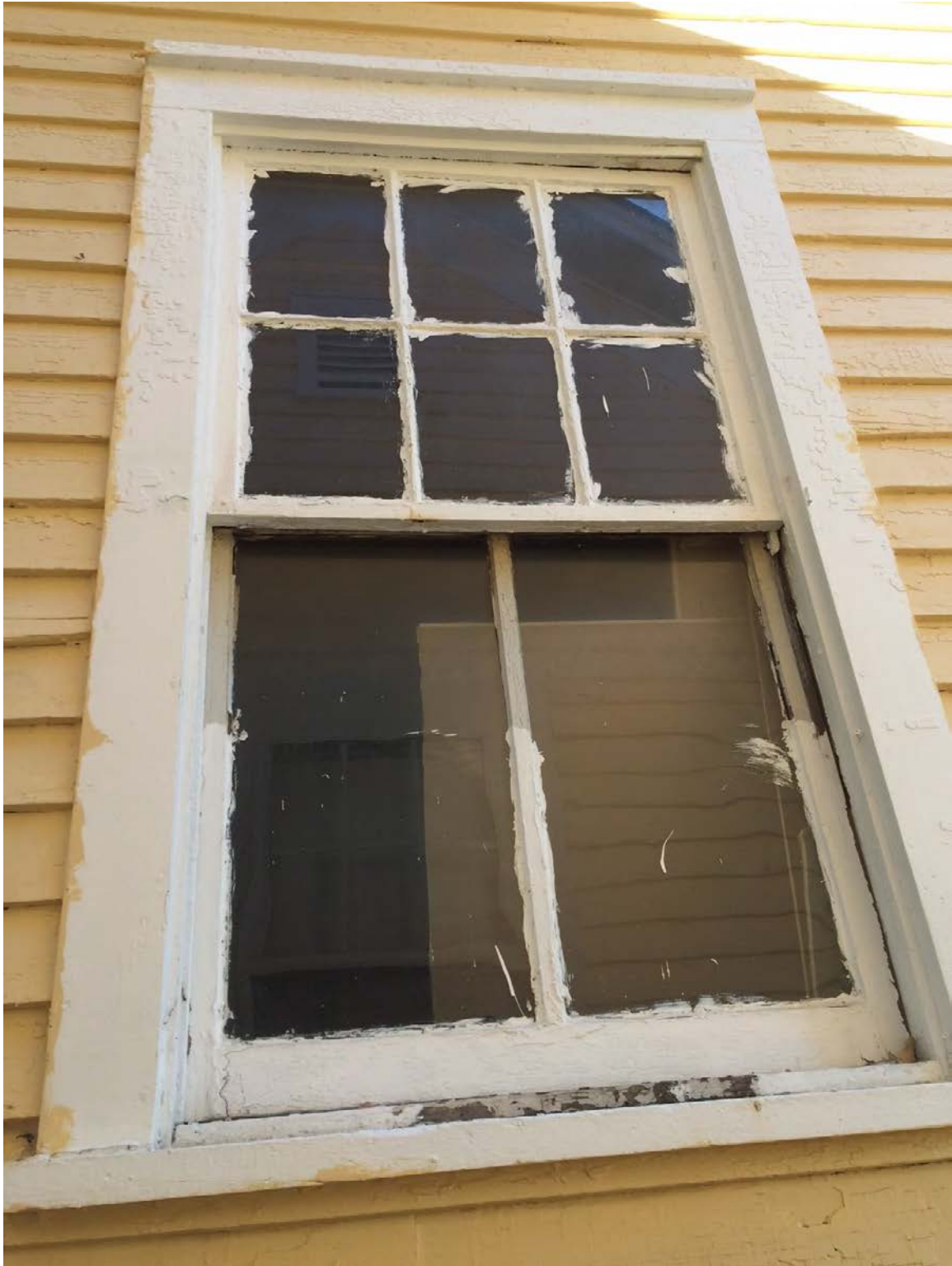
1209 Harvey - 6-over-1 window proposed to be replaced on south side of house
