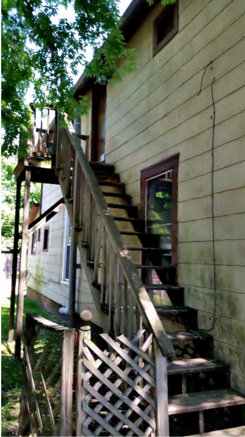
708 Morgan – Fire steps on NW side to be rebuilt
