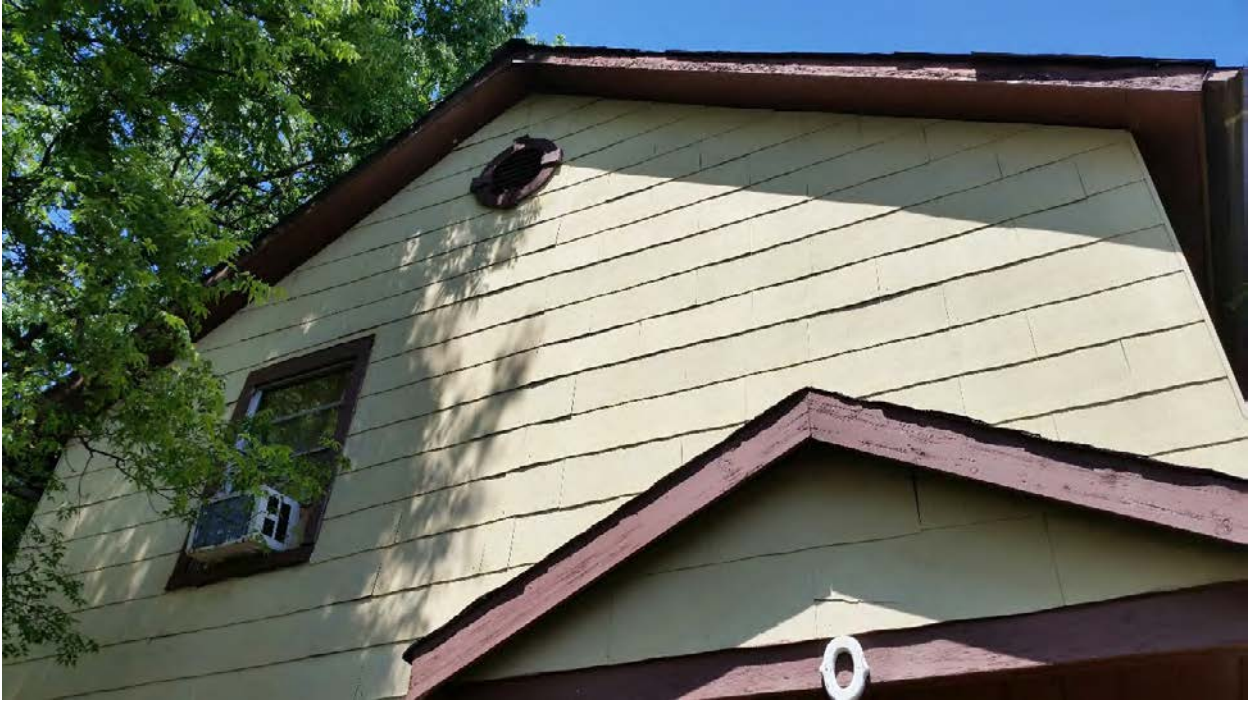
708 Morgan - Front second level showing covered window
