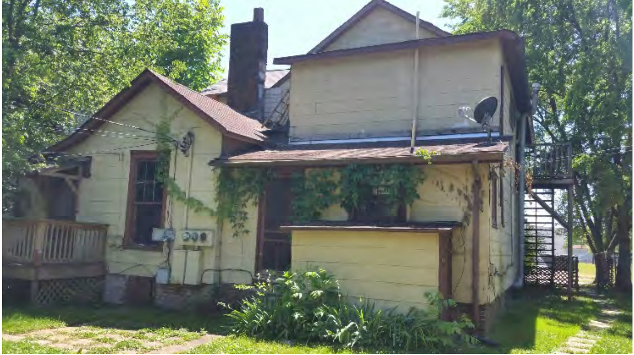
708n Morgan - Rear of house showing room for relocating fire stairs
