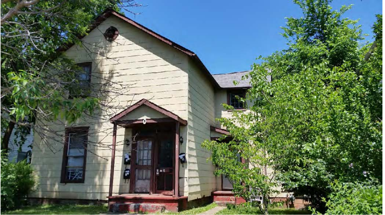
708 Morgan - Front façade
