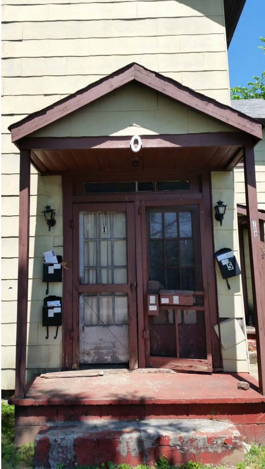
708 Morgan - Non-original French door front entry with pedimented stoop
