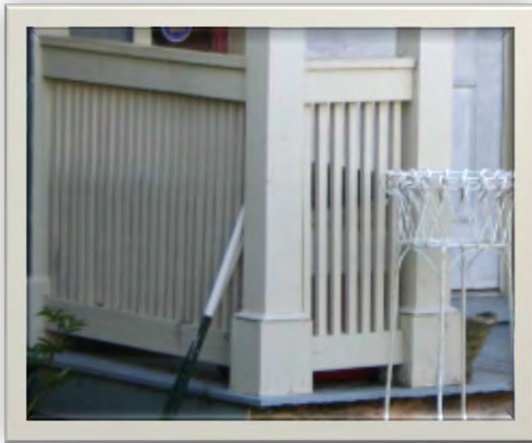
Type of porch post base proposed for 708 Morgan – 5 inches with canted top
