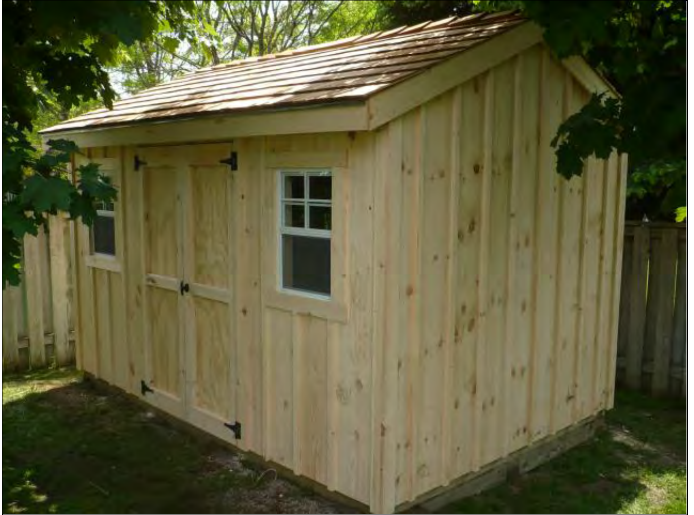
800 N. 4 th Avenue -- Example of shed type with board and batten sheathing (no windows proposed)
