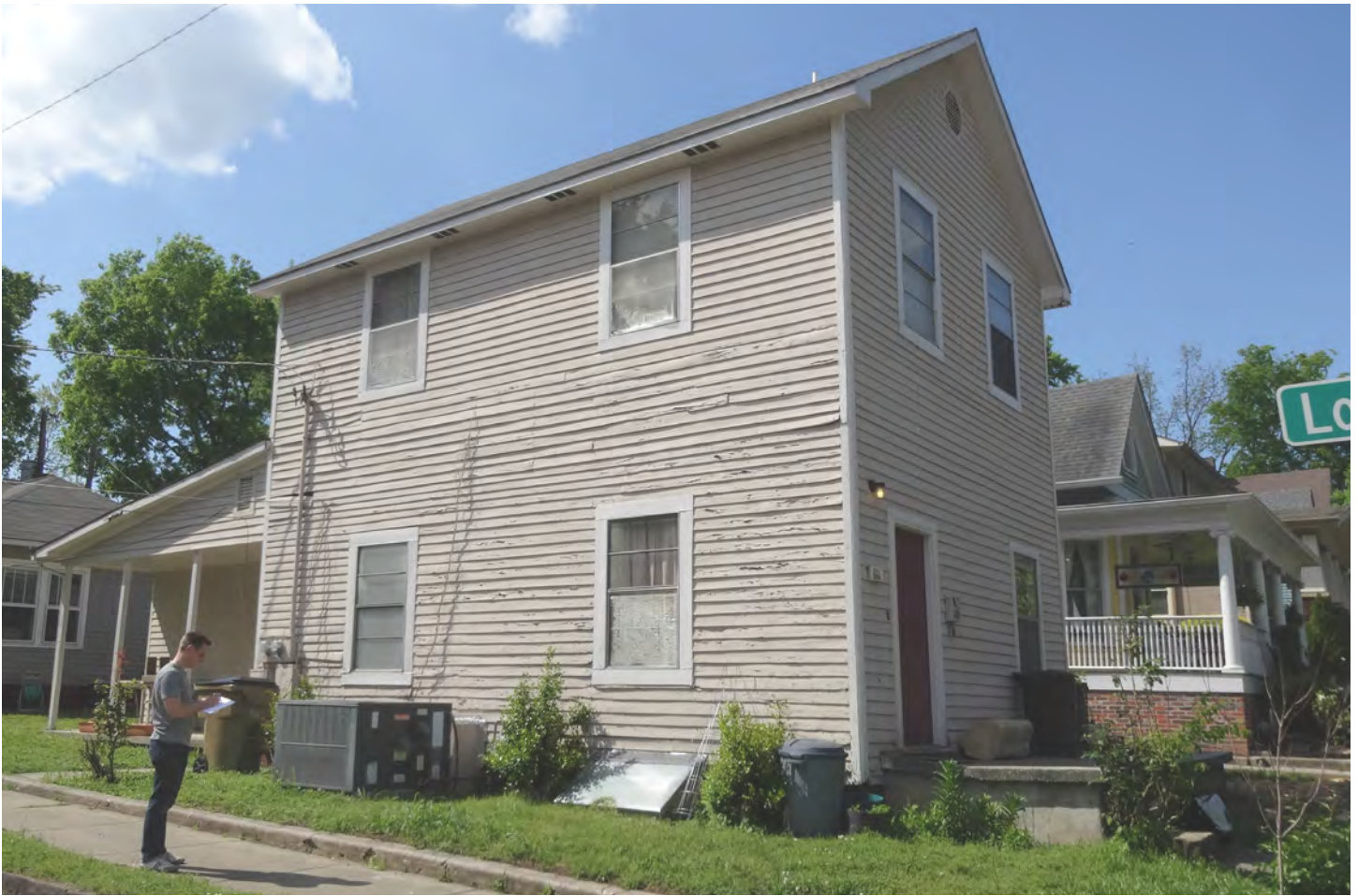
EXISTING CONDITIONS: VIEW FROM CORNER OF ELEANOR & LOVENIA
