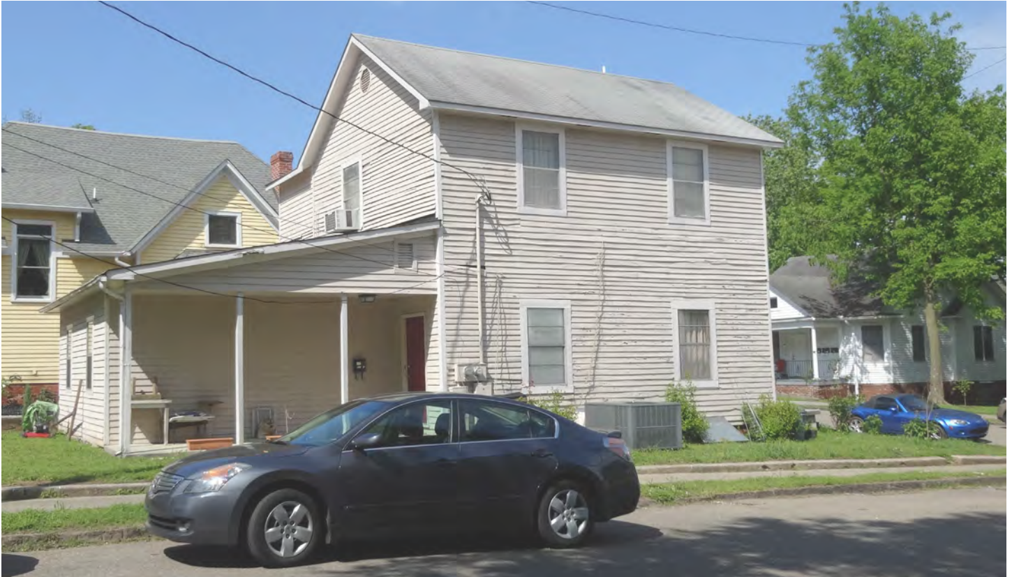
EXISTING CONDITIONS: SIDE ELEVATION (FACING LOVENIA ST.)
