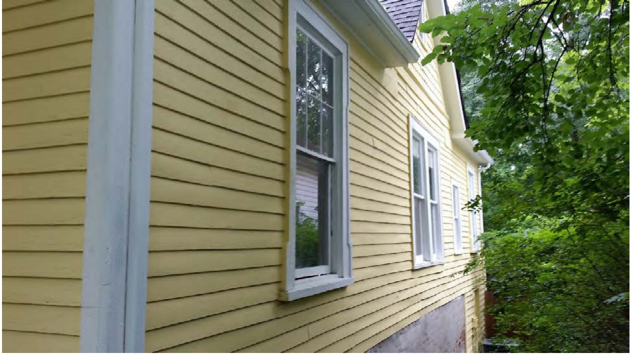
424 E. Oklahoma - SW side windows 4 & 5 from front corner
