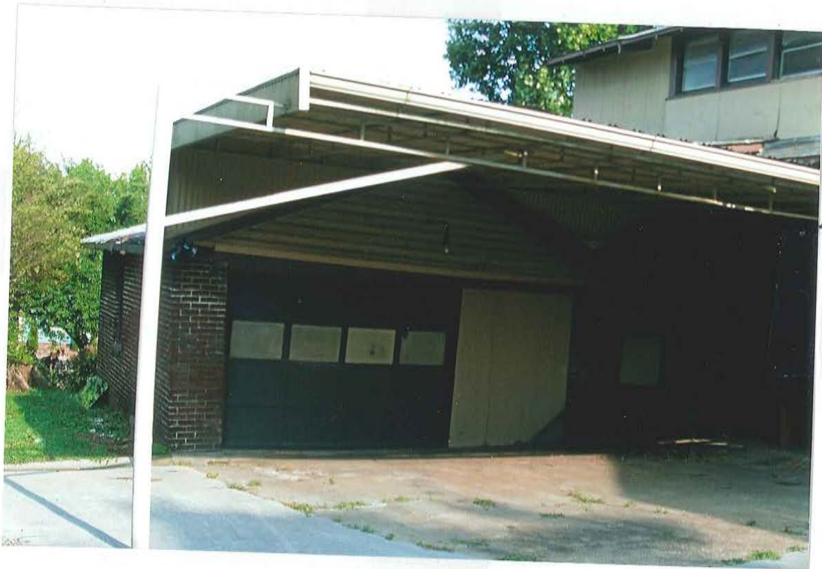
GARAGE/CARPORT ON BACKSIDE
