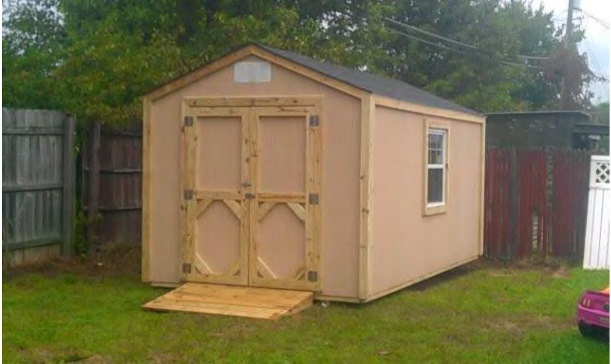
1701 Washington – Example of shed with 2 x 4 trim
