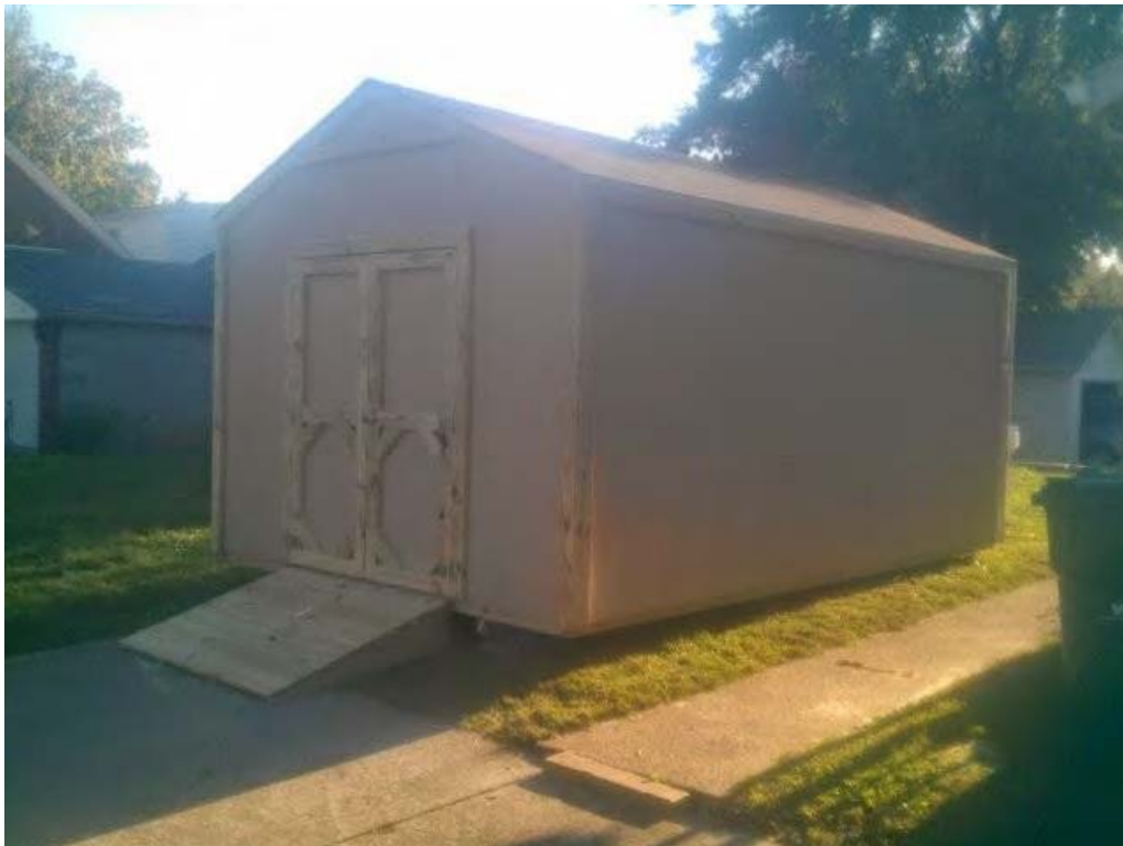
1701 Washington – Example of shed with no window and louvered vent gable
