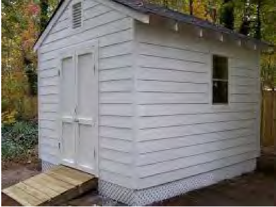
1701 Washington – Example of shed with overhang and lattice underpinning
