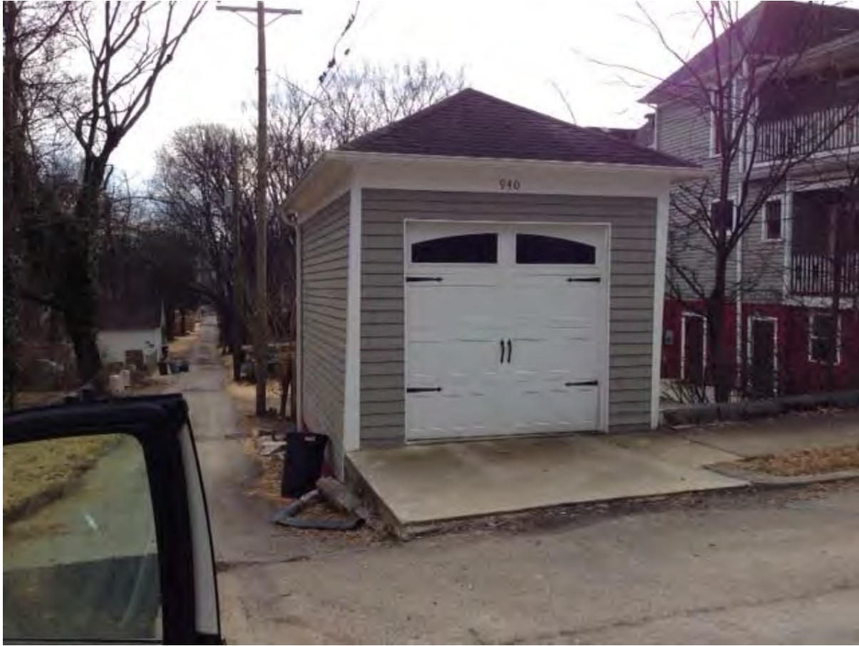
Example of pyramidal roof accessory structure with clapboard and carriage house door
