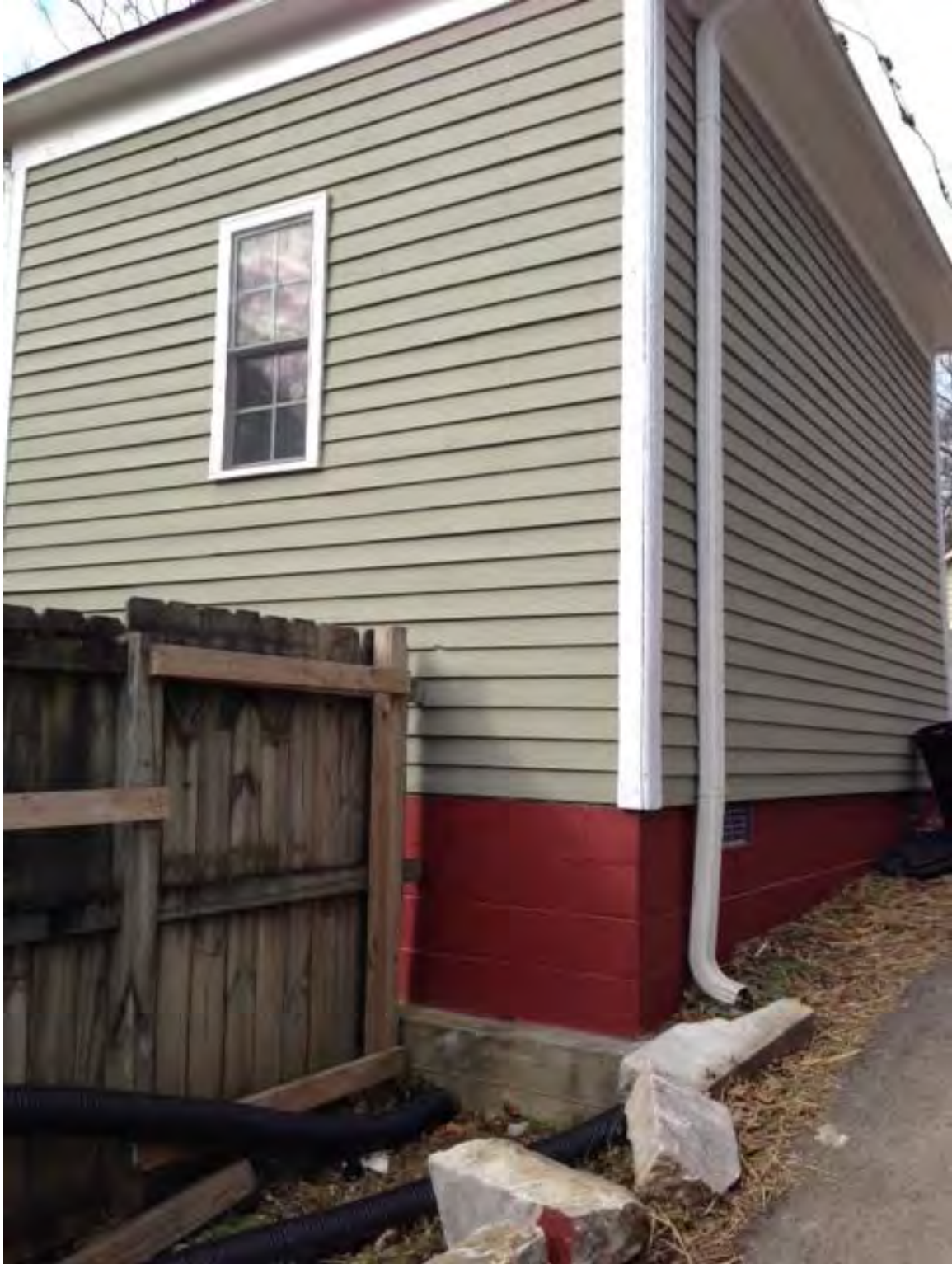
Example of corner trim and painted block foundation on accessory structure
