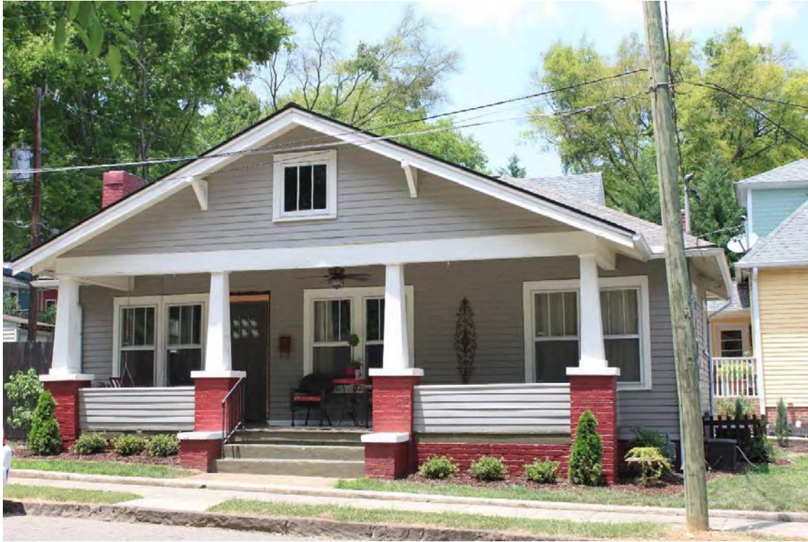
515 Lovenia – Front façade from street (windows on door have white marks)
