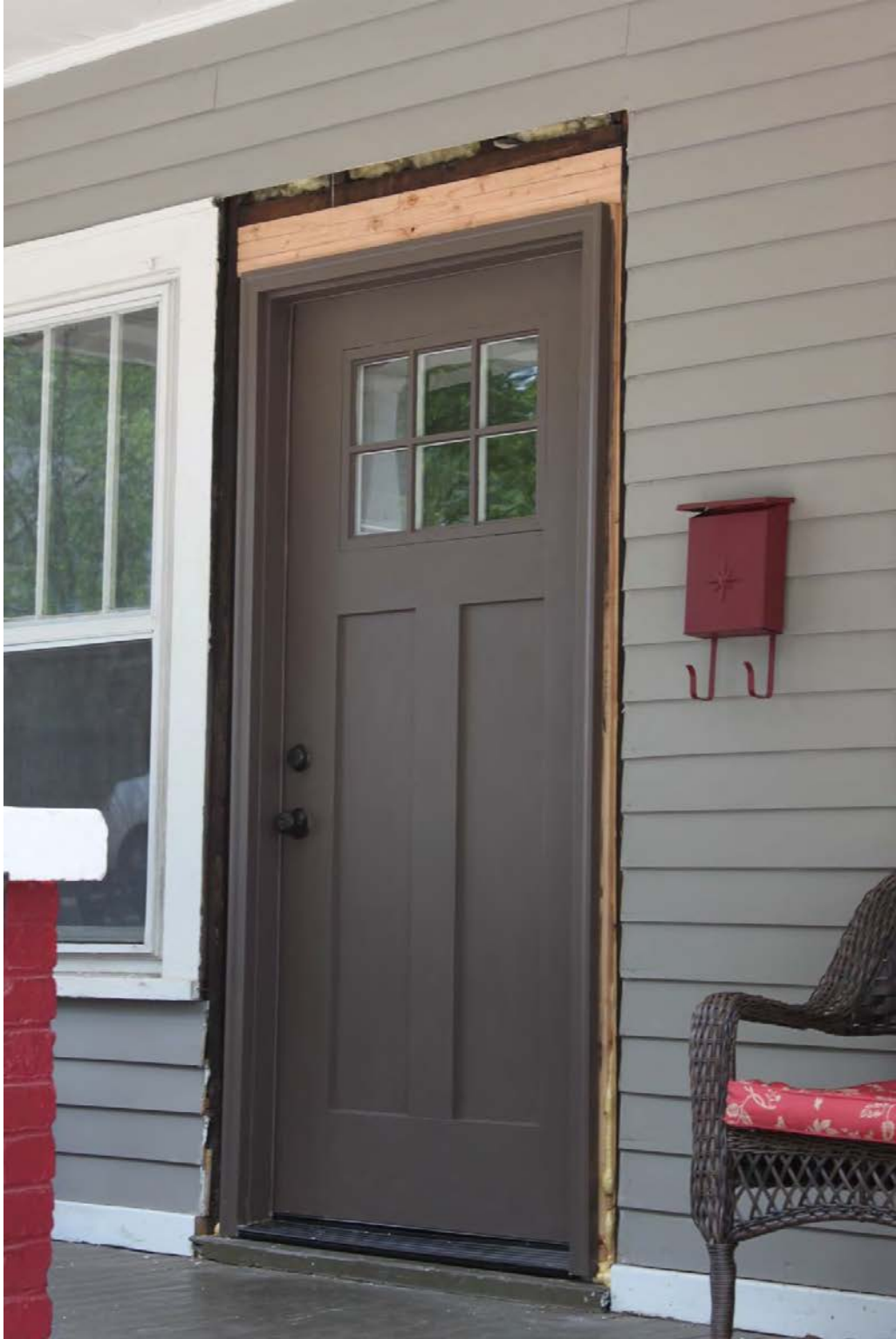
515 Lovenia – recently installed wood composite front door within existing opening
