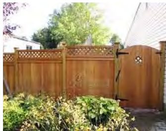
Std good neighbor fence with arch cut in an extra 2x6 above Std arbour and the gate build to match with an insert
