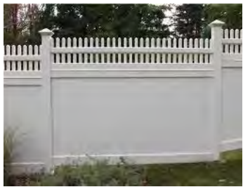
Std good neighbor fence with arch cut in an extra 2x6 above Std arbour and the gate build to match with an insert
