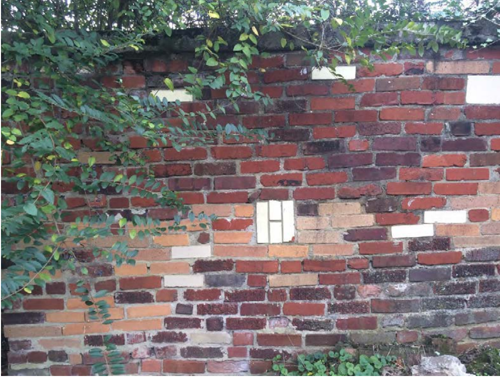
517 Oklahoma – Brick patchwork wall to be preserved
