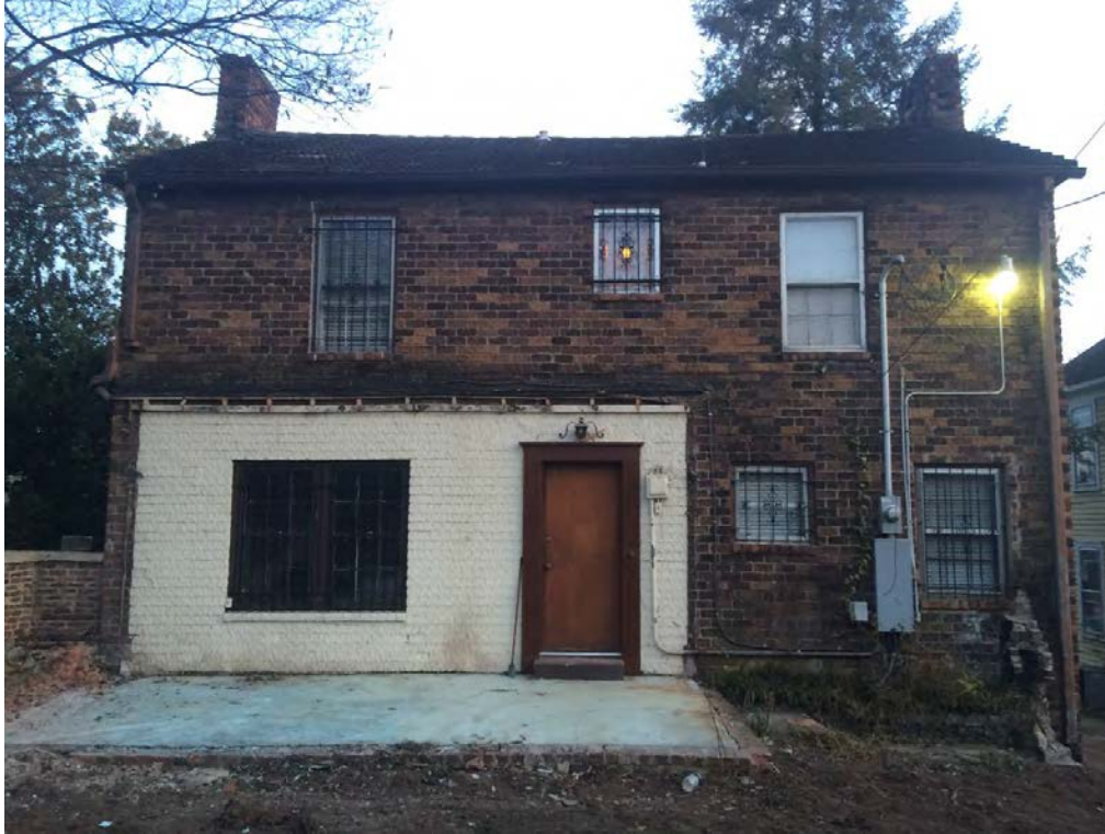
517 Oklahoma – Previously existing rear addition
