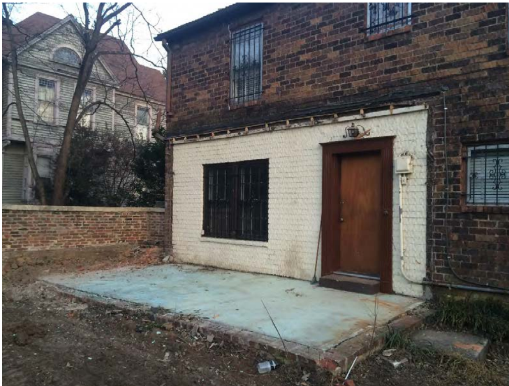
517 Oklahoma – Rear façade with addition removed
