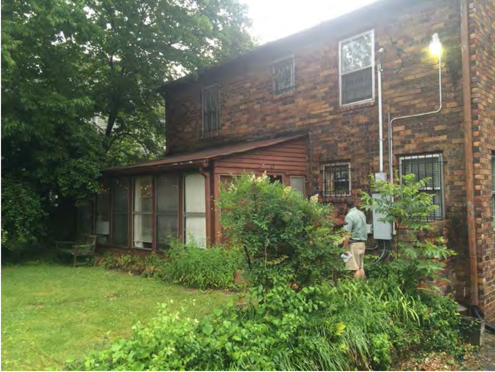
517 Oklahoma – Rear façade from SW with addition removed
