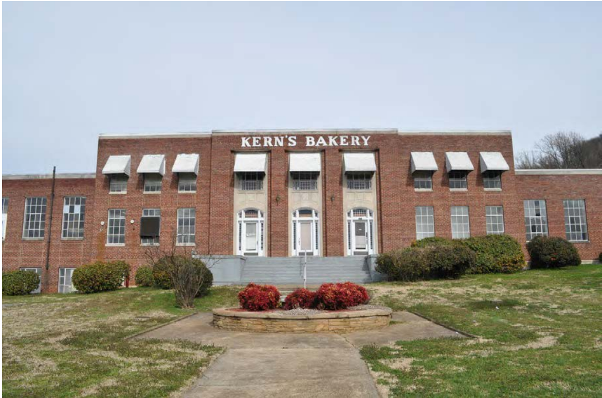
Kerns Bakery – Front façade, center section
