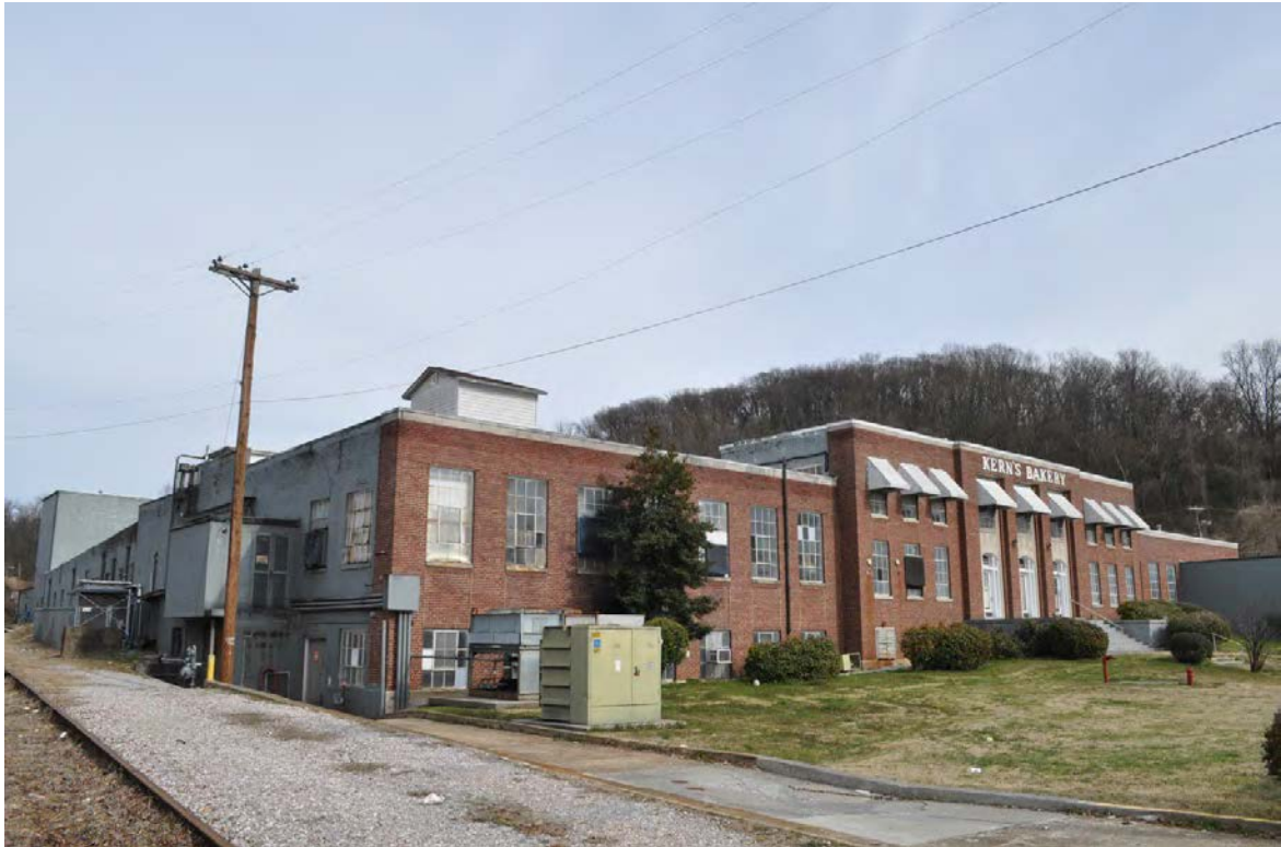
Kerns Bakery – North facade
