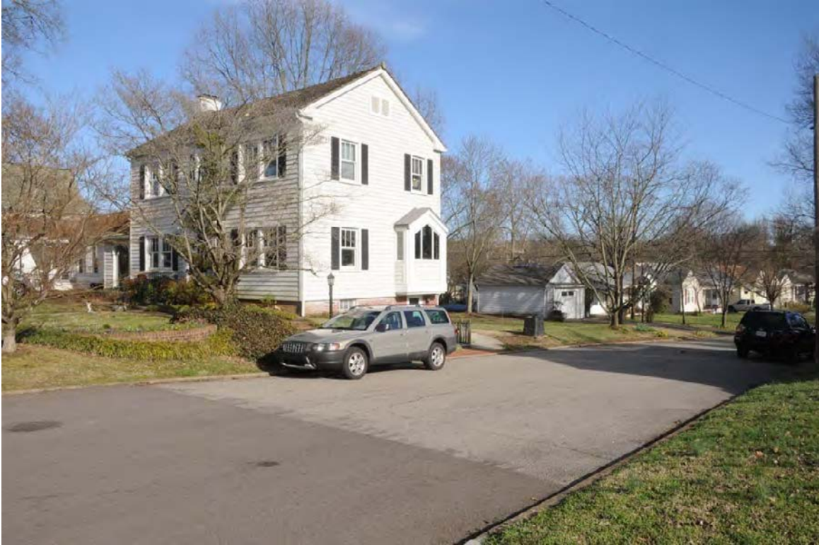
2100 Fairmont - View from the intersection of Miami Street with Fairmont Blvd.
