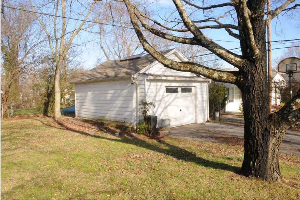
2100 Fairmont - View of existing garage from back yard
