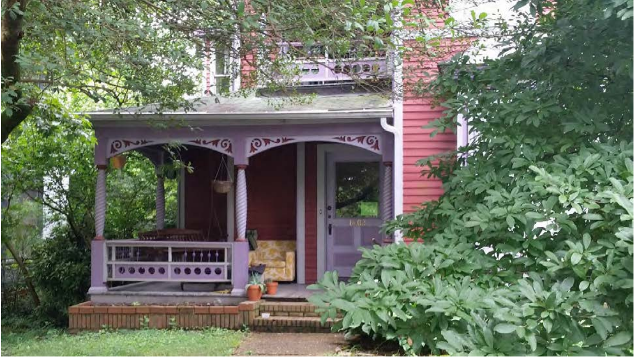
1802 Washington Ave. – Shingle front porch roof
