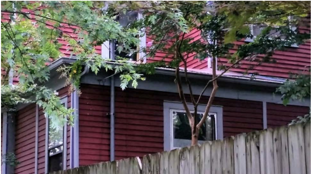
1802 Washington Ave. - Close-up of rear addition roof
