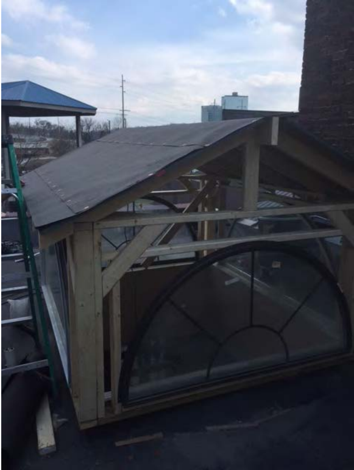
114 E. Jackson – Roof dormer under construction
