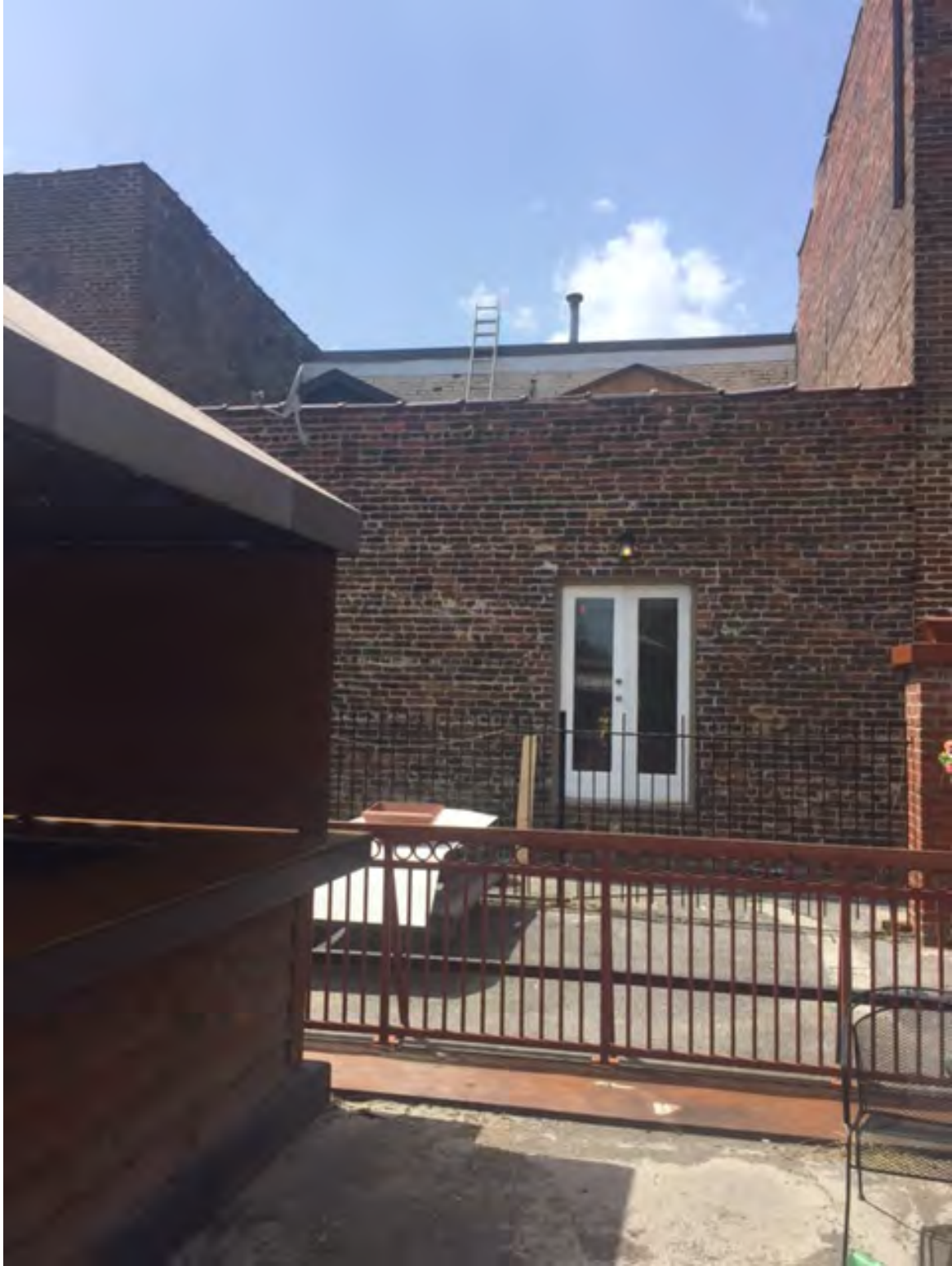
114 E. Jackson - Rear roof deck showing new pair of doors
