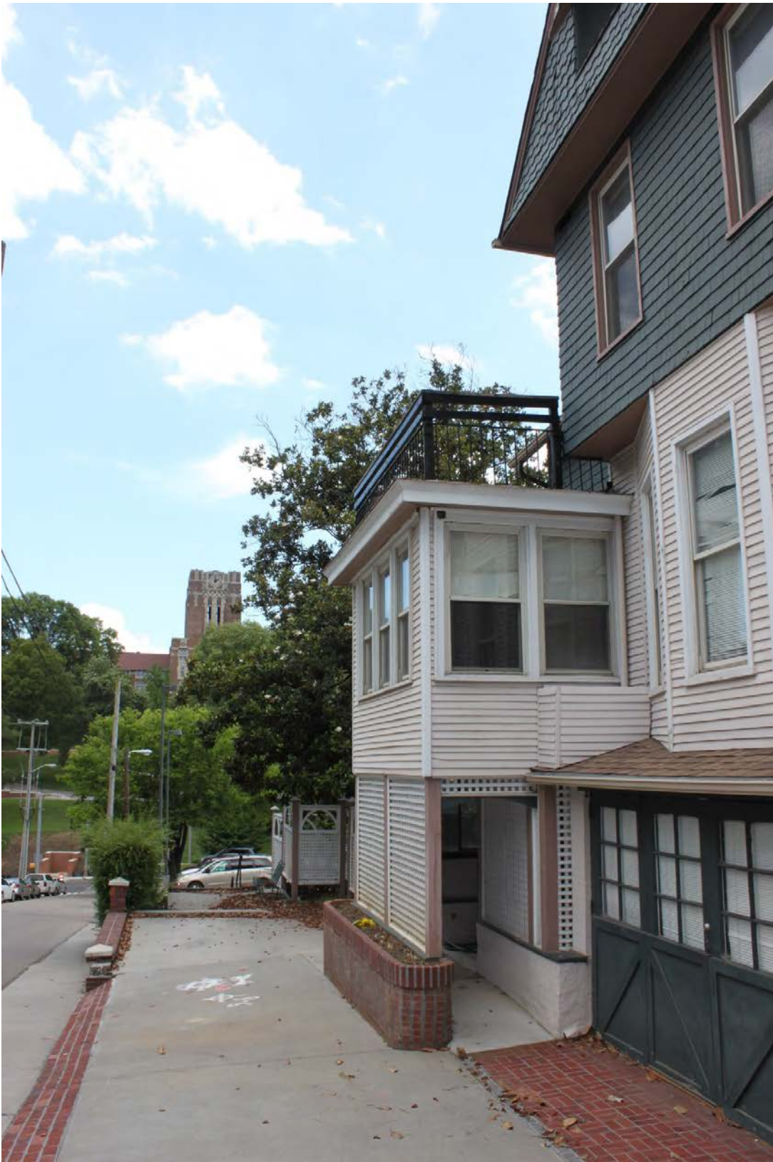
1302 White Avenue- East side looking south, showing removed addition
