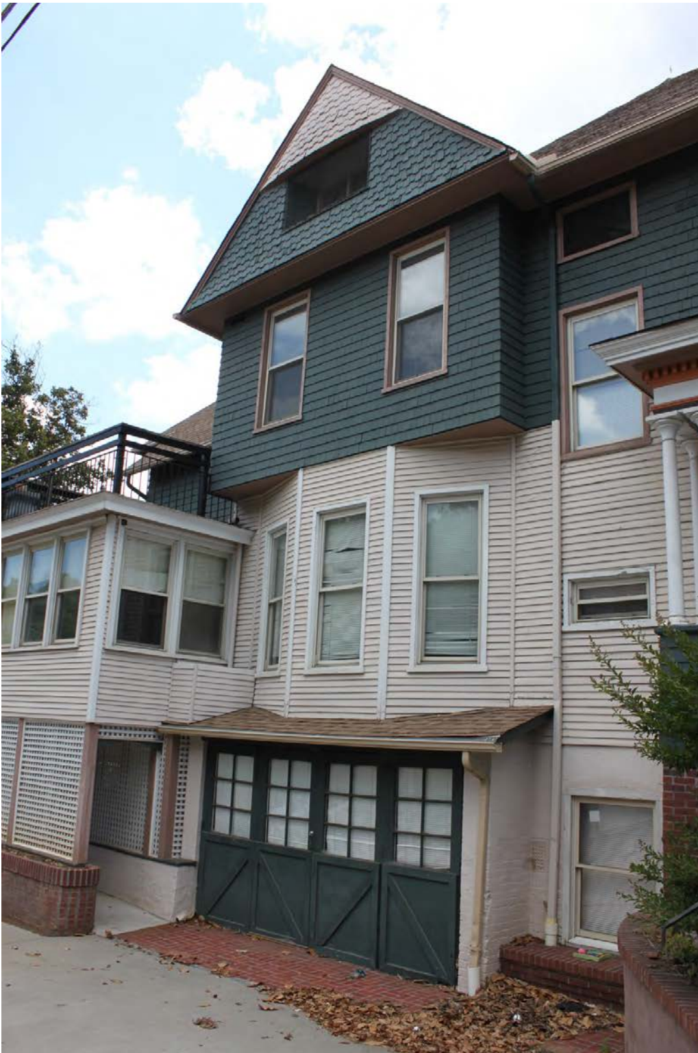
1302 White Avenue – East elevation – close-up
