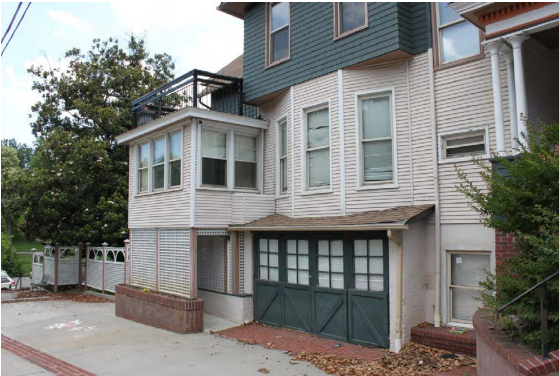
1302 White Avenue – East elevation showing removed addition
