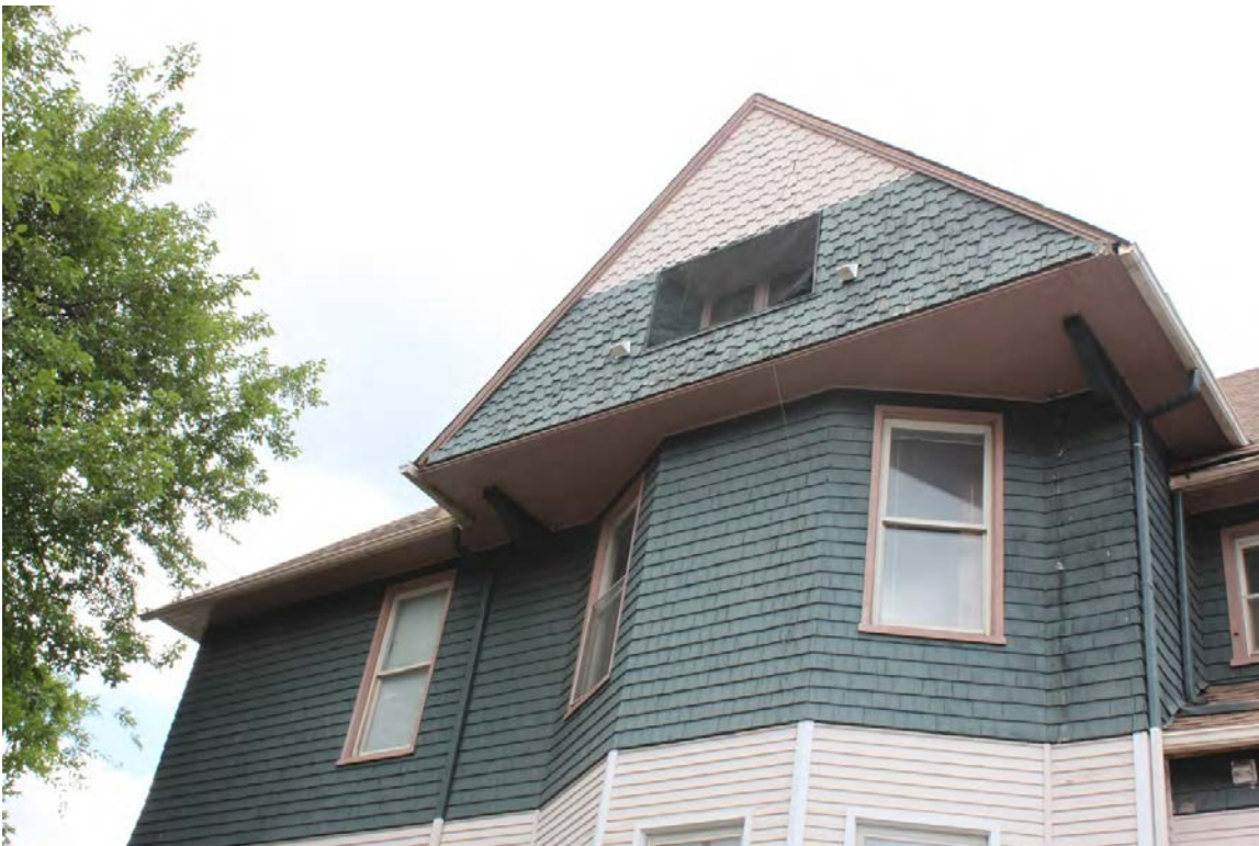
1302 White Avenue – West side gable, close-up
