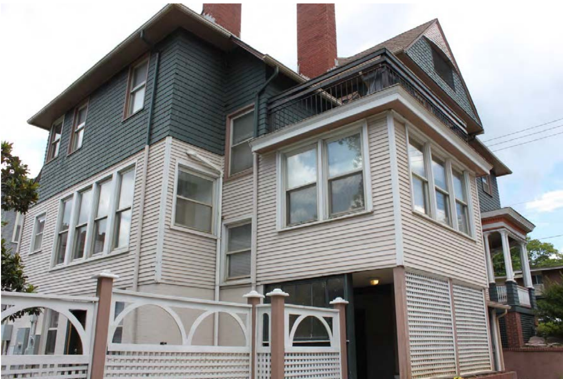
1302 White Avenue – South elevation (rear) showing removed addition
