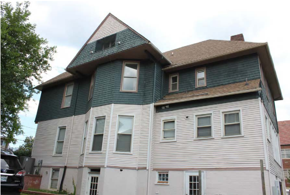
1302 White Avenue – West elevation
