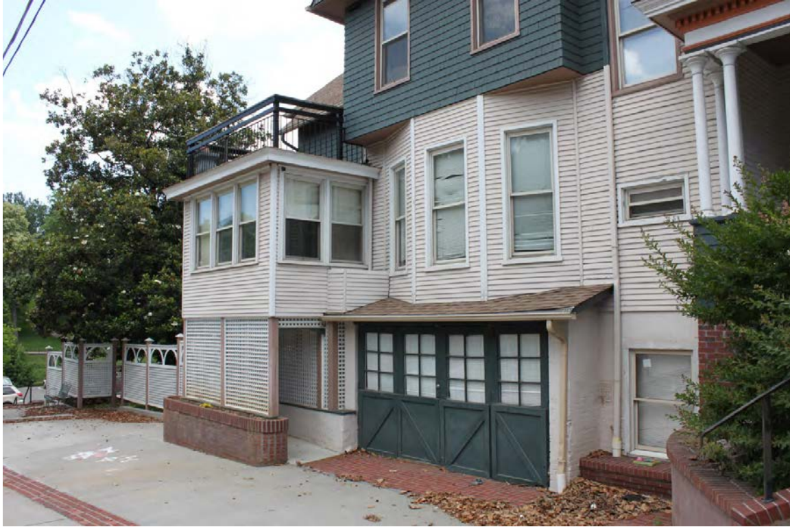
1302 White Avenue – East elevation showing removed addition
