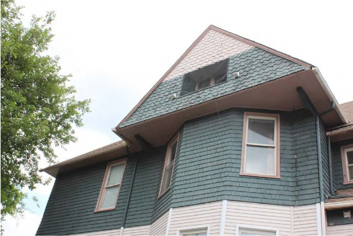
1302 White Avenue – West side gable, close-up
