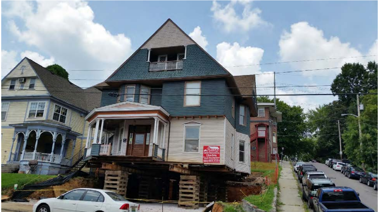
1201 Clinch Avenue looking north up 12th Ave.
