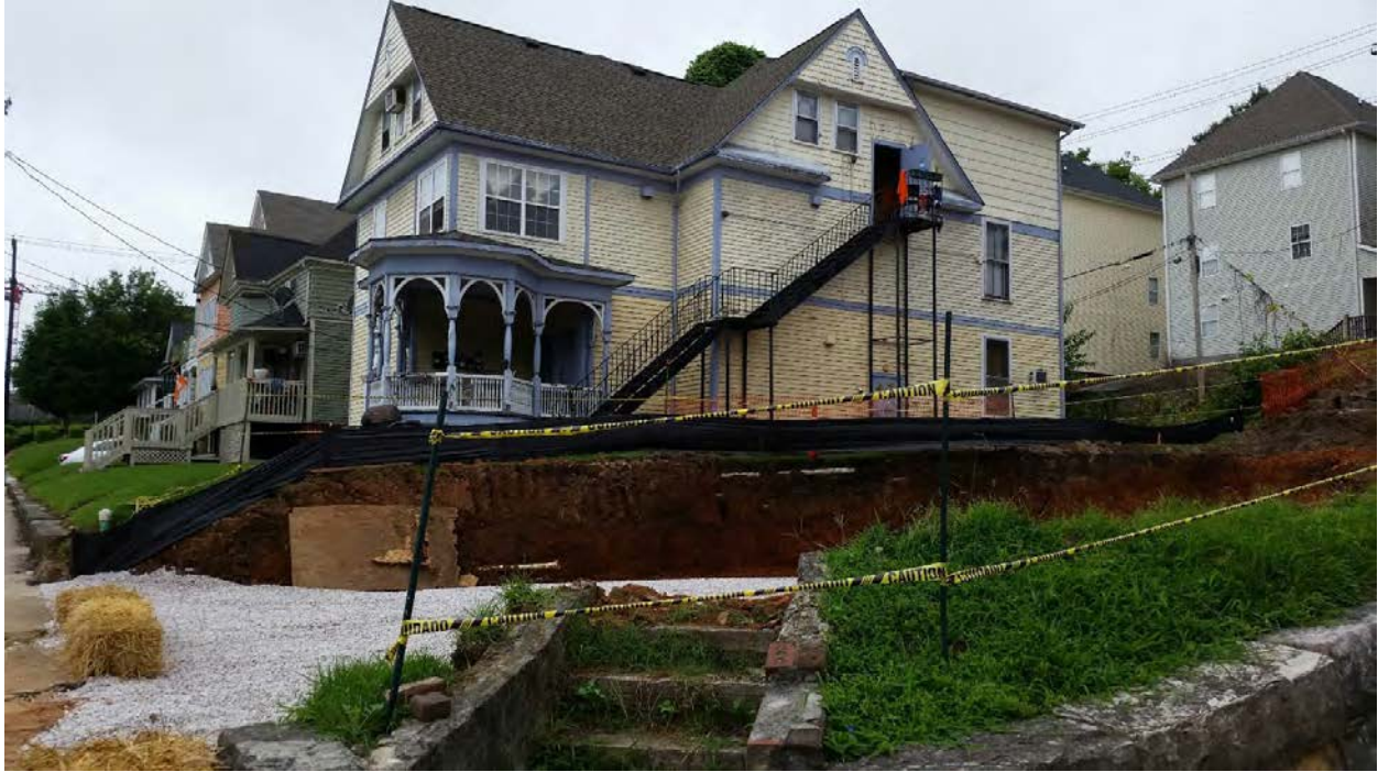
1302 White to 1201 Clinch - View of site from 12th St.
