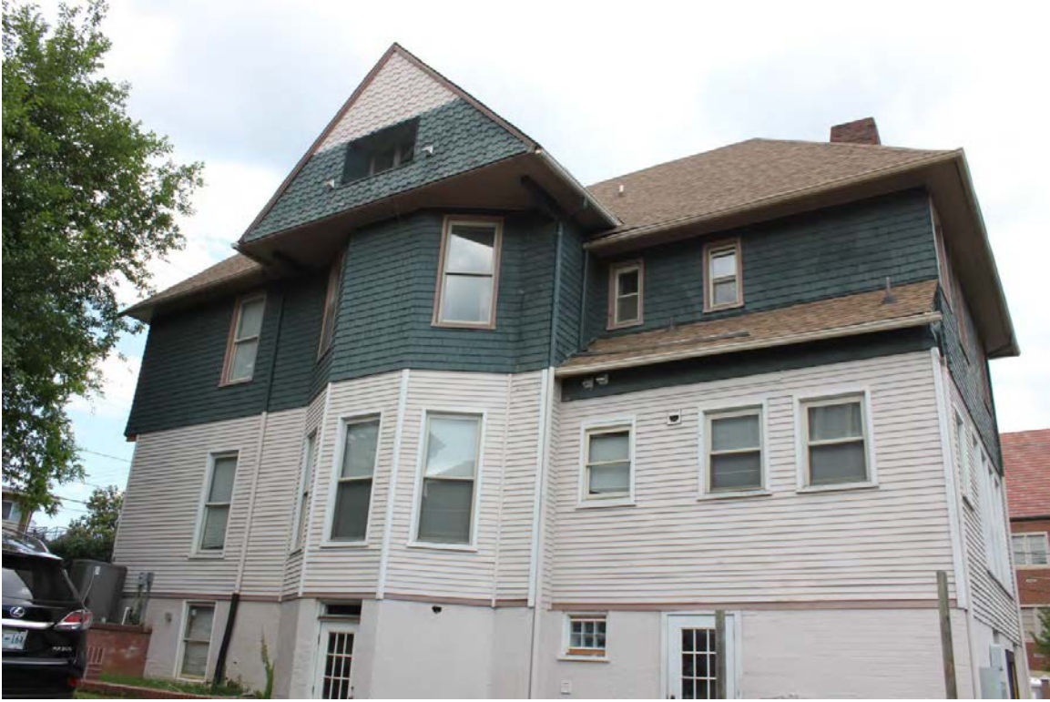
1302 White Avenue – West elevation
