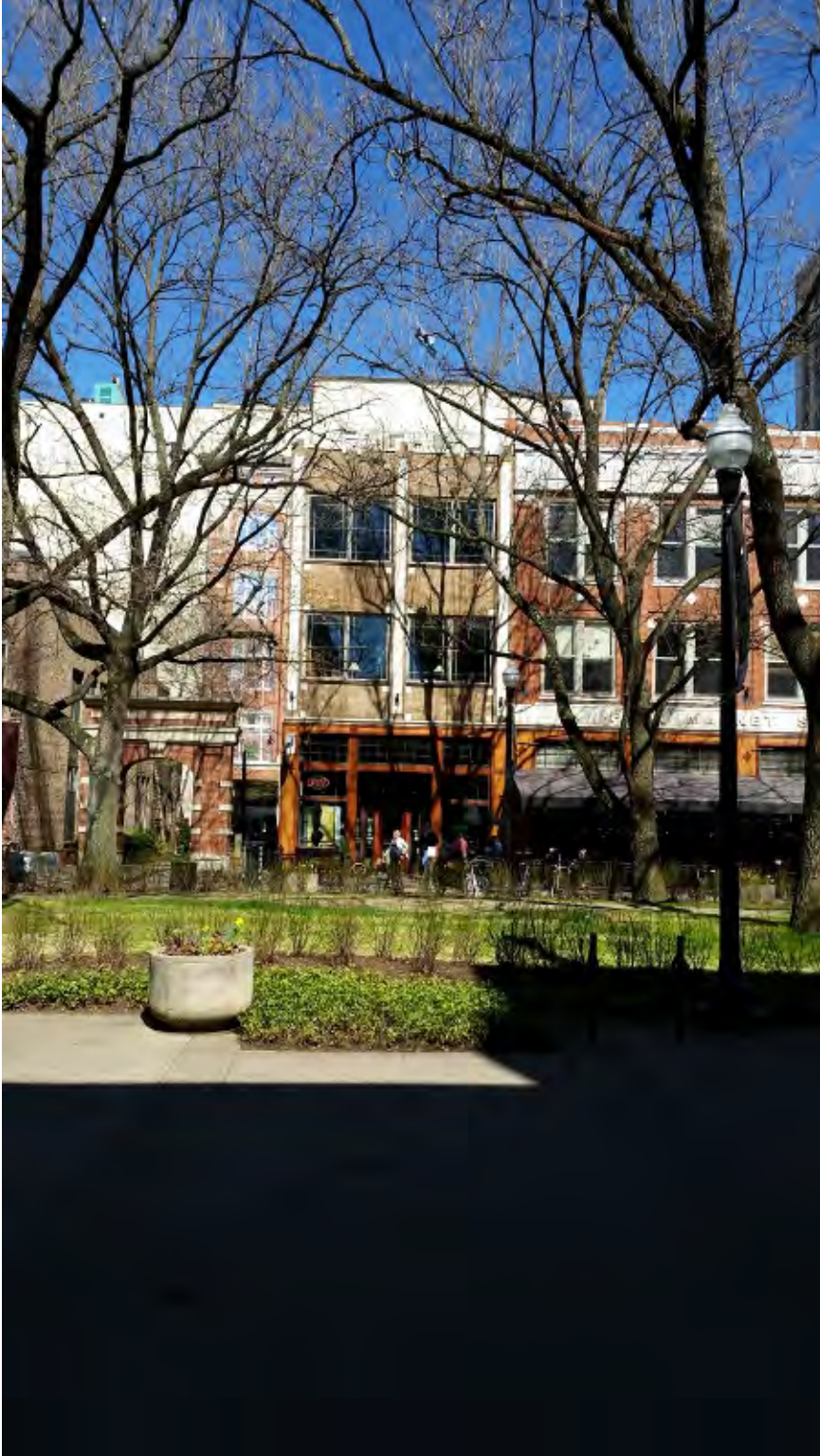
Example of brick parapets #1
