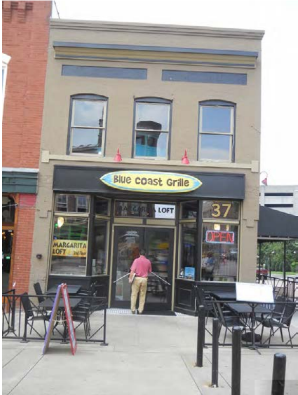
Example of brick parapets #3
