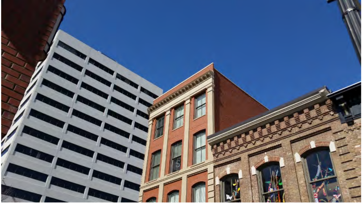
Example of brick parapets #2
