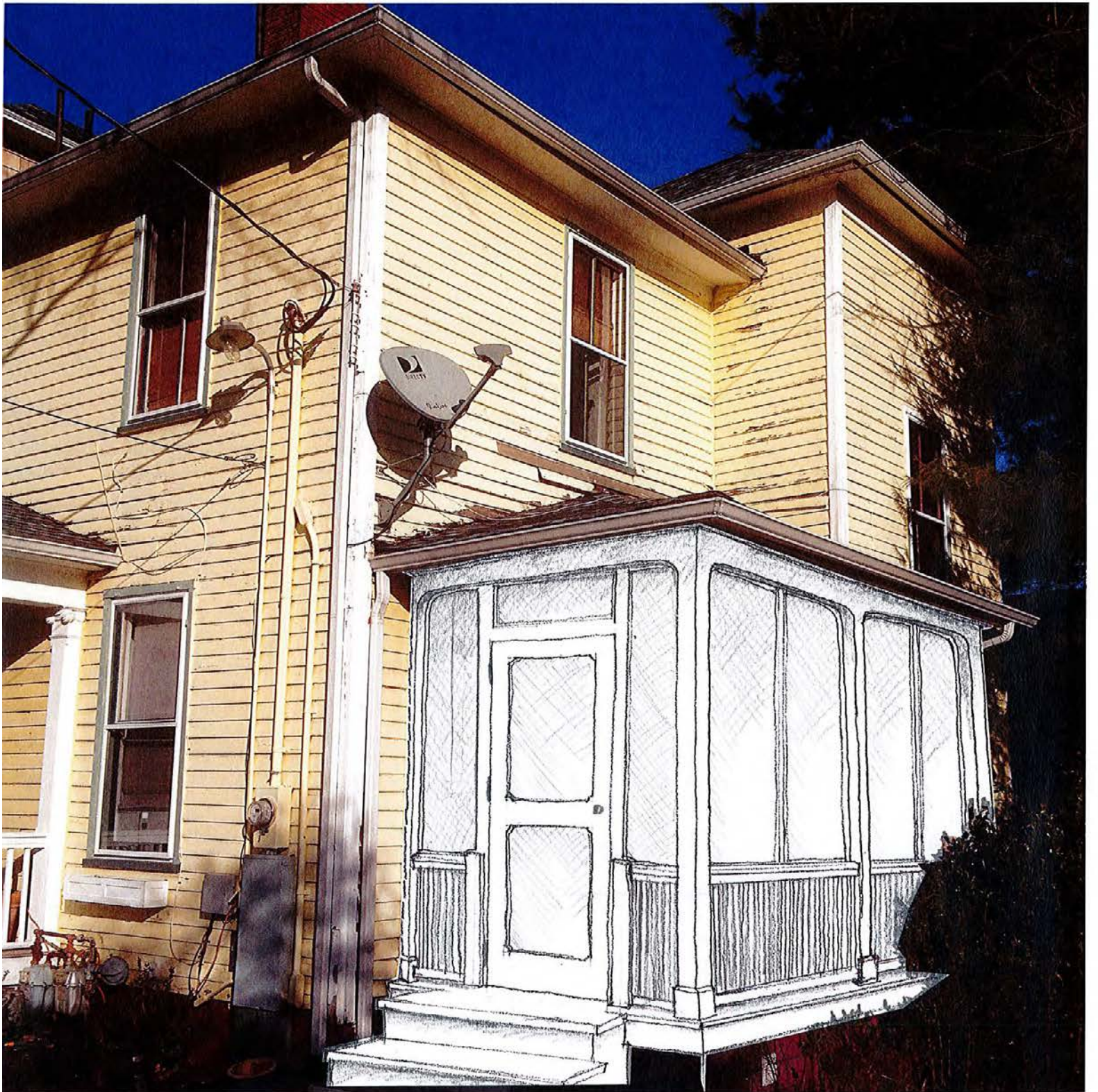
1000 Thompson Place - View of porch from southwest corner
