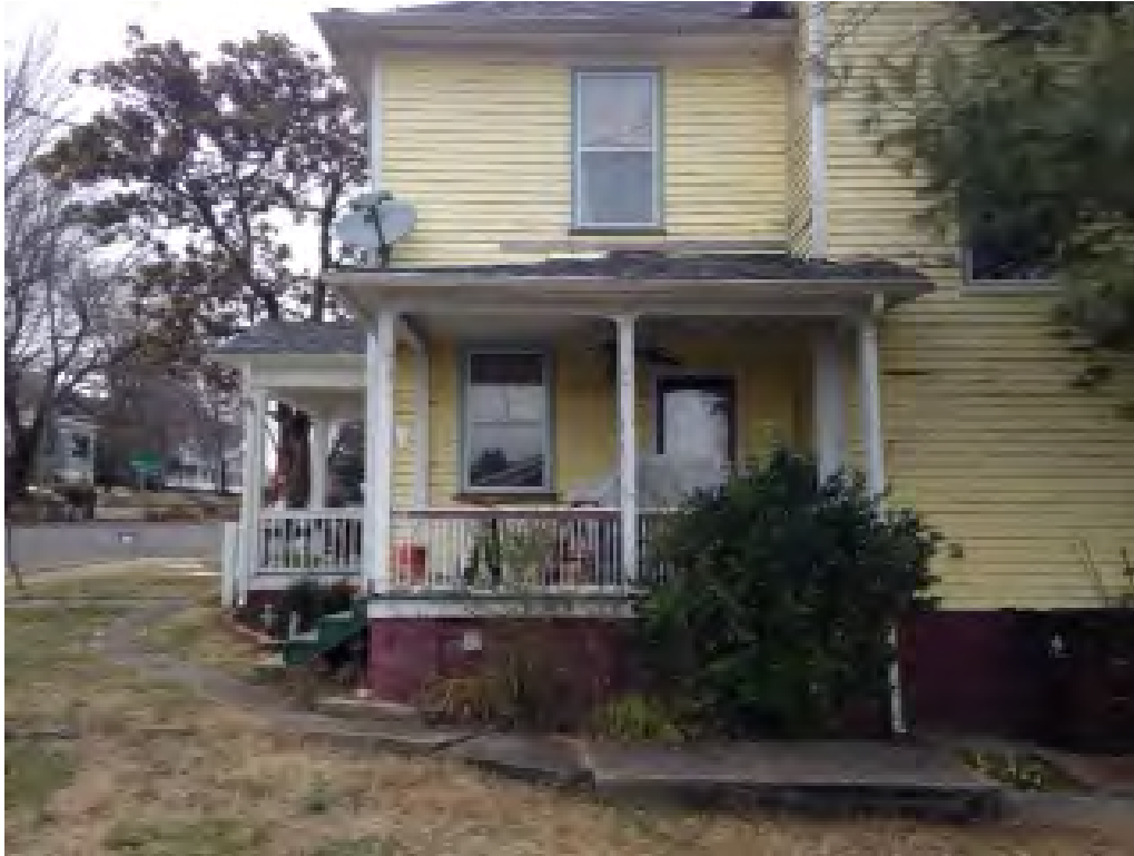
1000 Thompson Place – View of porch from rear (south)
