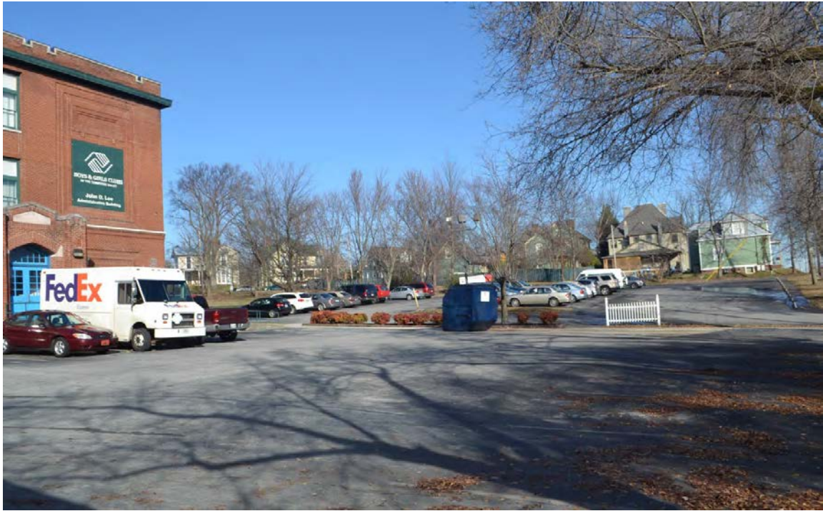
Moses School from east end looking northeast
