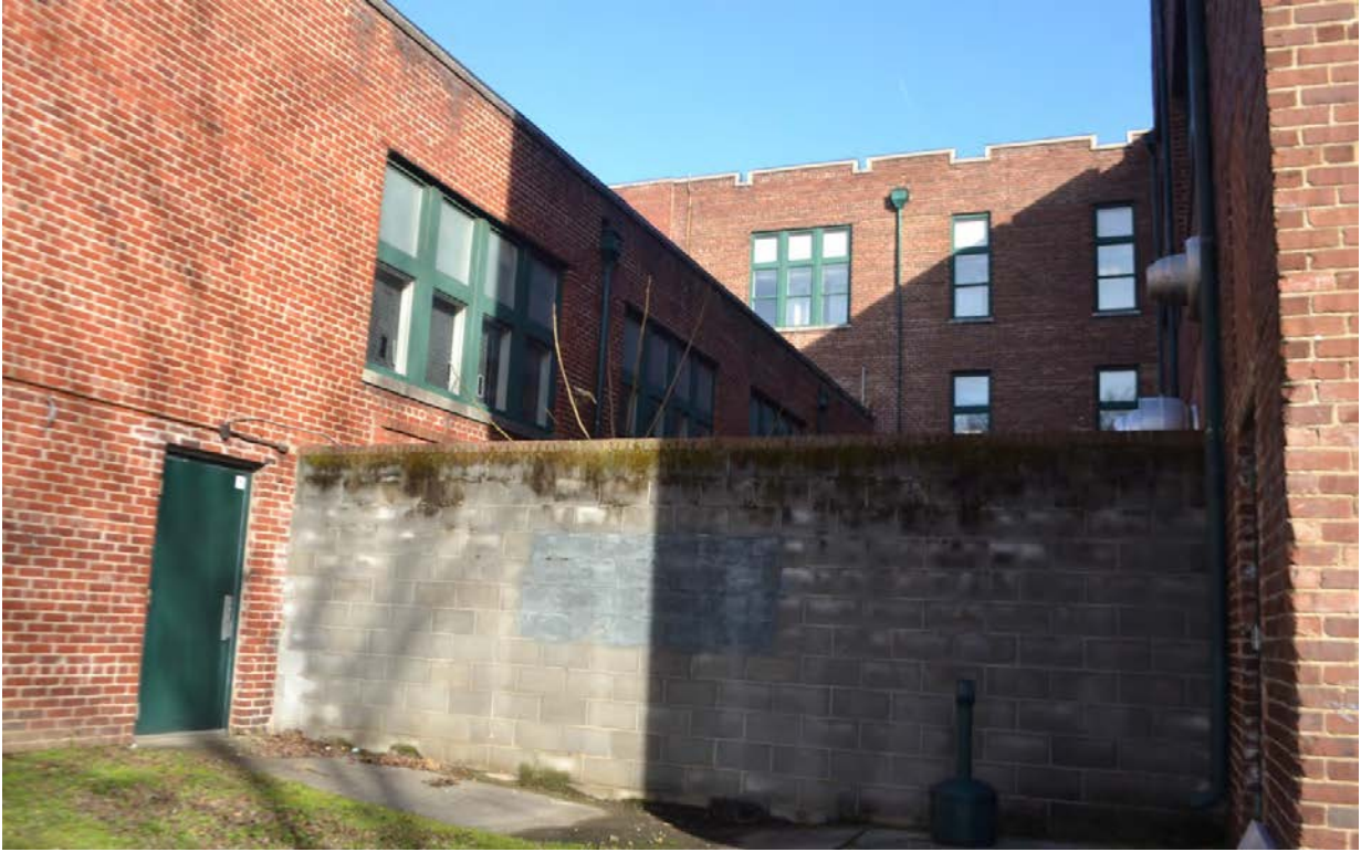
Moses School from rear (south side) looking toward location of gym
