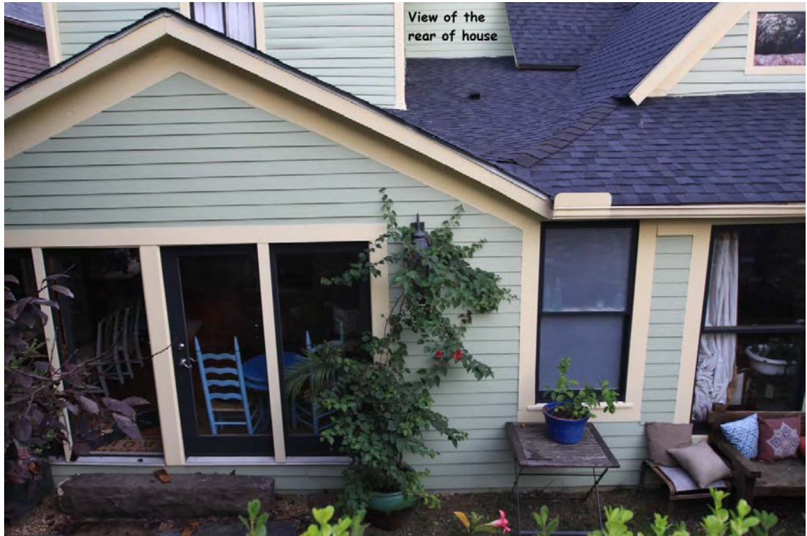
915 Luttrell - Rear of main house
