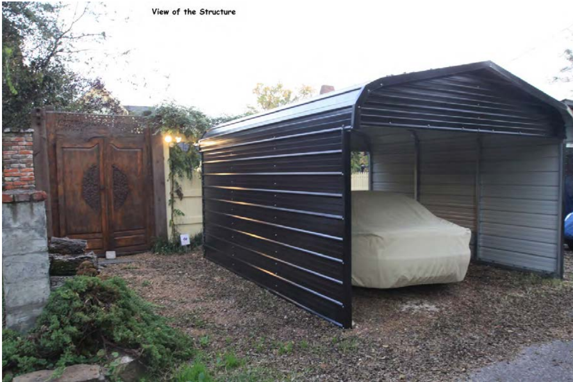
915 Luttrell - Installed accessory structure
