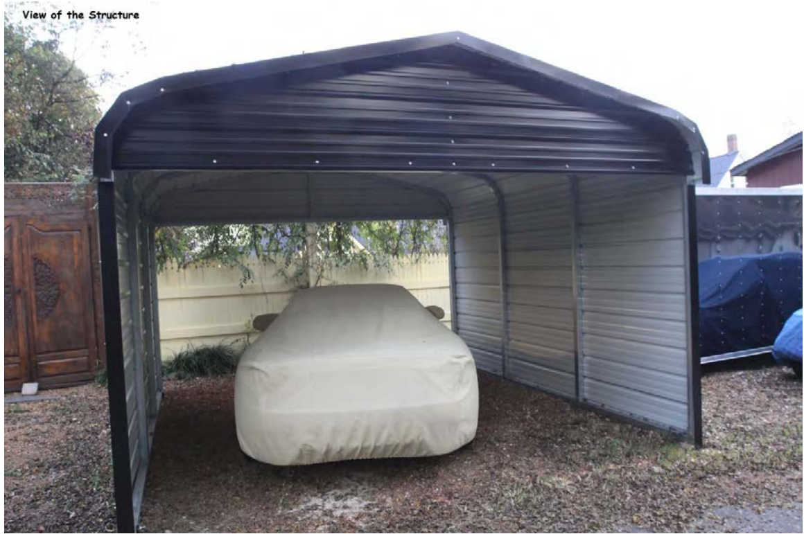
915 Luttrell - Installed accessory structure
