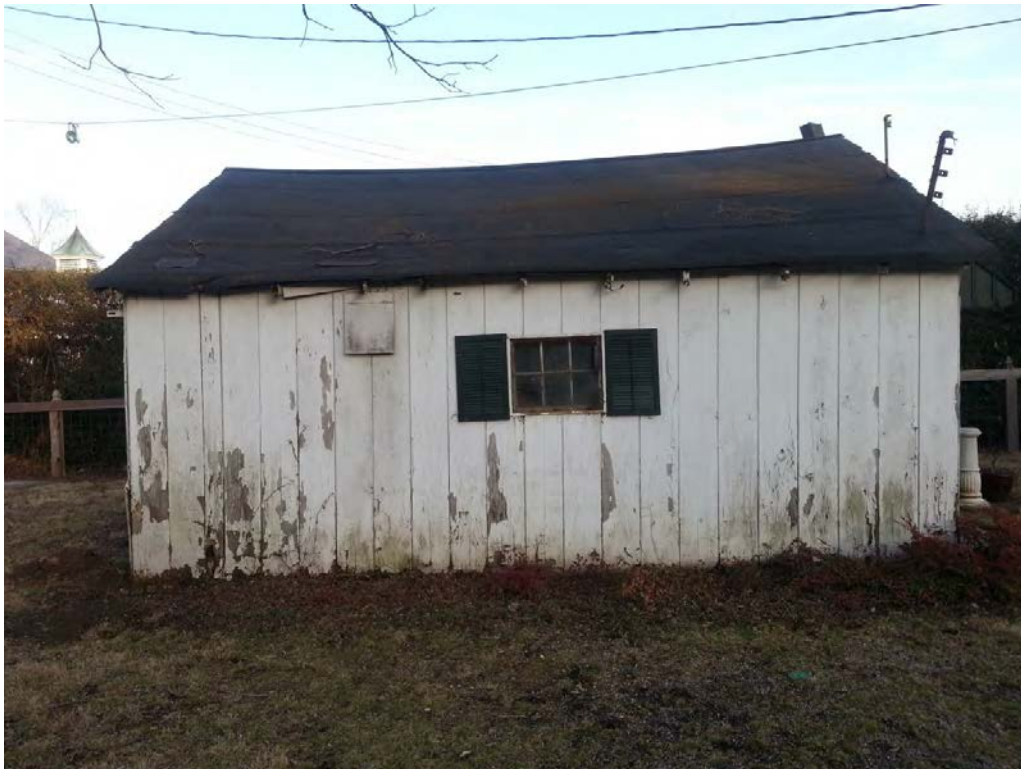
119 W. Glenwood garage - West elevation
