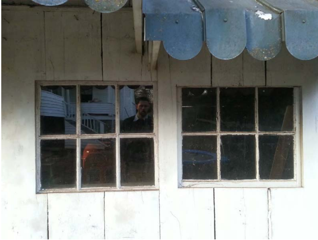
119 W. Glenwood - Front window detail
