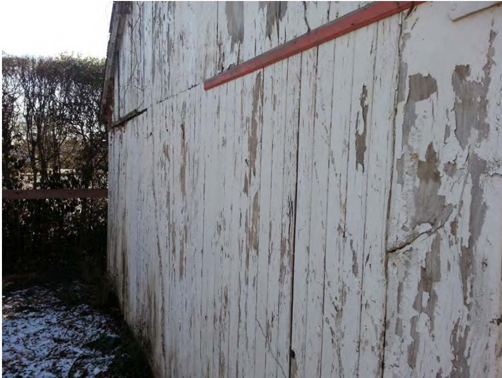
119 W. Glenwood - Alley-facing side
