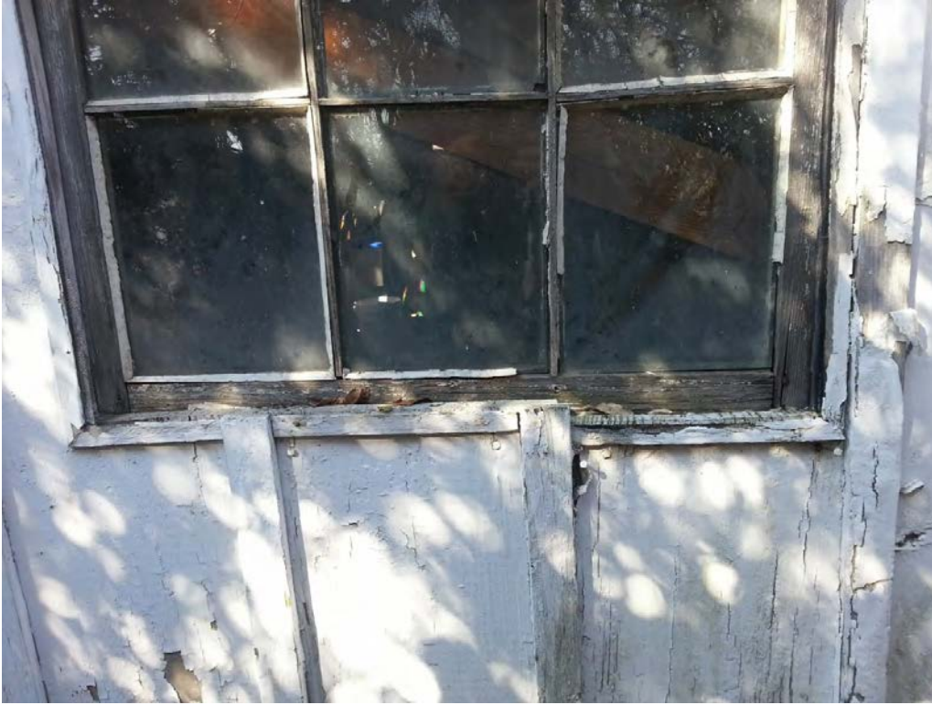
119 W. Glenwood - East window and board and batten close-up
