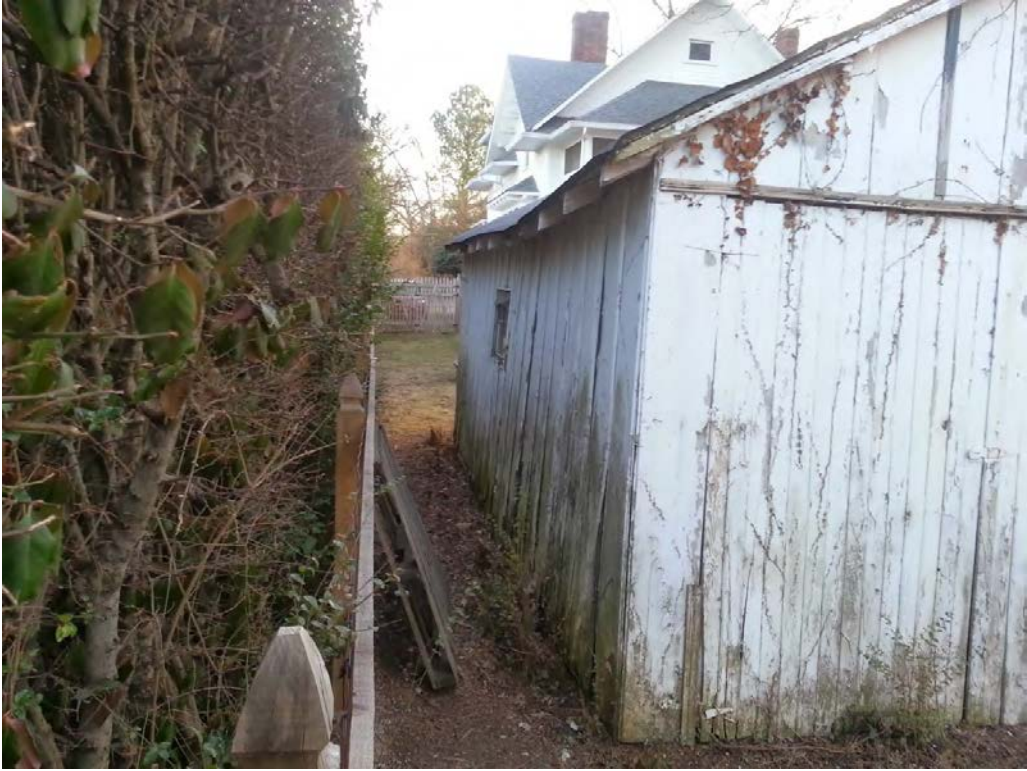
119 W. Glenwood - East side looking toward house
