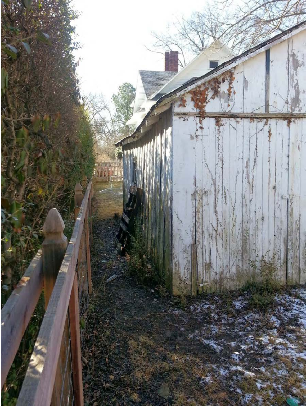
119 W. Glenwood garage - East side
