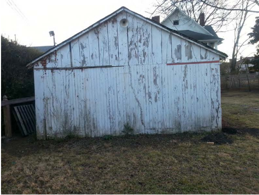
119 W. Glenwood garage - Alley elevation side
