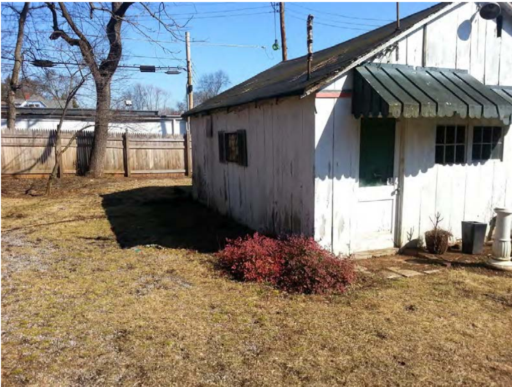
119 W. Glenwood - West and front elevations
