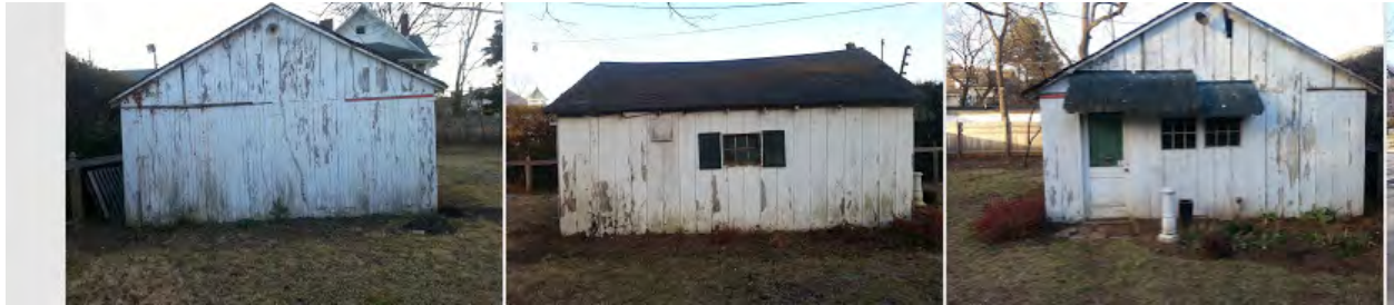
North side of structure (old carriage style doors on left half):
