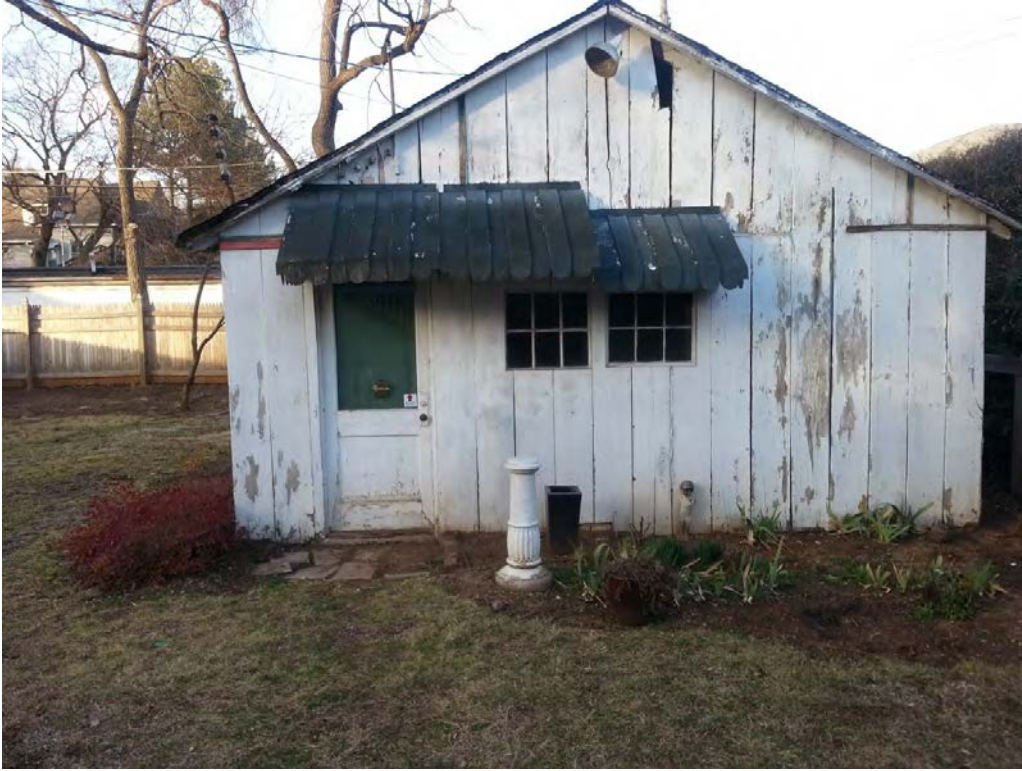
119 W. Glenwood garage - Street-facing elevation
