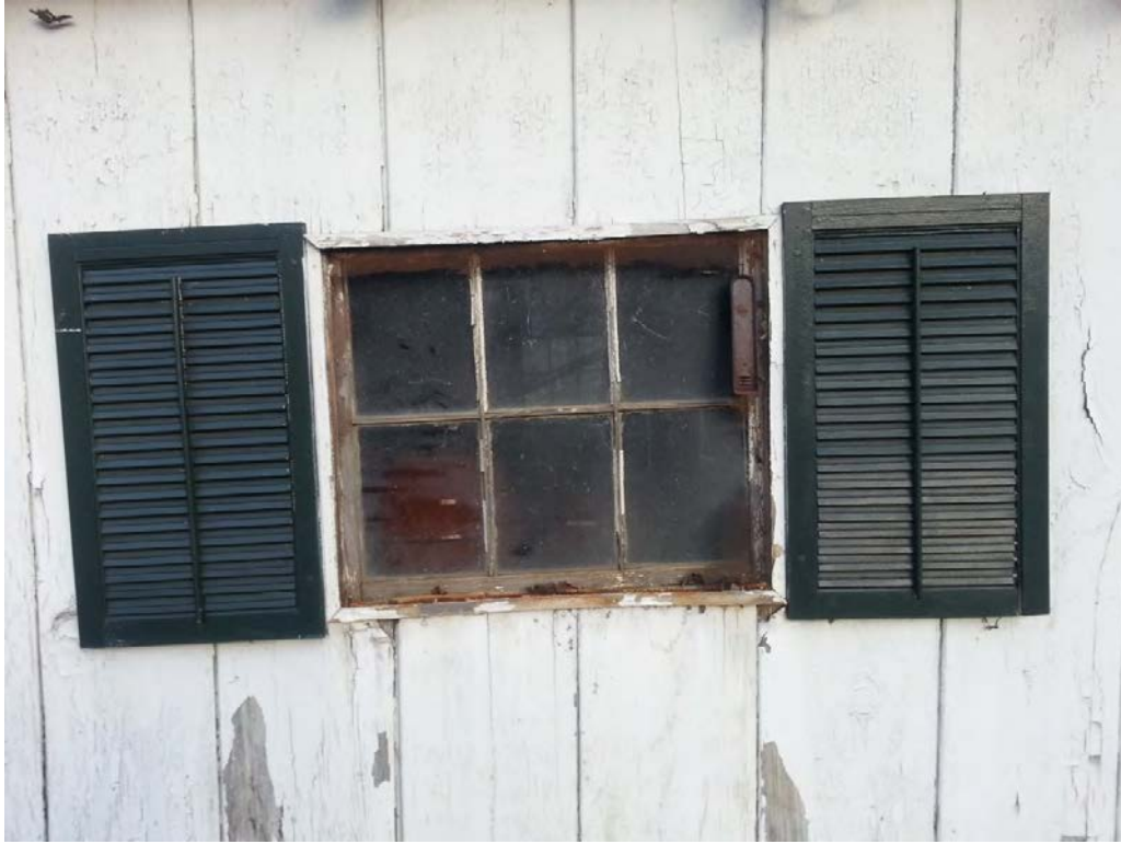
119 W Glenwood - Window on west side
