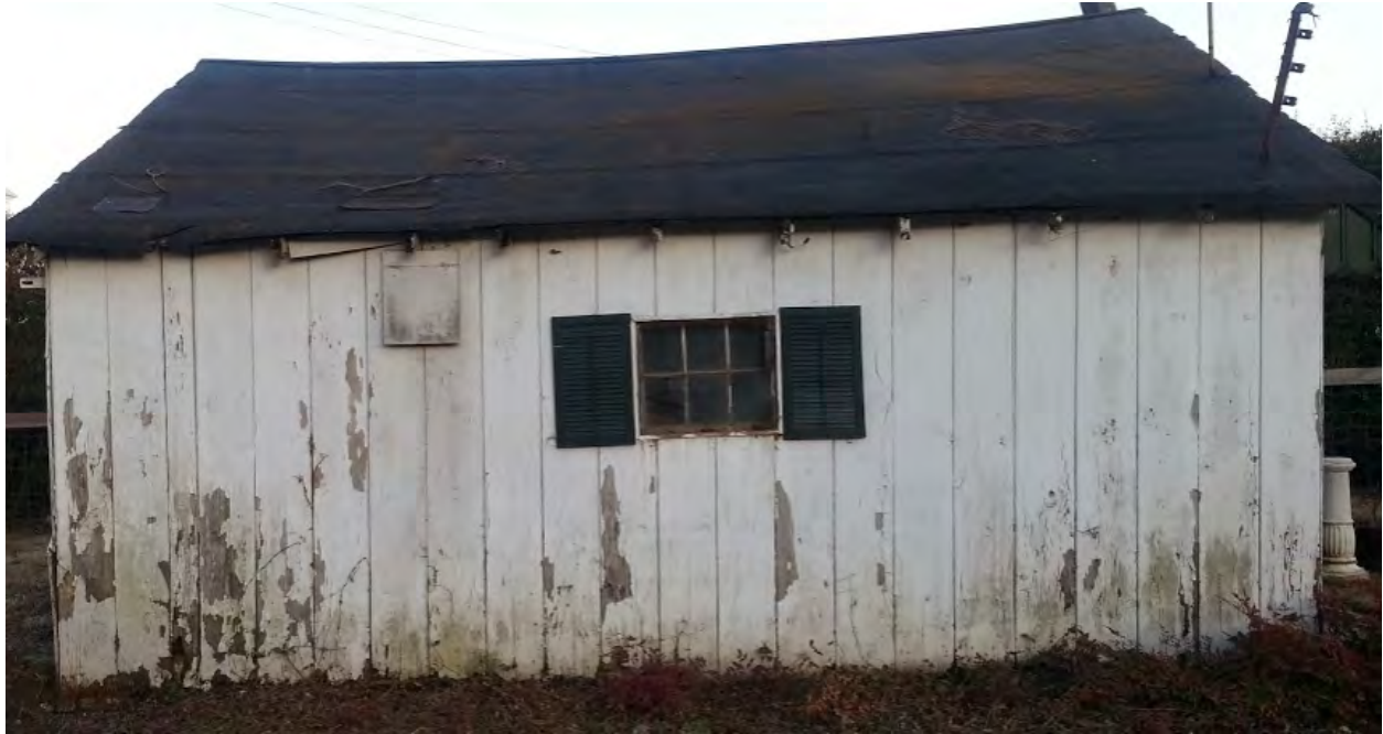
South side of structure
