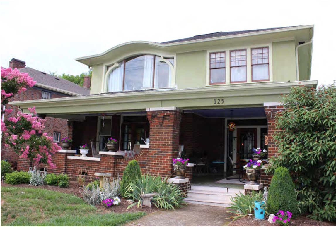
Subject property, south façade, 2014. 125 East Glenwood Avenue.
