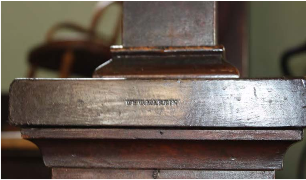
Staircase: Stamp of the stairbuilder. William Martin is listed in Knoxville city directories as a stairbuilder dating back to the 1870s.
