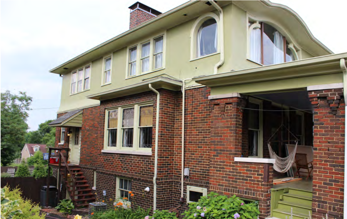
Subject property, west façade, 2014. 125 East Glenwood Avenue.
