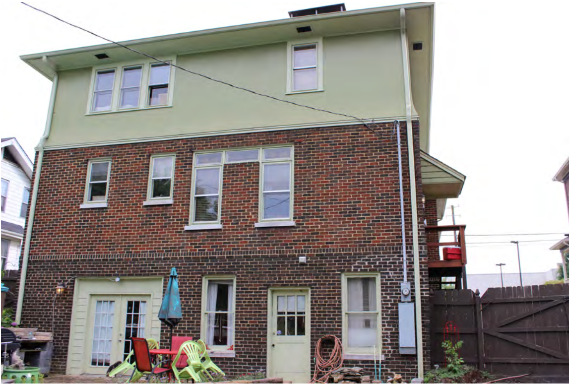
Subject property, north façade, 2014. 125 East Glenwood Avenue.
