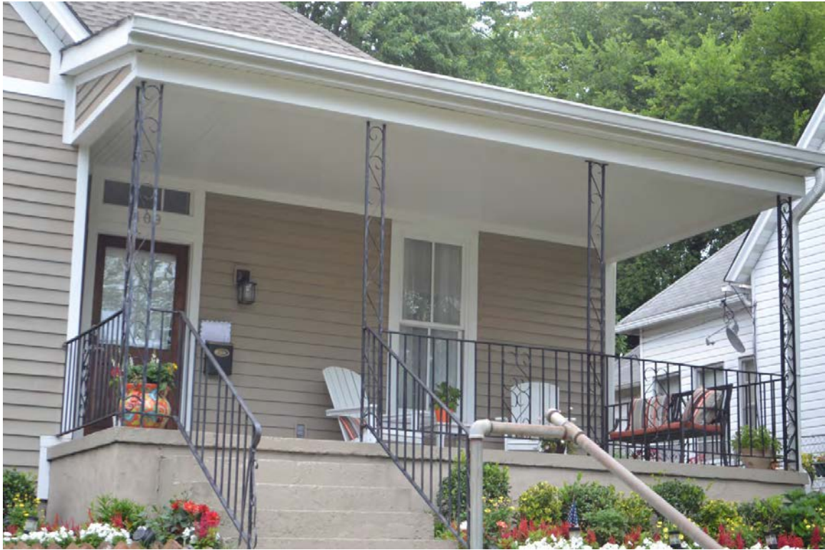
409 E. Oklahoma Ave. - Close-up of porch
