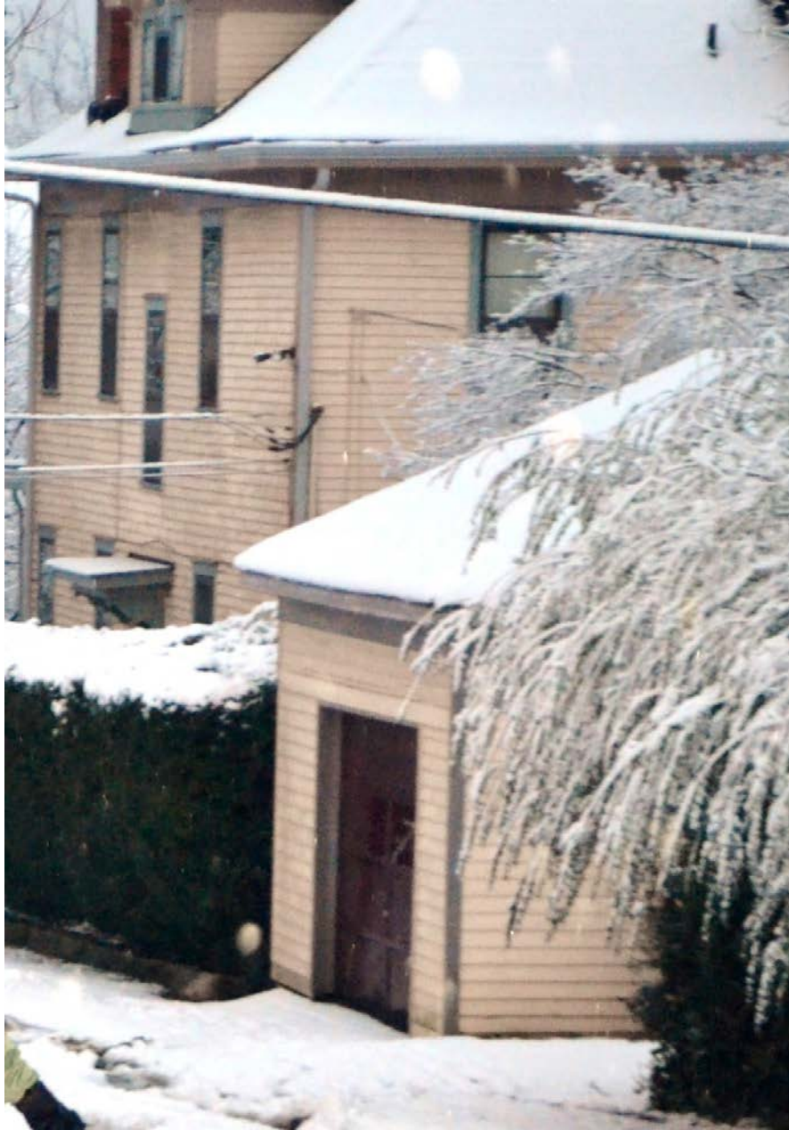
941 Eleanor Street garage facing Caswell Street
