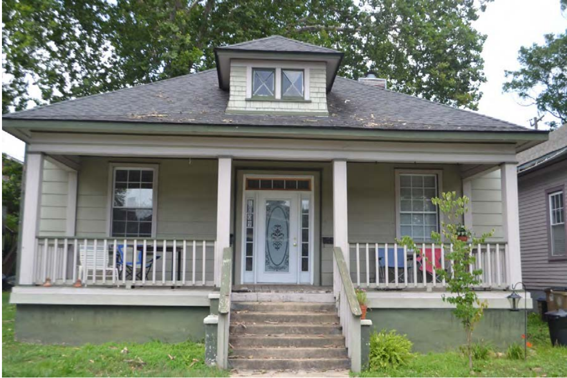
1015 Gratz St. – 1009 Gratz Street replacement windows
