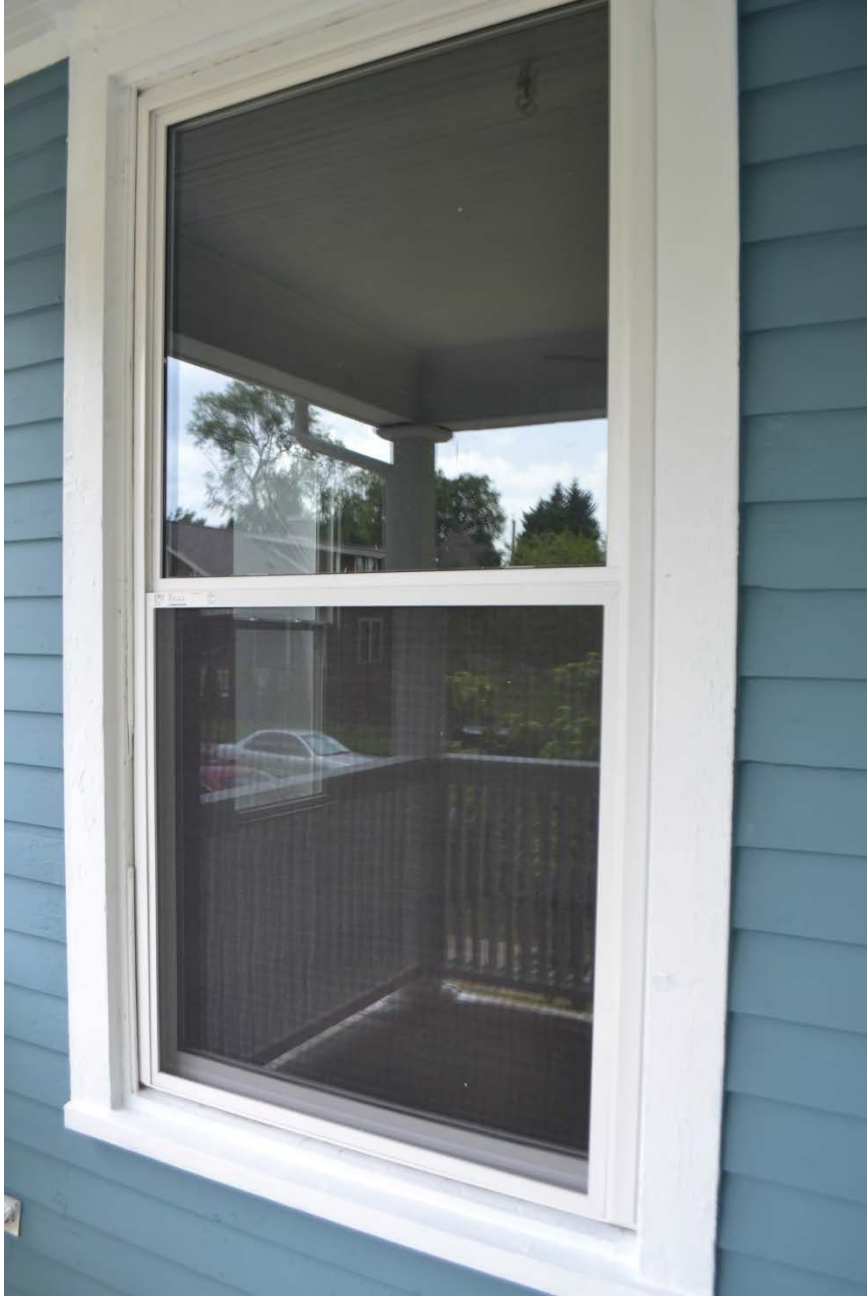
1015 Gratz St. – Vinyl replacement window on front with storm window
