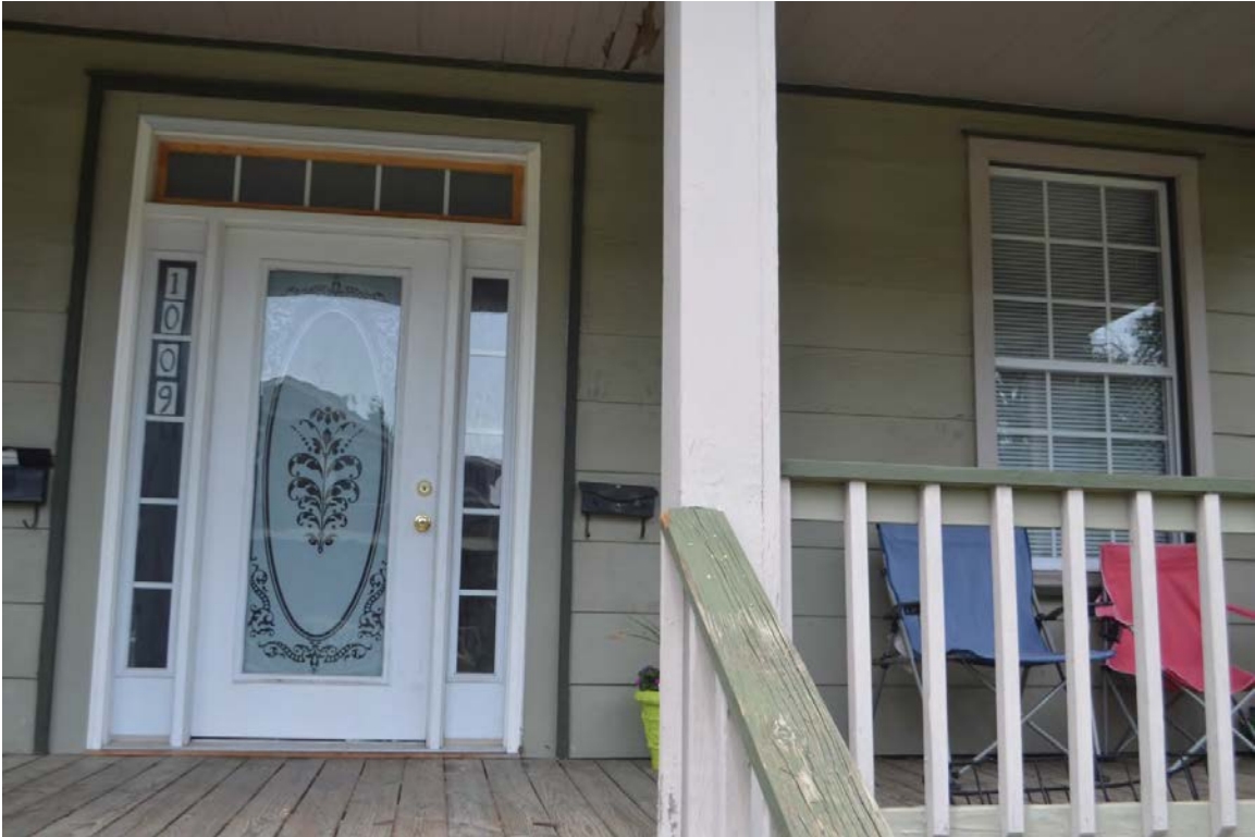
1915 Gratz St. – 1009 replacement front door
