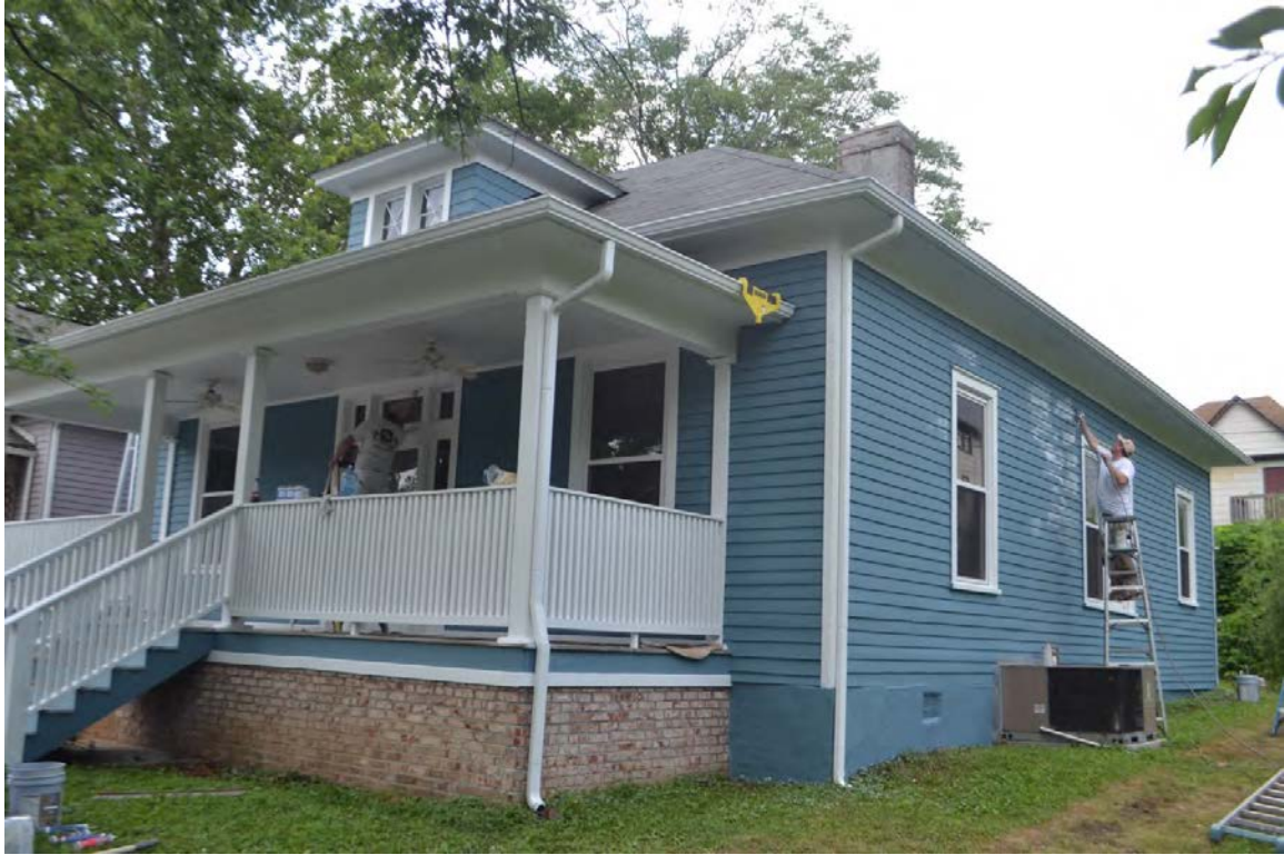
1015 Gratz St. – Front and north side
