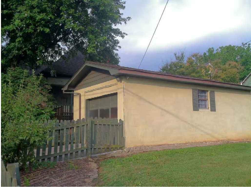
145 Leonard Place – Garage building
