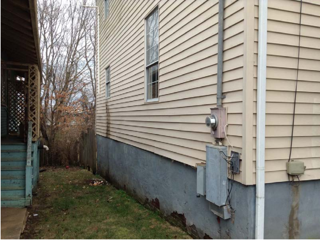
1206 Luttrell – North side
