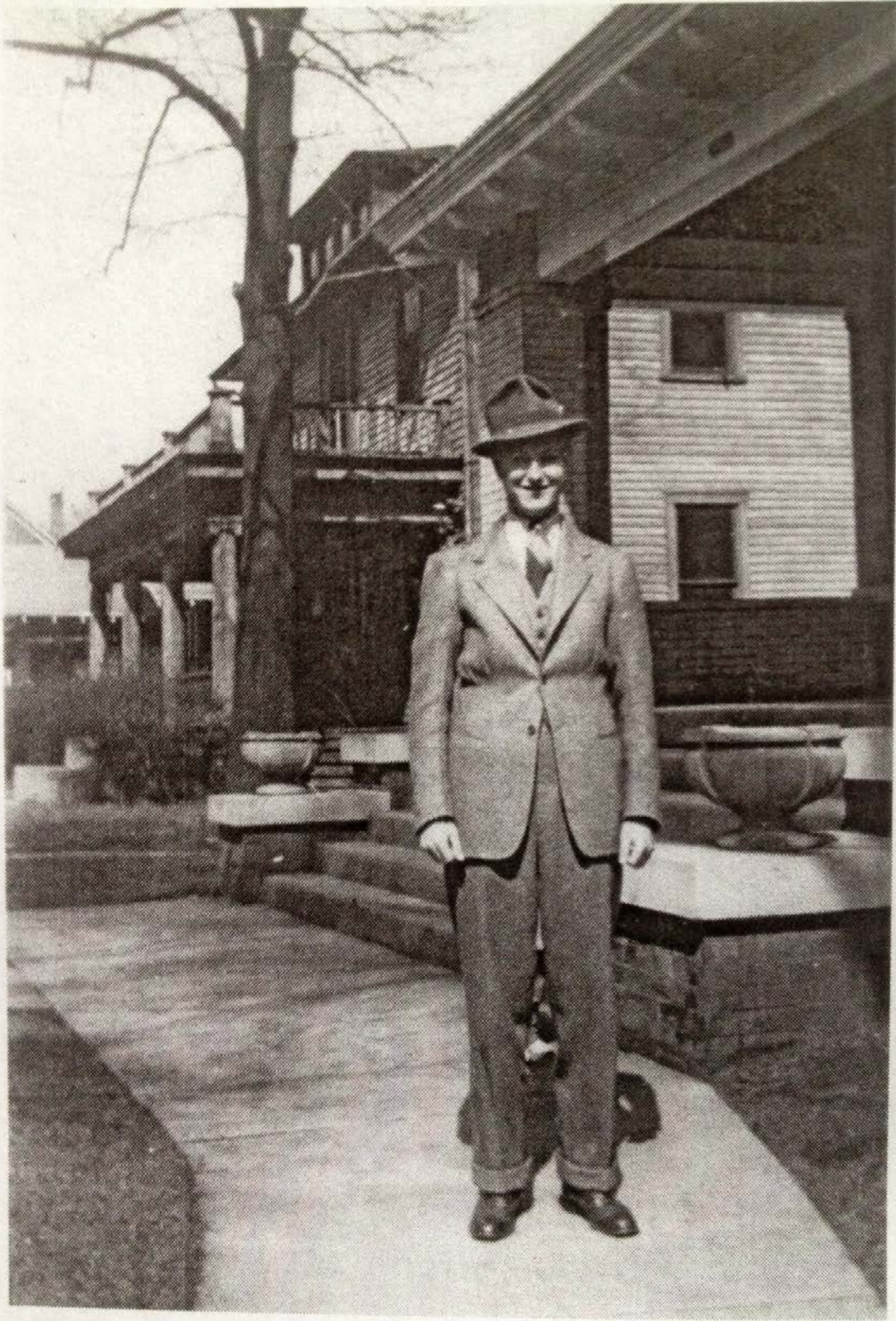
1206 Luttrell – Older photograph
