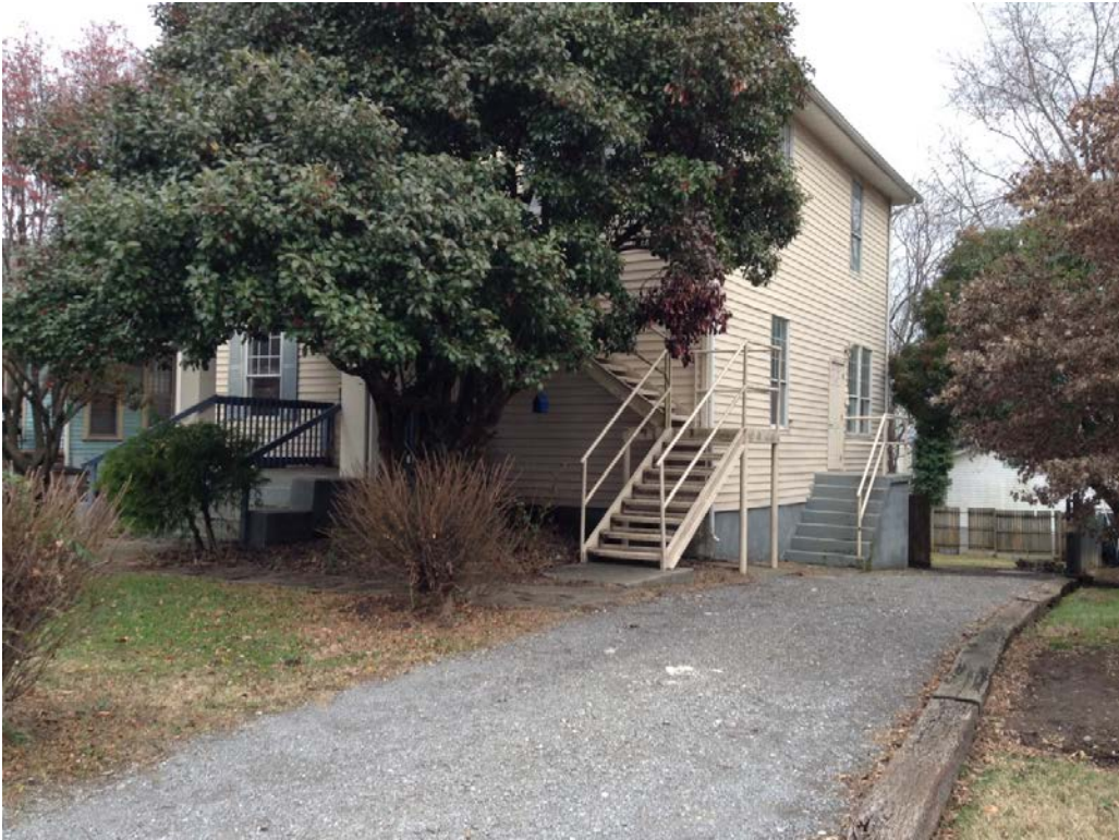
1206 Luttrell –View from southwest
