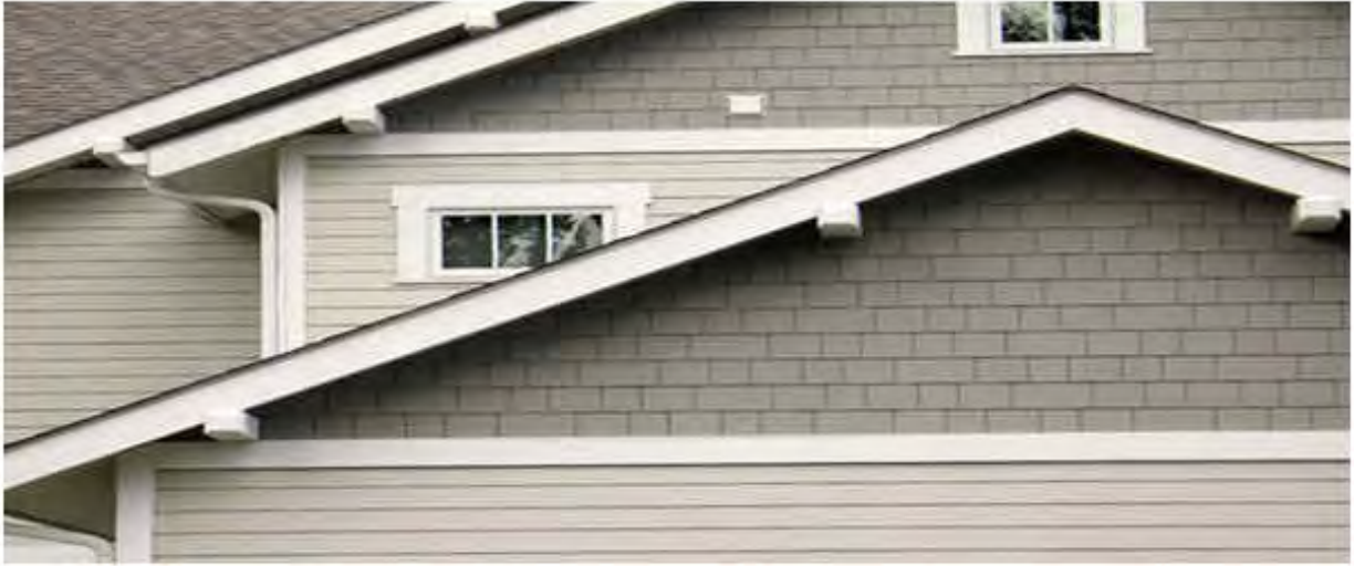
11029 Lake Ridge – Fiber cement board and shingle example
