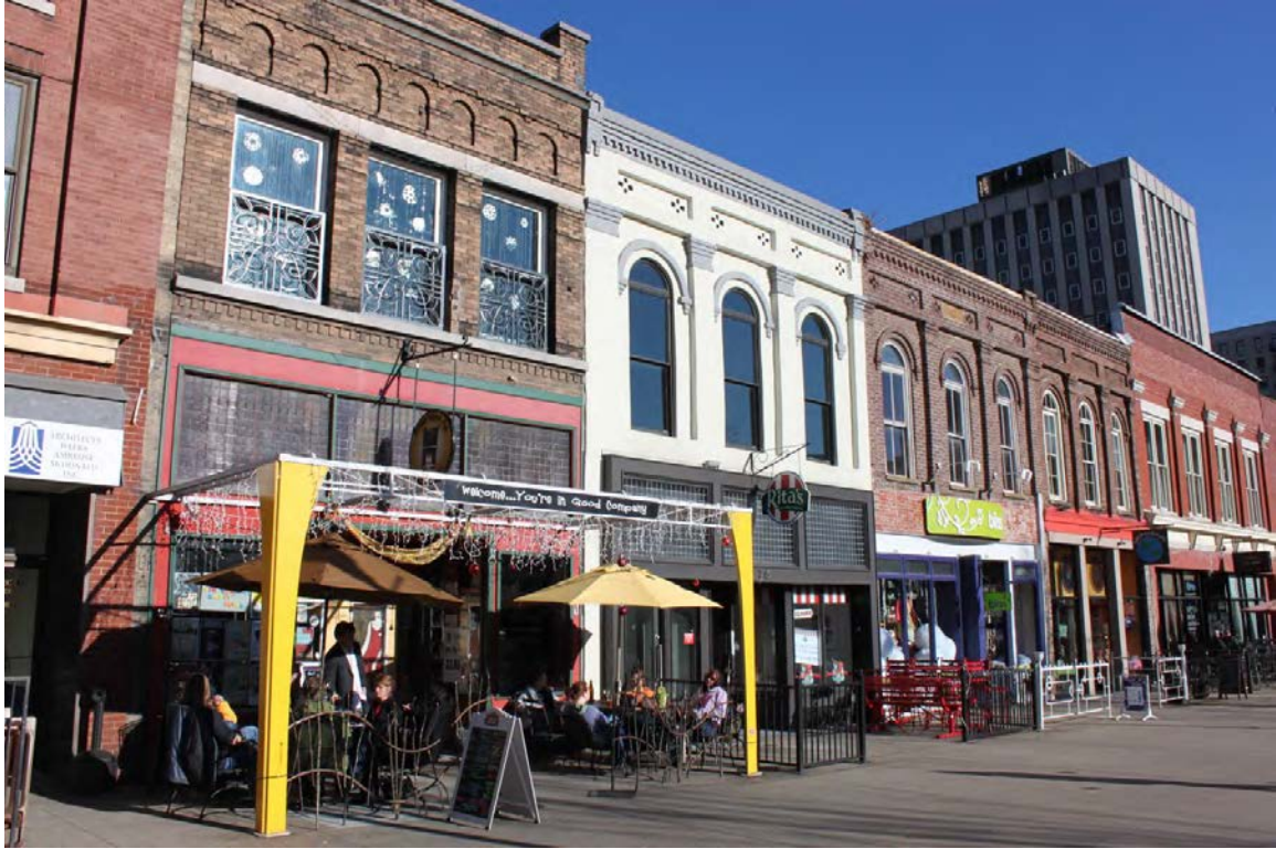
Market Square facades – East side
