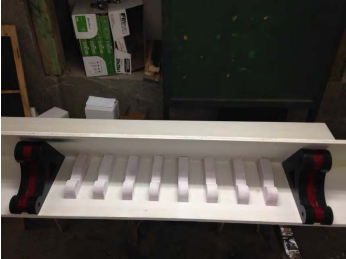
28 Market Square - Partially painted cornice mock-up
