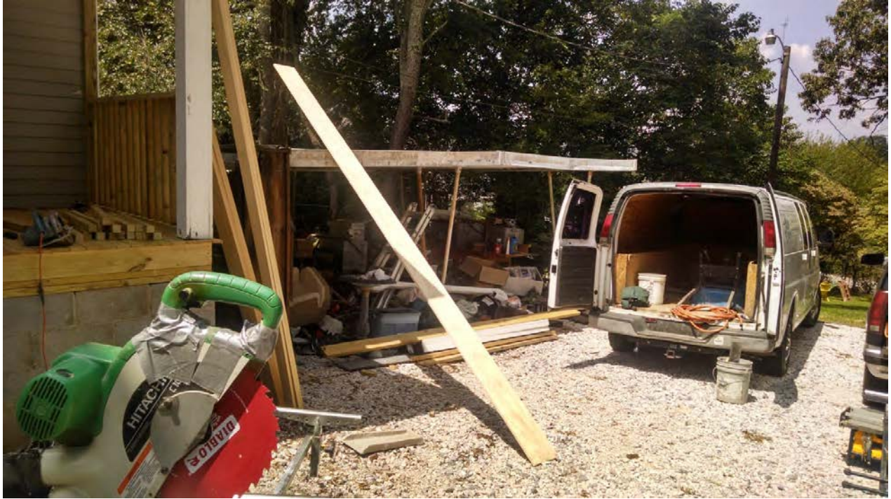
311 E Scott - Existing carport & porch corner
