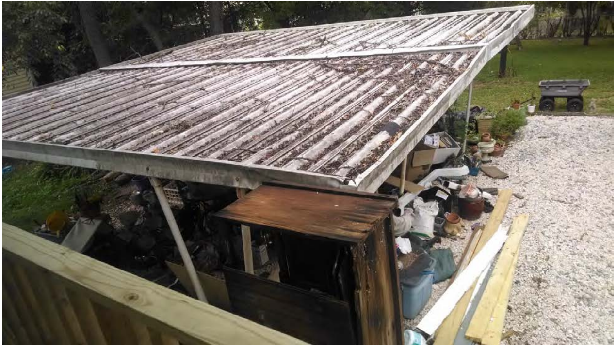
311 E. Scott - Existing carport from rear porch deck
