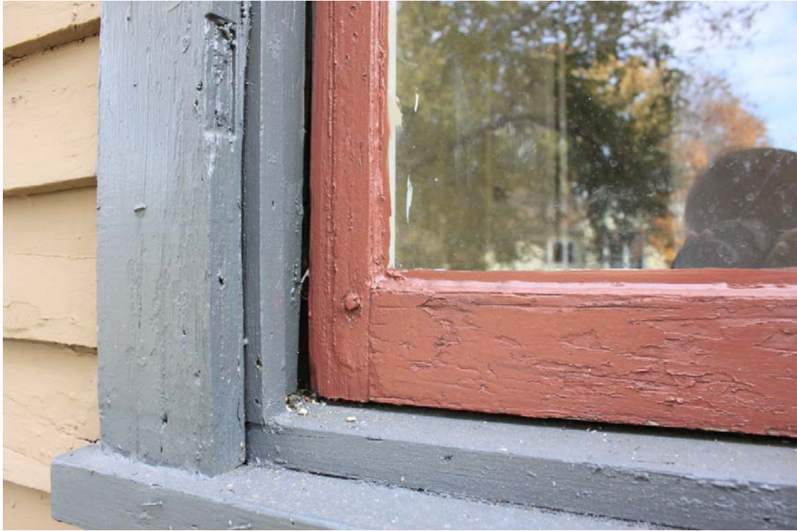
725 Deery – North side window close up
