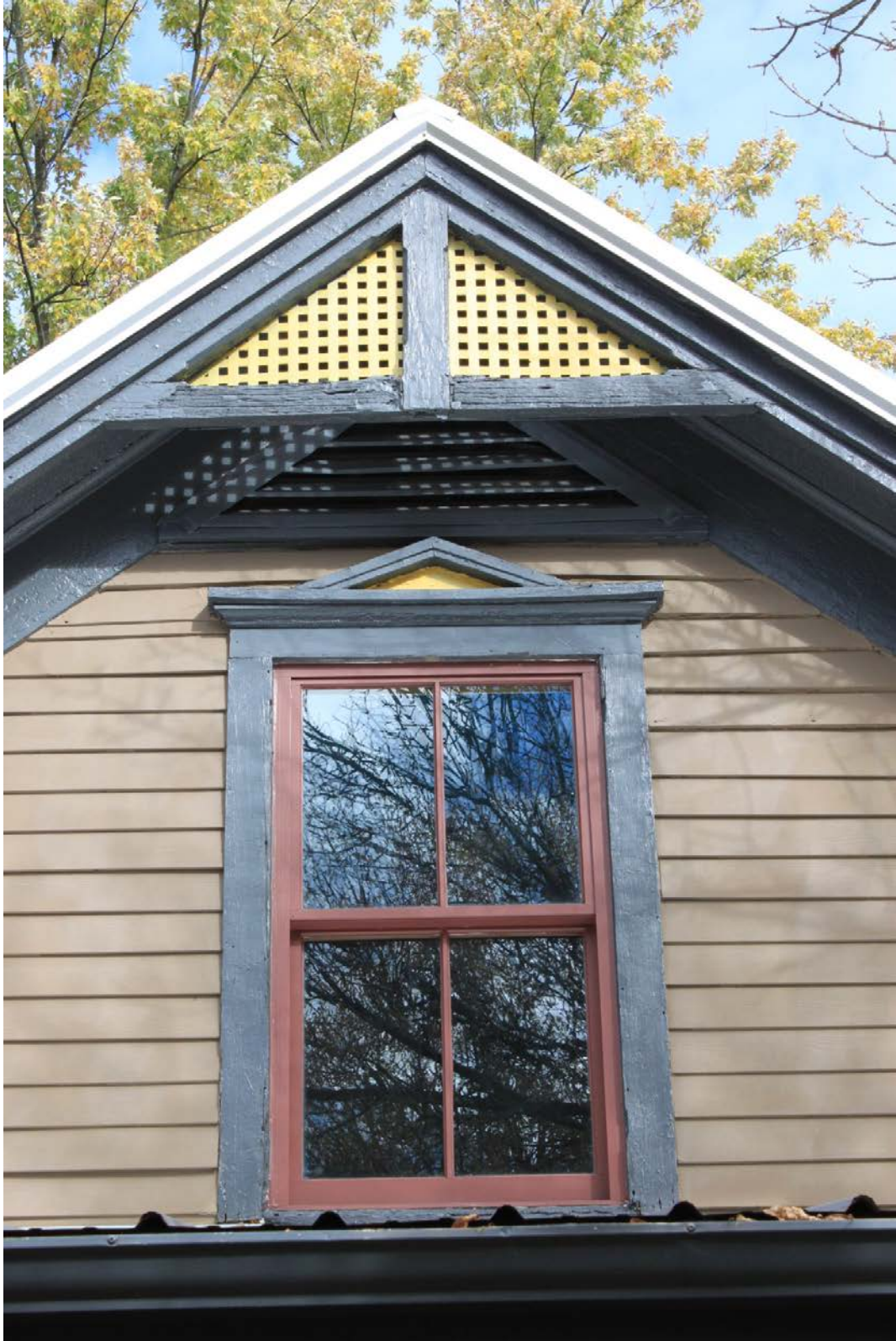
726 Deery – Upper front window replacement
