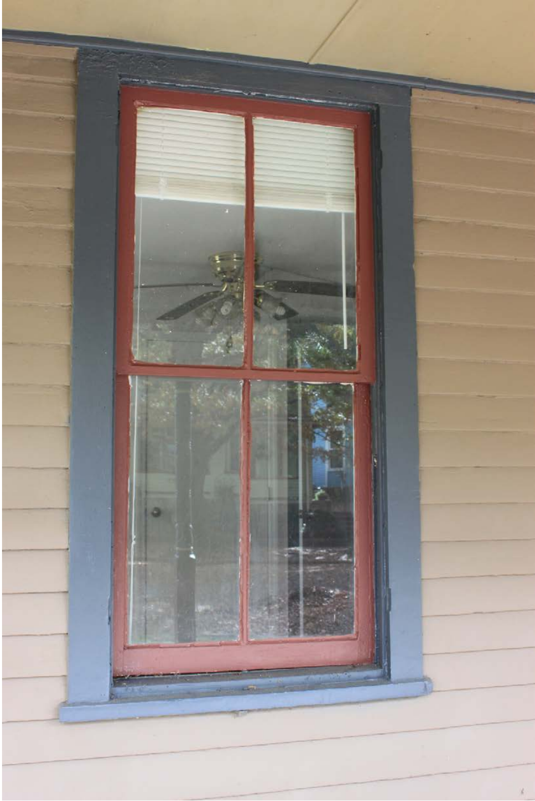
726 Deery – 1st level front window under porch roof
