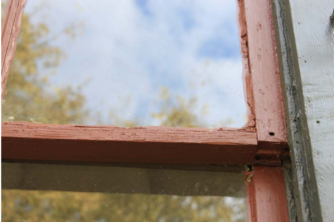
725 Deery – North side window close up
