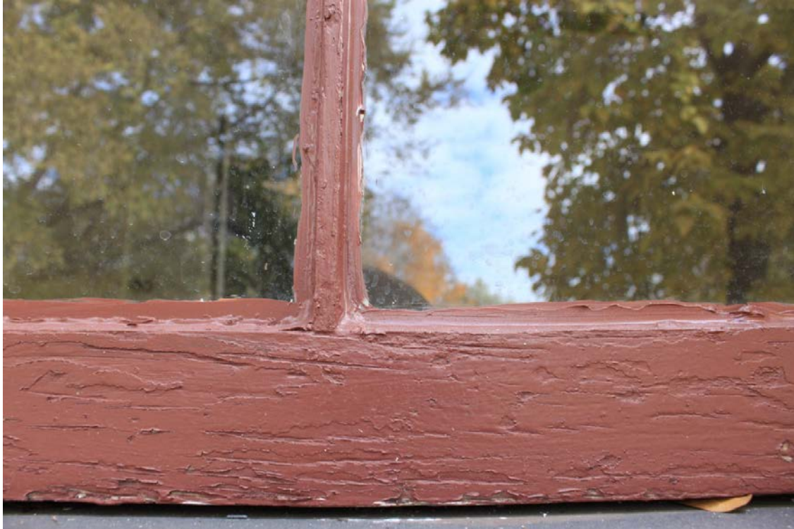
726 Deery – North side muntin close - up
