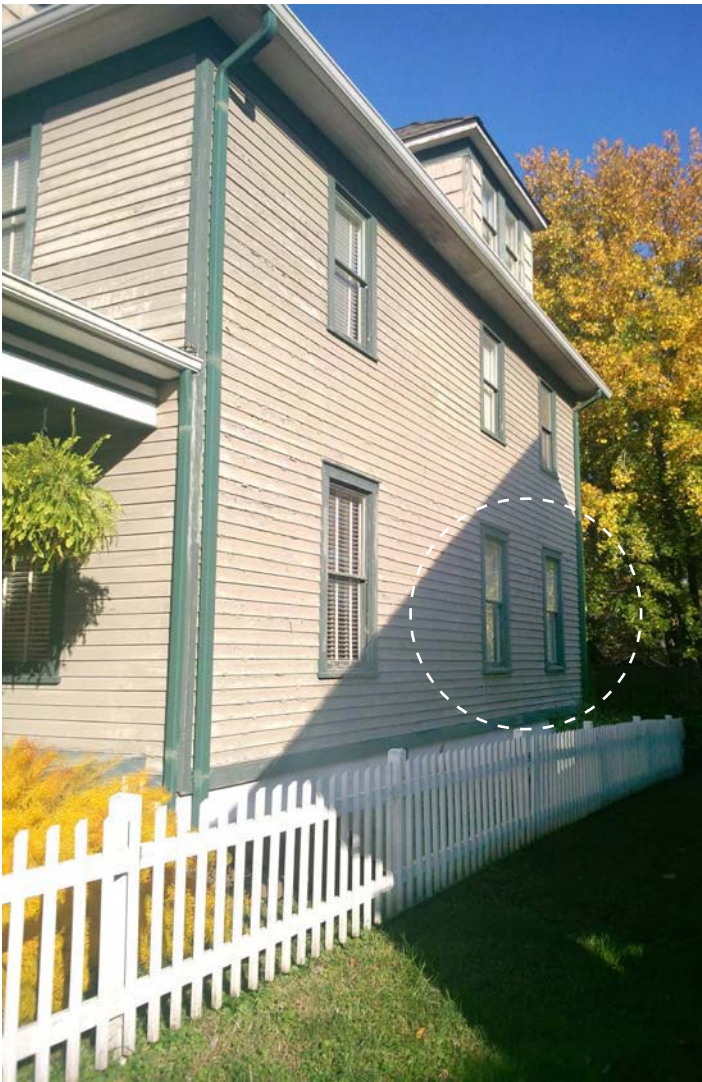
Existing kitchen windows
