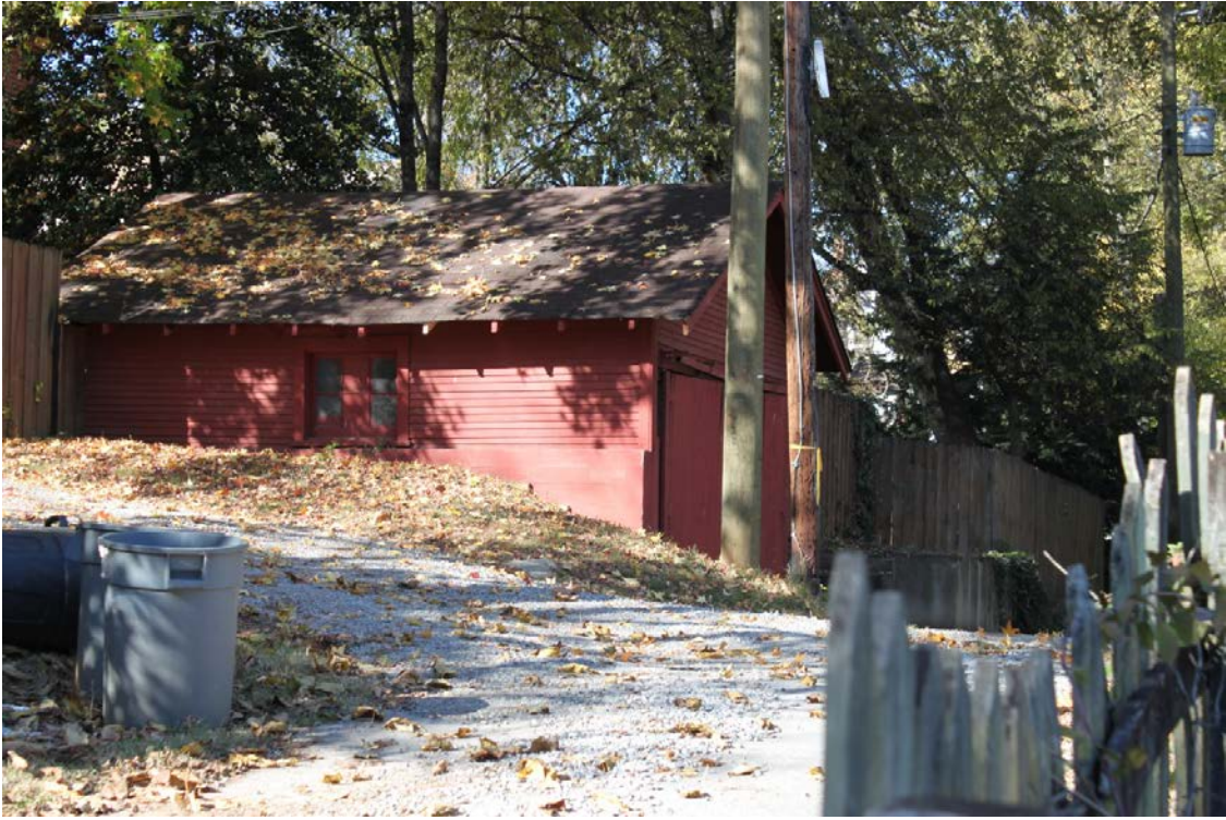
906 Luttrell – Existing garage from alley
