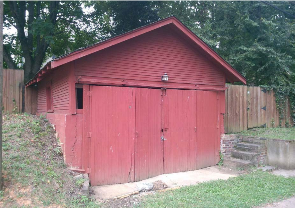
Existing garage (view from alley).
