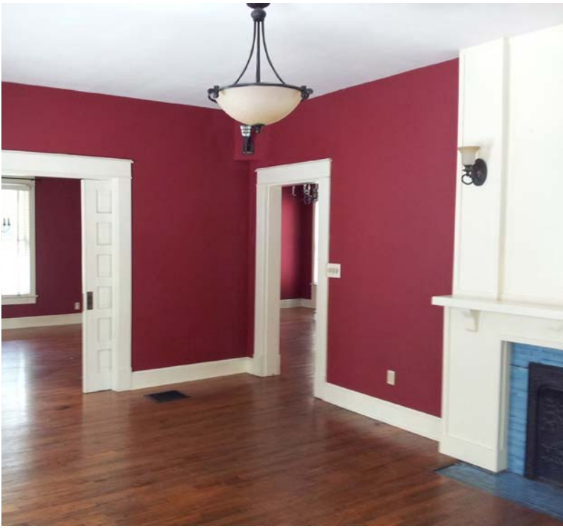
Existing fireplace on north wall of new kitchen
