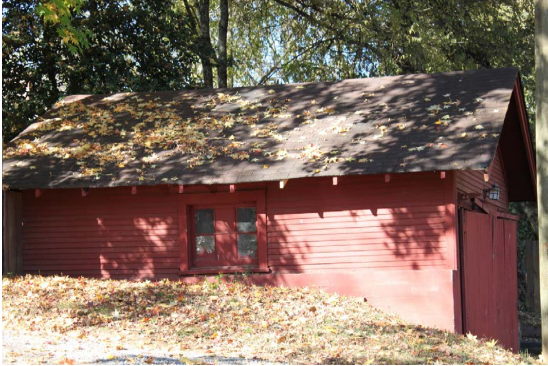
906 Luttrell – Existing garage
