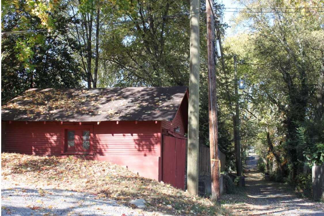
906 Luttrell – Existing garage looking north up alley from Gill Ave.
