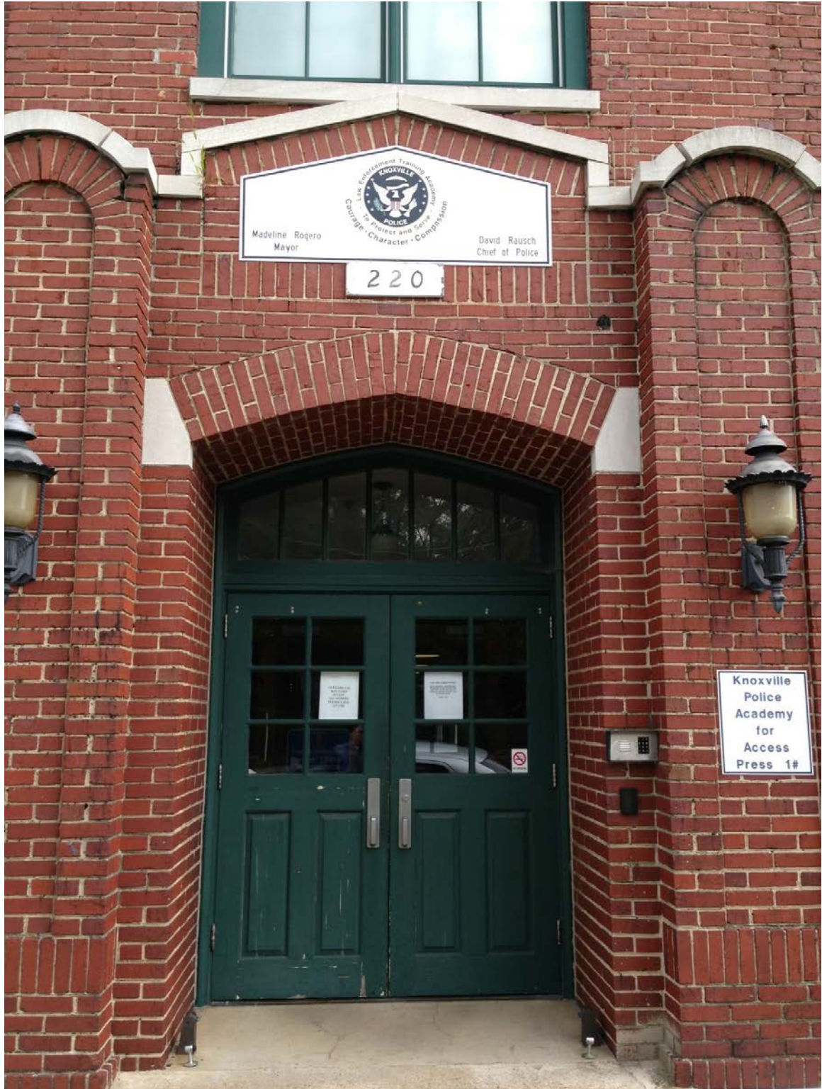
Moses Center- Carrick Street entry doors
