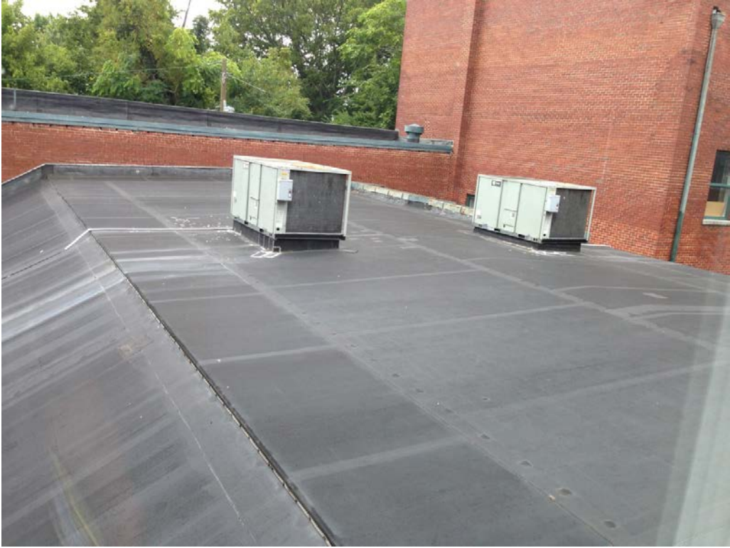
Moses Center- Gym Roof
