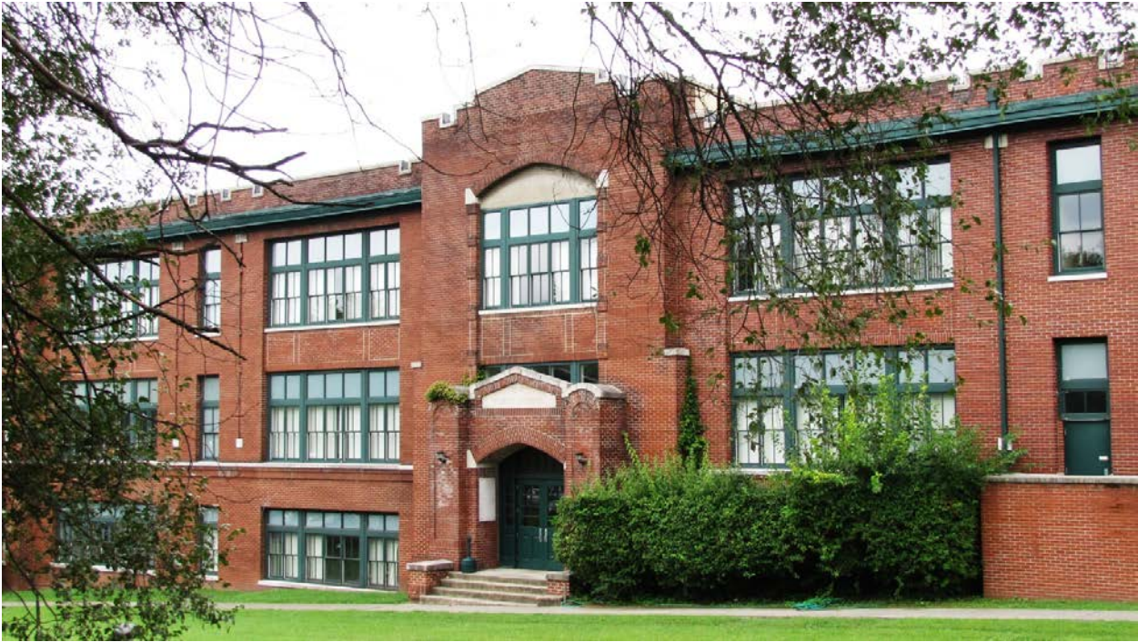
Moses School – Front entrance
