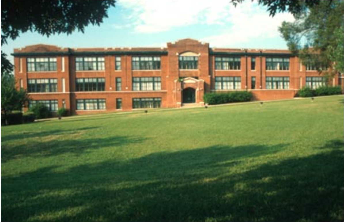
Moses School – Front façade
