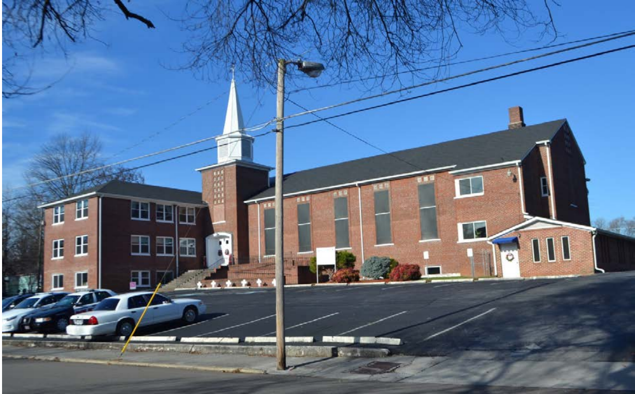
Church and surface parking lot to north
