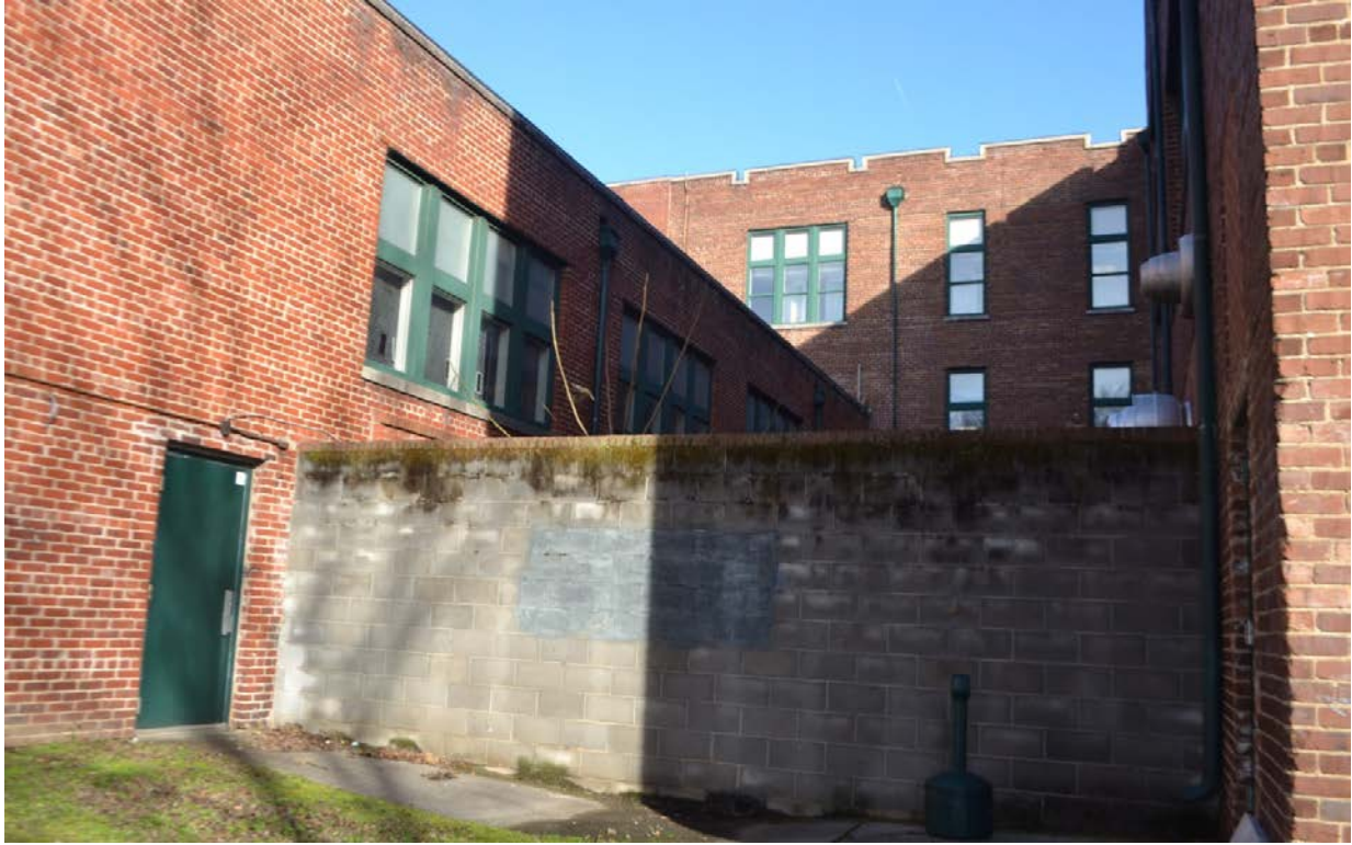
Moses School form rear (south side) looking toward location of gym
