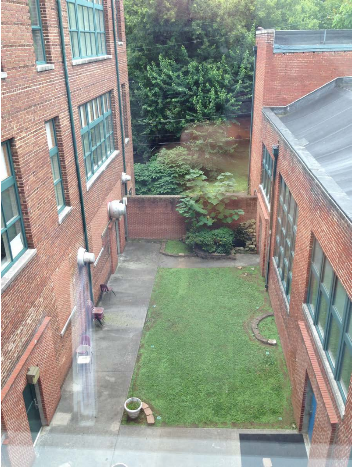
Moses Center- Courtyard and Gym Facades
