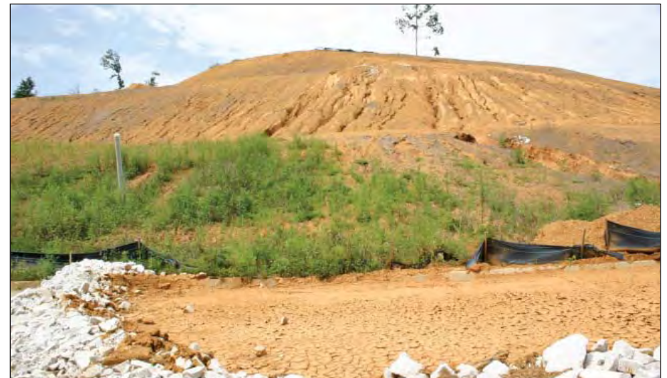
The above image was taken in September of 2008 during clearing and grading of phase III of the Wildwood Subdivision. Below: As of August 2009, the same area remained unstable. A portion of the hillside washed out closing a road in the neighborhood and causing water quality violations.
