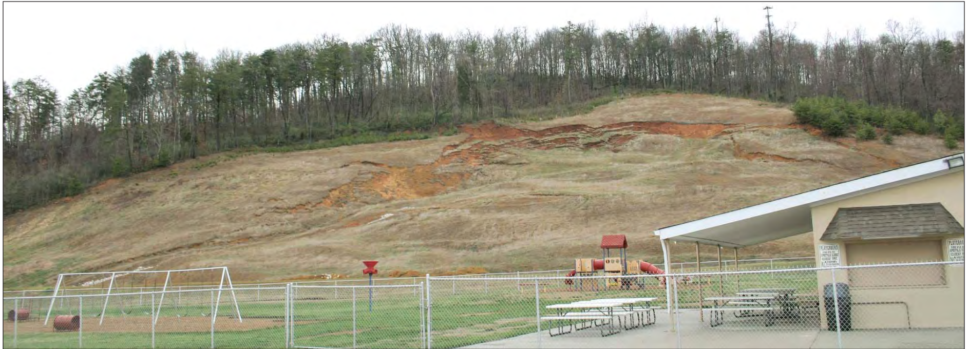
Soil slumping shown in the hillside area behind the playground demonstrates continued failure of the soil even after multiple attempts to stabilize the site.
