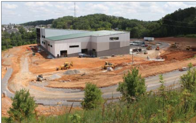
Construction of Local Motors Microfactory, August 2015
