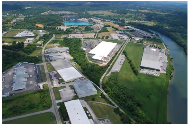
Forks of the River Industrial Park
