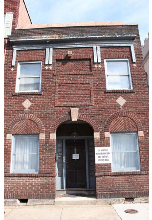
A series of demolition requests have spurred a review of the Downtown Design Review Guidelines.
