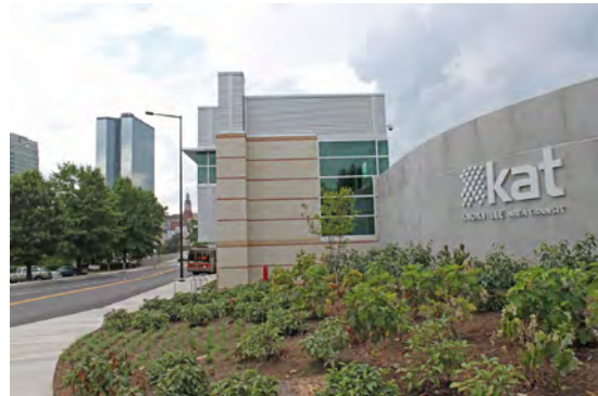
Knoxville Station Transit Center
